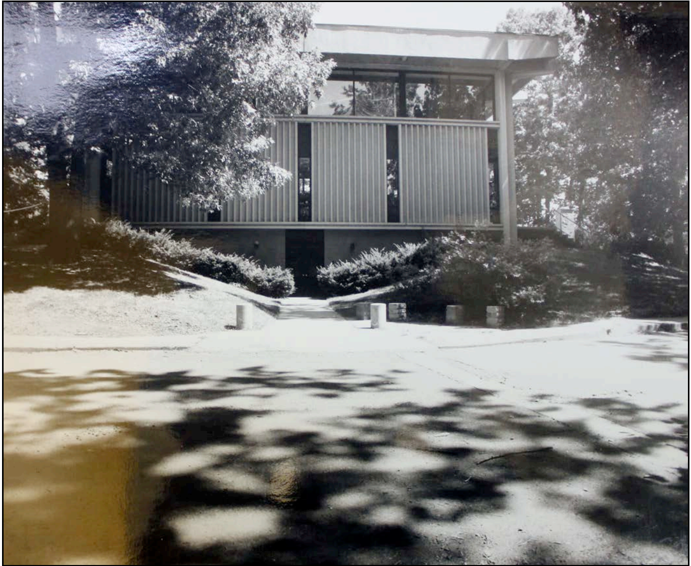
Image 32: Photograph south elevation looking north, pre-construction by Dustin Construction Co, Inc., dated July 22, 1993. From the Archives of the Unitarian Universalist Church of Arlington.
