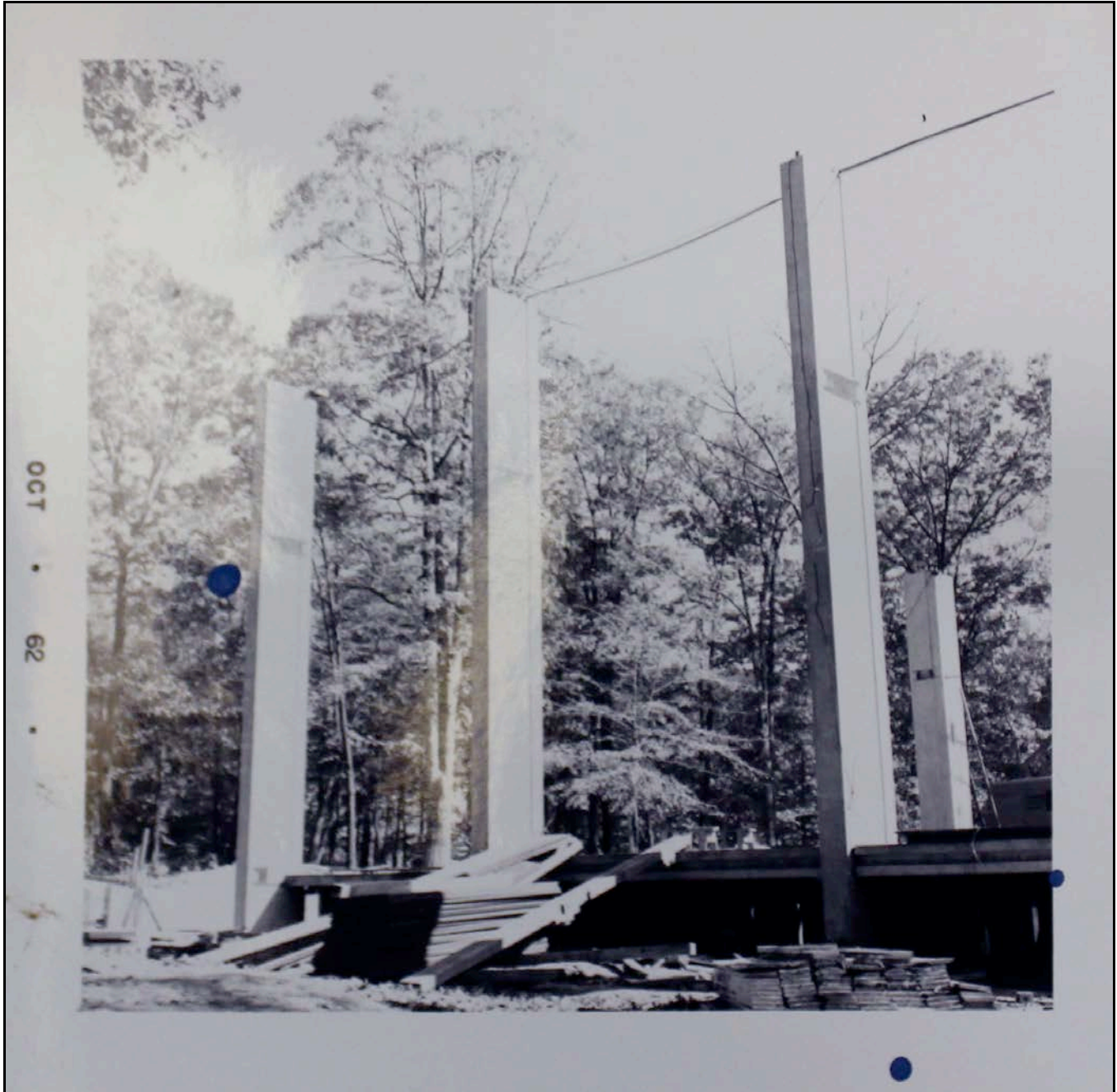
Image 22: Photo of Sanctuary Construction, dated October 1962. From the Archives of the Unitarian Universalist Church of Arlington.
