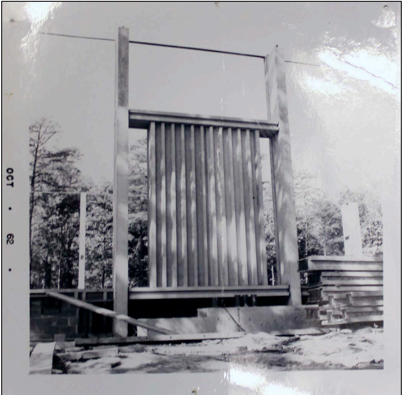
Image 23: Photo of Sanctuary Construction, detail concrete panel, dated October 1962. From the Archives of the Unitarian Universalist Church of Arlington.
