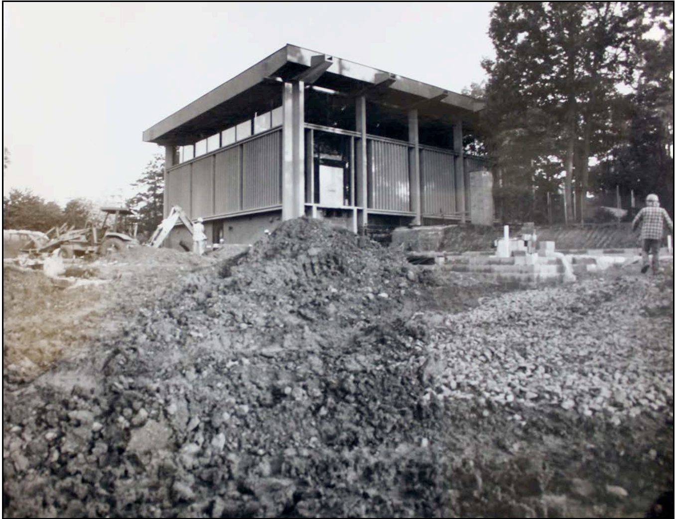
Image 33: Photograph looking northwest during construction by Dustin Construction Co, Inc., dated August 25, 1993. From the Archives of the Unitarian Universalist Church of Arlington.
