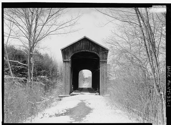
Shoreham Railroad Bridge (1897) Shoreham, Addison County, Vermont Rutland Railroad Company, Builder Howe truss
