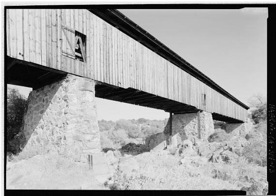
Knight's Ferry Bridge (1863) Knight's Ferry, Stanislaus County, California Schuylkill Construction Company, Builder Howe truss
