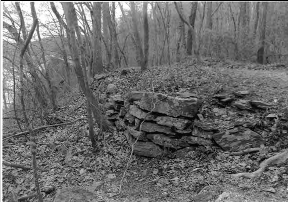
Photo 14 of 40 Canal Works (NR#46), East of Locks 2 & 3, view S
