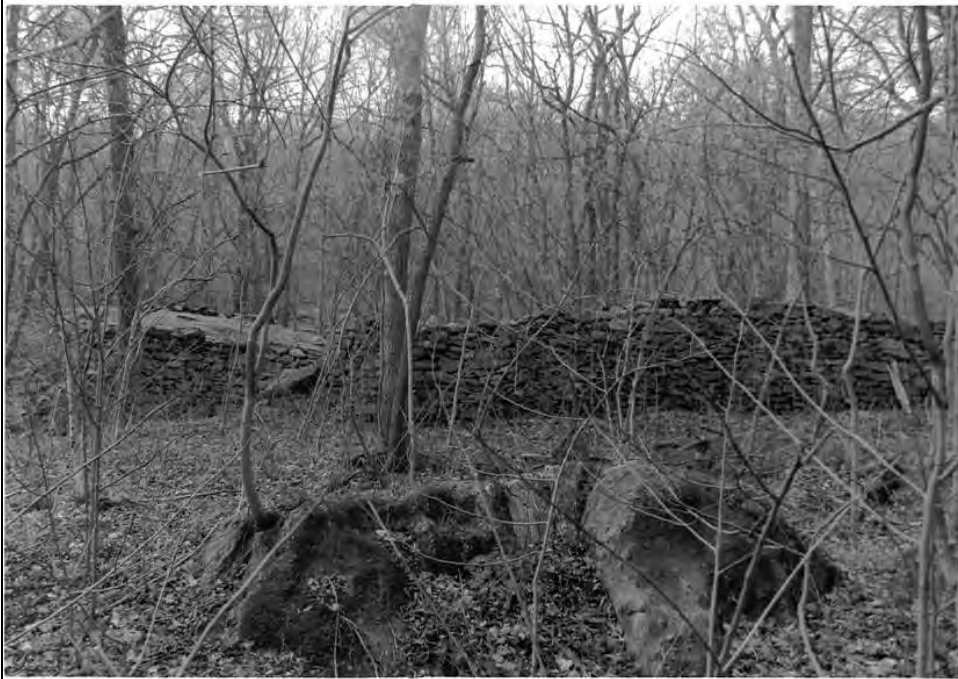
Photo 10 of 40 Collecting Basin Wall, SE corner (NR#37), view SW
