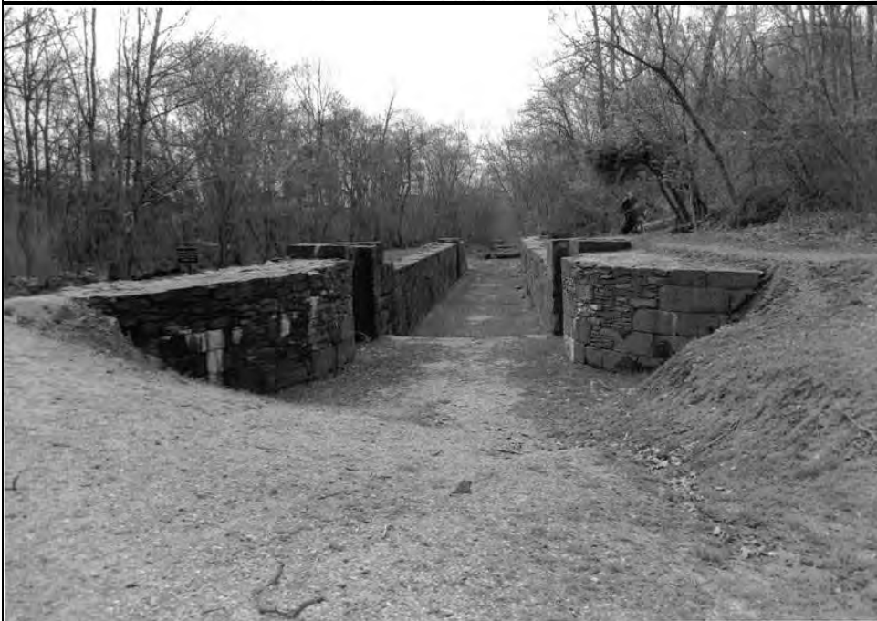
Photo 12 of 40 Lock 1, view S (NR#41)
