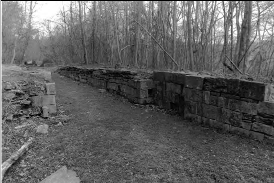
Photo 13 of 40 Lock 2, view NE (NR#42)
