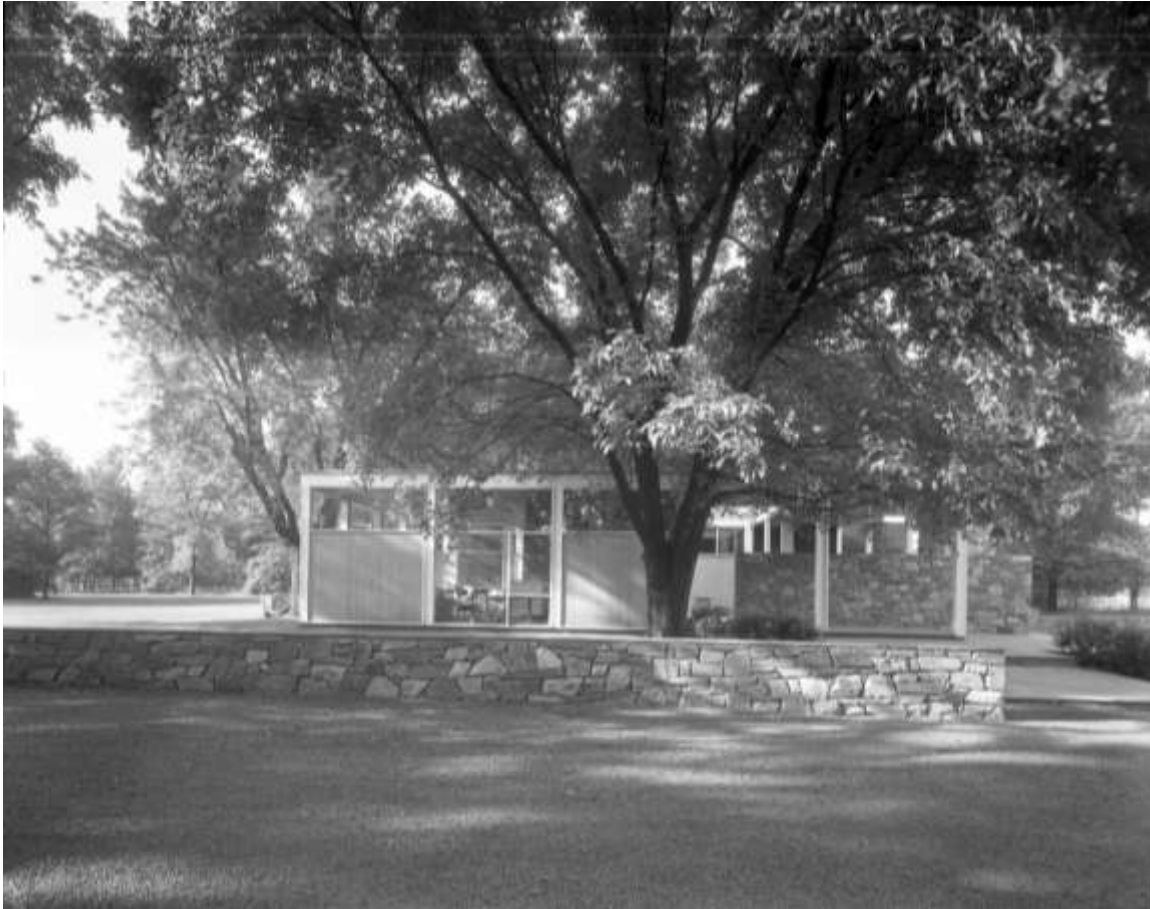
10 of 11: View of the Goodman addition from the entry courtyard, ca. 1954. The path to the house is at the right. The visitor is confronted first with a stone wall, obscuring the open courtyard beyond, and the entry door is hidden to the left. From the Robert C. Lautman Photography Collection, box 34, courtesy of the National Building Museum, Washington, D.C.
