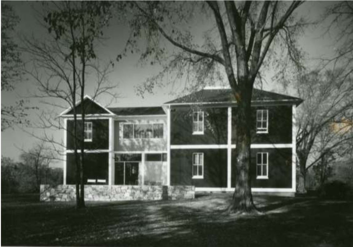
6 of 11: Photograph of southern façade of farmhouse post Goodman renovation, ca. 1954, showing the original farmhouse (right) and the additions of the hyphen (center) and gabled structure (left). From the Robert C. Lautman Photography Collection, box 33, courtesy of the National Building Museum, Washington, D.C.
