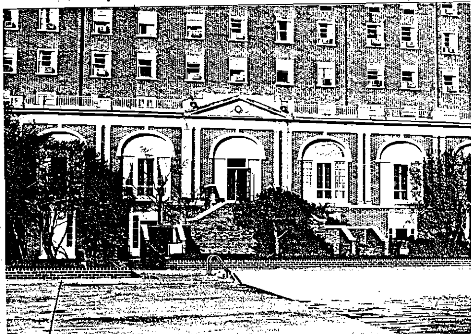
Detail of south elevation
