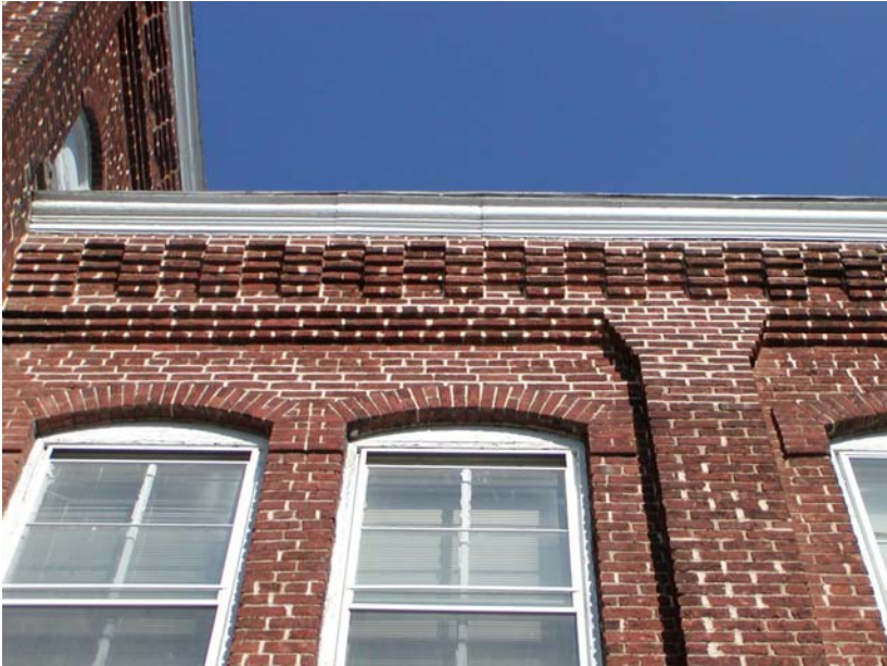
Brick detailing at cornice line
