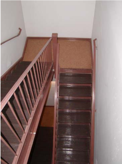
Staircase was rebuilt in existing location to meet code
