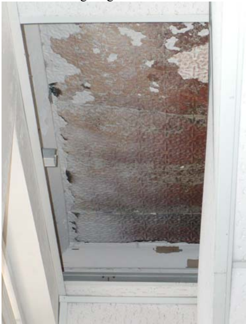
Original ceiling in place above dropped ceiling in classroom/apartment
