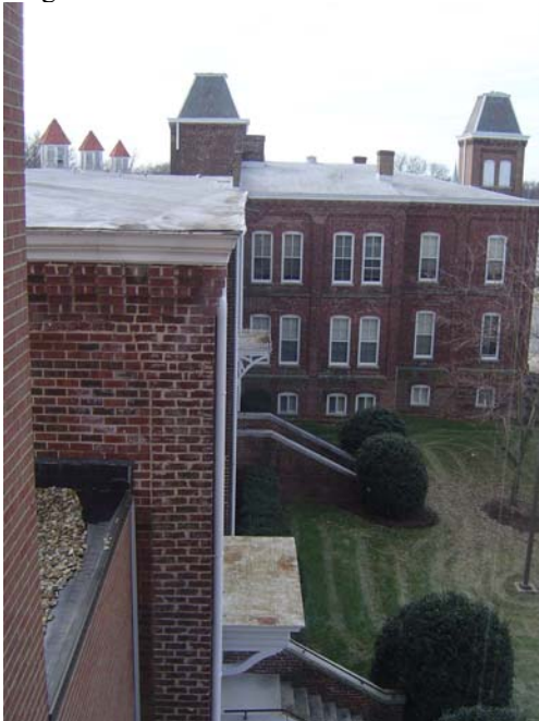
Roof of Fairmount School
