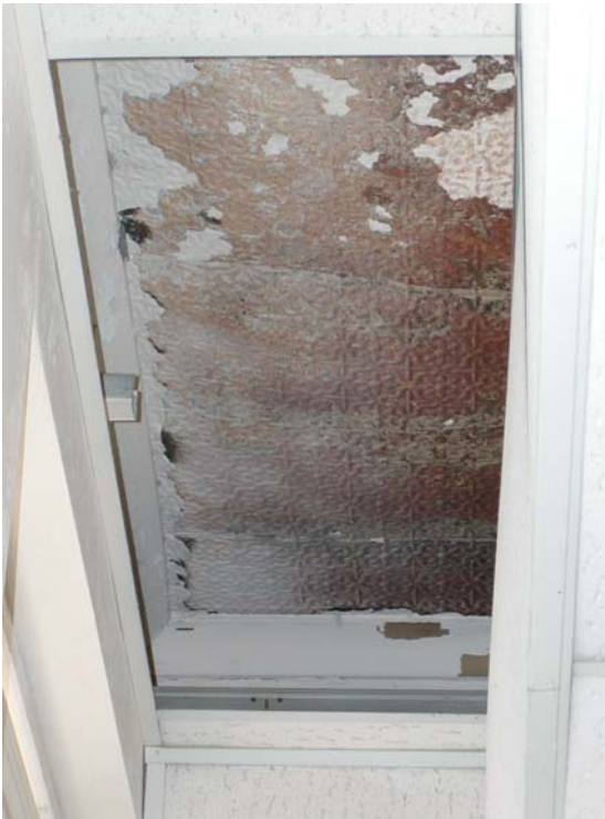
Tin ceiling in classroom/apartment
