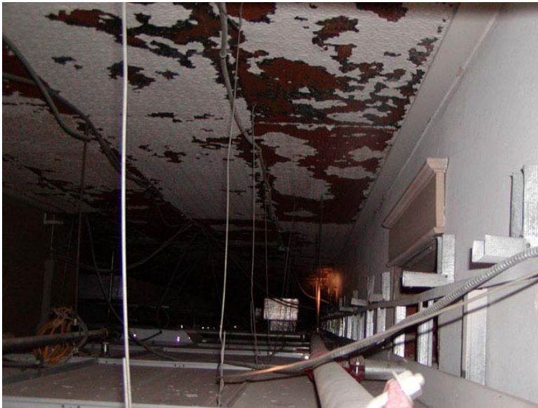
Corridor looking north above dropped ceiling tiles
