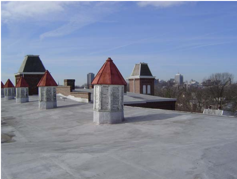
Roof of Fairmount School
