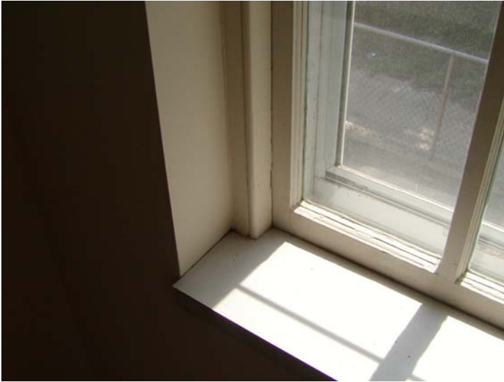
Original sashes and jambs, but trim encased beneath present drywall
