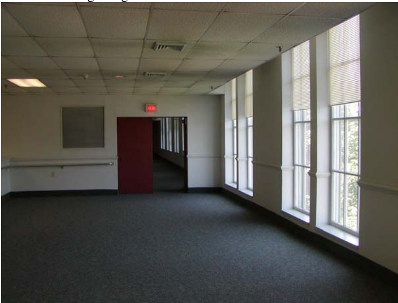
There was no wainscoting along corridors and in the classrooms, but a high chair rail was used to define “wainscot” area defined by paint instead of paneling
