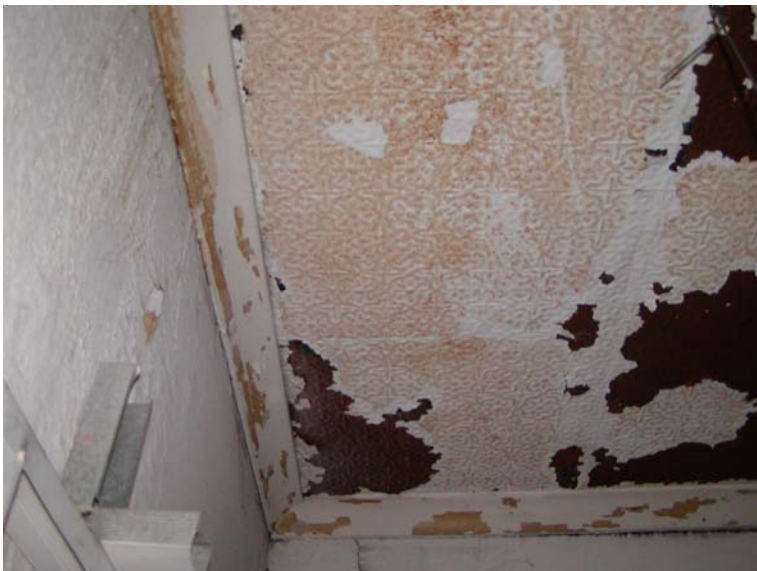
Corridor ceiling above dropped ceiling tiles
