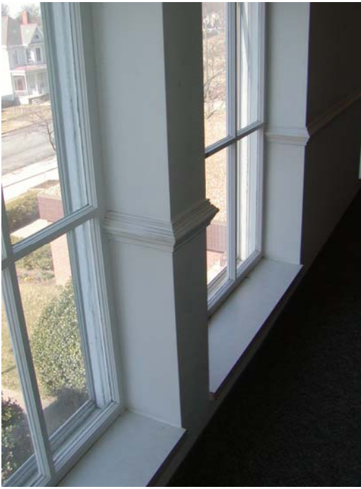
Reproduction wood windows “in kind” (had been removed in the 1950s)
