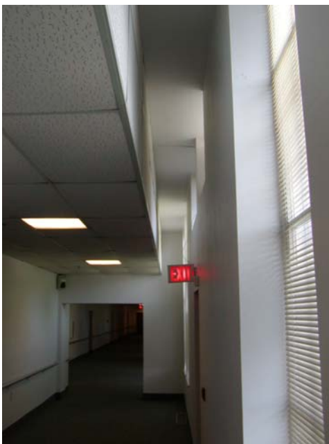
Original ceiling height revealed in corridor
