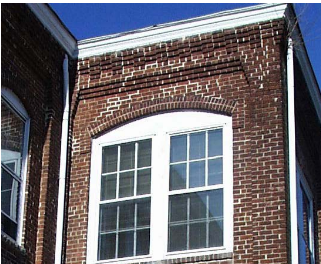
1909 addition brick detailing at cornice line
