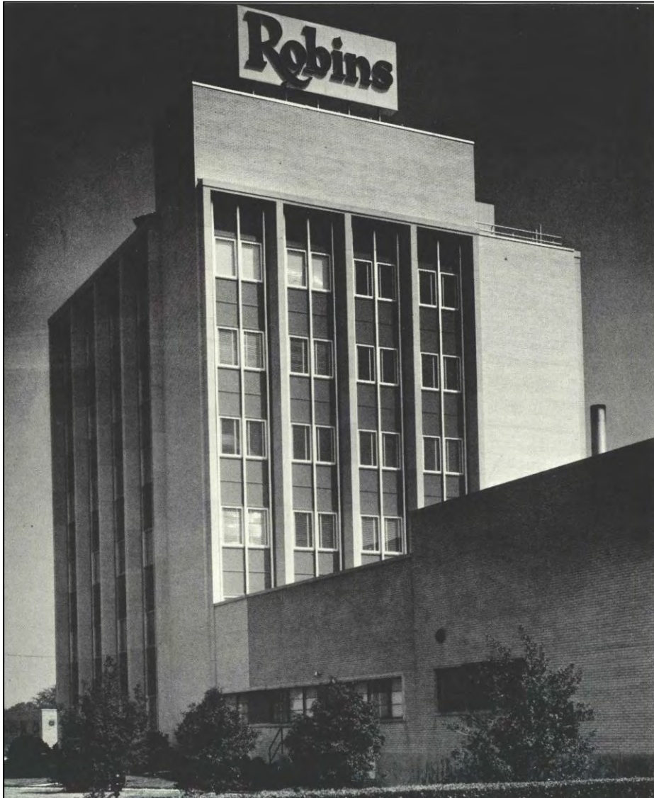
The Robins illuminated sign in 4 foot letters can be clearly seen from the Richmond-Petersburg turnpike.
