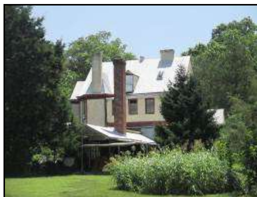
Remnants of Nickel's greenhouse at the back of 3001 Condie Street
