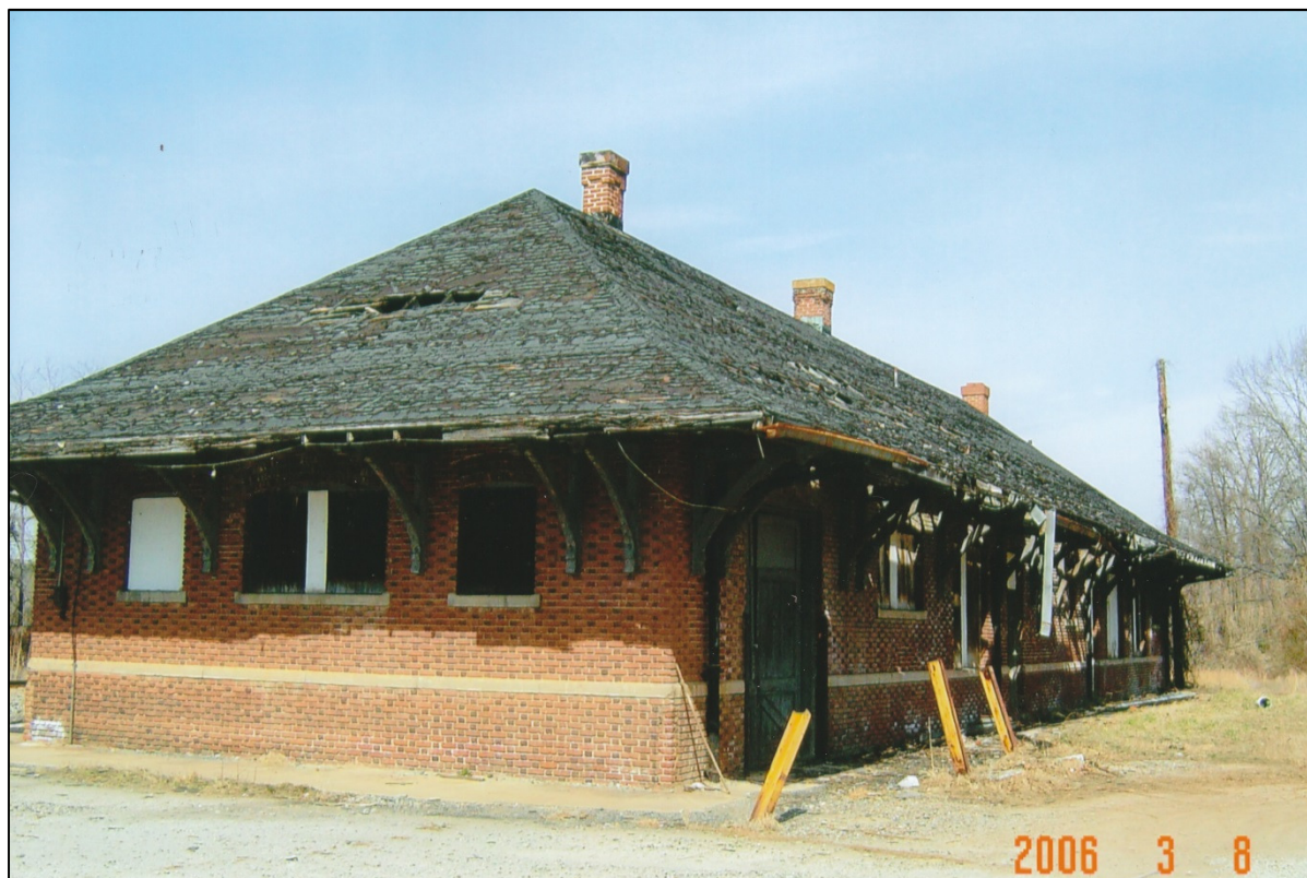
Fig. 3 Chatham Depot in 2006, shortly before its restoration began (Pittsylvania Historical Society)
