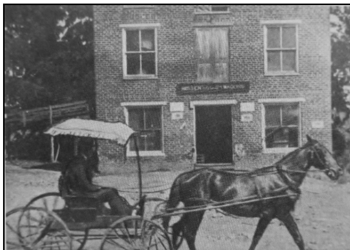
Figure 4. The brick warehouse built by Thomas Claiborne Creasy. The building, located at 101 South Main Street, is the oldest extant building in the Gretna Commercial Historic District (227-5002). Source: Tyler, The Junction .
