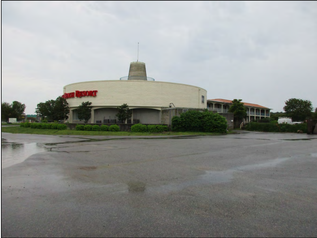
Figure 12. DHR # 065-5046. Sunset Beach Resort at 32246 Lankford Highway.
