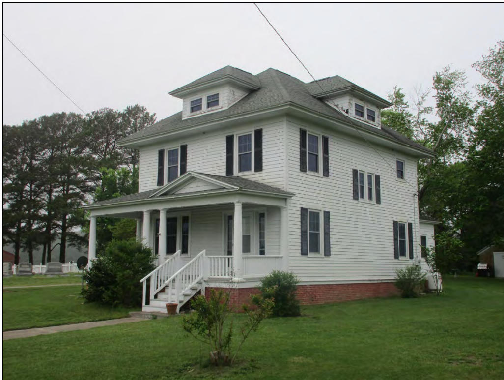
Figure 26. DHR # 217-5026. American Foursquare residence, 4140 Seaside Road.
