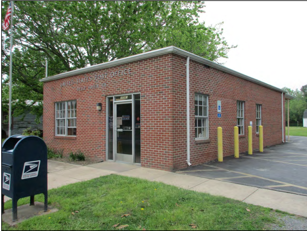
Figure 37 (DHR # 167-5001-0005). Belle Haven Post Office, 35561 Belle Haven Road.
