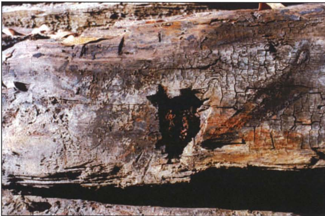
Figure 36. Triangular notch to start a spoon bit.
