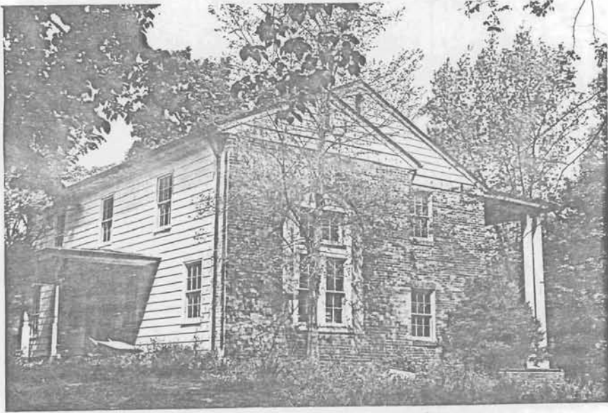
The Weaving House at "ALDIE" Manor. Rear Catslide Roof now modified to a full two story. Now a private dwelling. 53-115 (2617)
