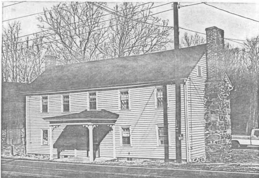
Two story frame dwelling, either of Log or Brick Nogging construction. Some beeded weatherboards remaining. Original solid M&T and Pegged window frames. Good period sash. Exterior rubble stone chimney capped in brick. There was apparently a wing on the west end at one time. Last quarter of the 18th Century, or early 1800's. 53-525 (3496)
