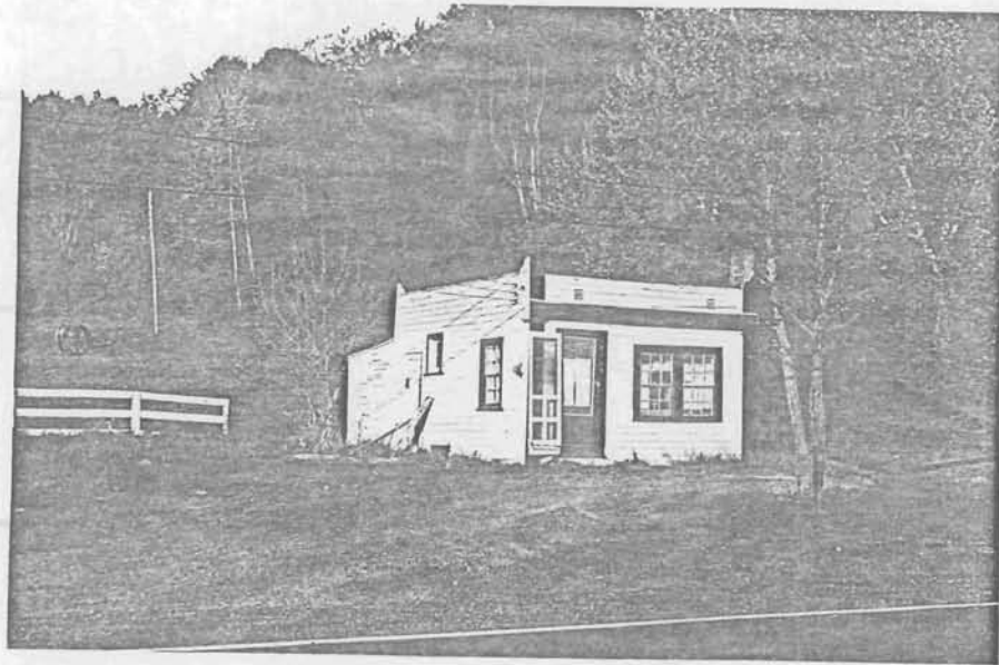
Circa 1940's commercial structure. Of no Architectural importance. See Reccomendations. 53-539 (3504)
