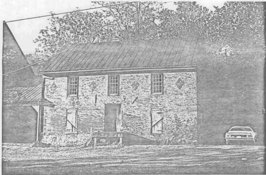
West end Wing, which contained the Store House. 53-113 (3503)
