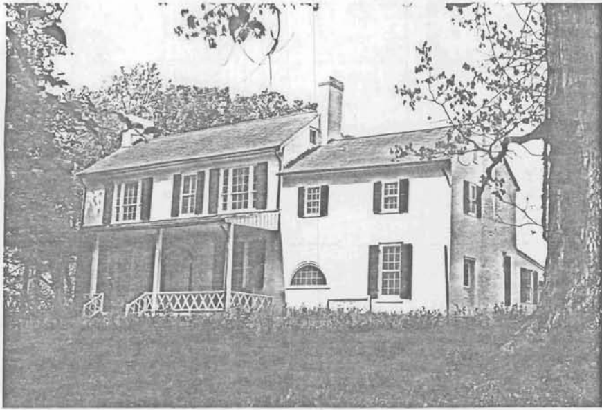
"ALDIE" built for Charles Fenton Mercer, circa 1810. Exterior windows changed and some interior woodwork by the diZeregas in the mid to late 1800's. Other more drastic changes were made to the interior by Commander Bullis, during his ownership. 53-115 (2617)
