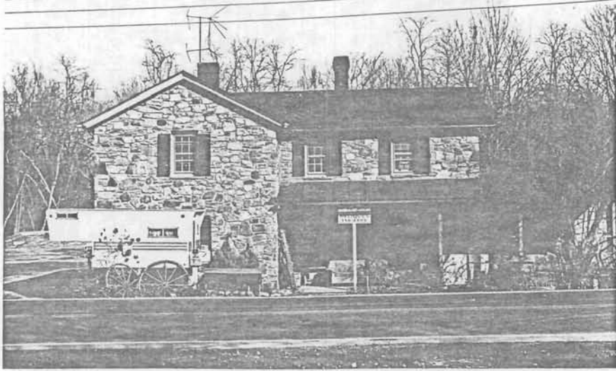
Mid 1800's two story frame dwelling with later exterior veneer, done in the mid 1900's. 53-524 (3496)
