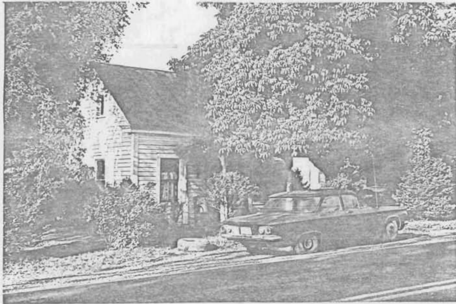
Pleasing One and one half story Frame, turn of the Century, Dwelling. Small scaled Entrance Stoop with turned posts. 53-548 (3503)
