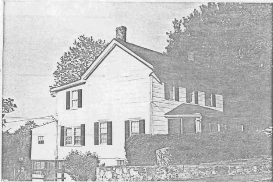
Turn of the Century Two Story Frame Dwelling. Original sash and shutters. Pleasant entrance Stoop. Good state of preservation although shingleing distracts somewhat from the quality. 53-555 (3507)
