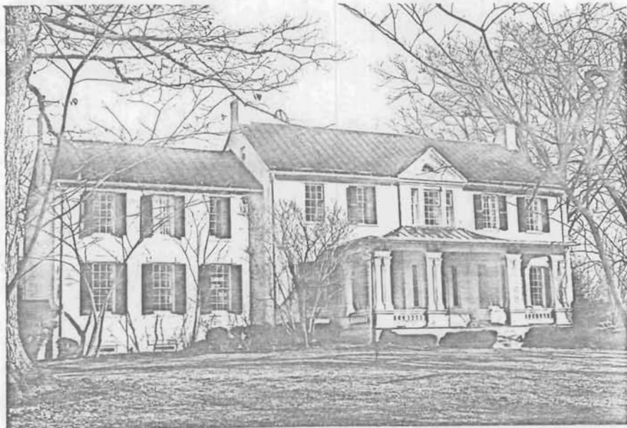
BERKELEY HOUSE. Early 1800's two story Brick dwelling in excellent state of preservation. Pleasantly scaled Pavilion and one story entrance porch with elaborate door unit. 53-532 (3496)
