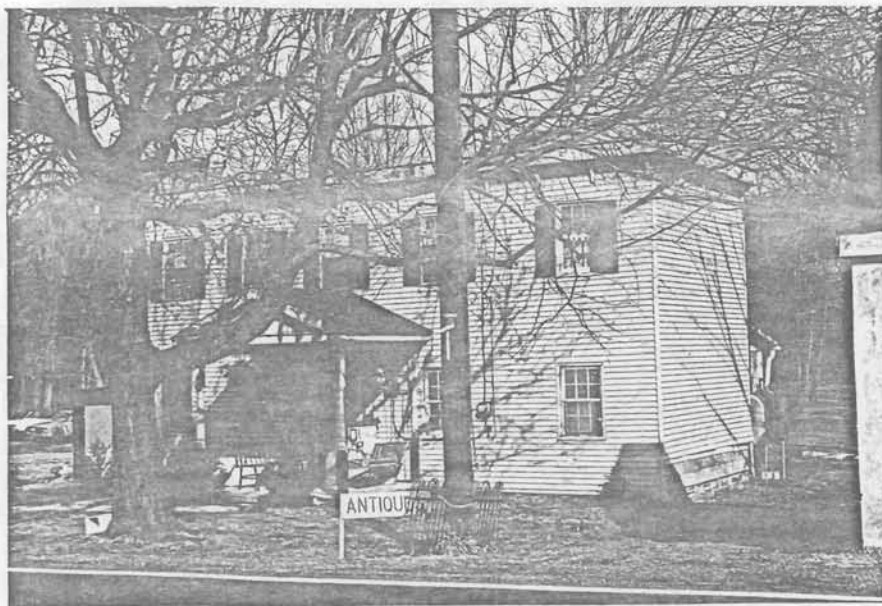
Mid 1800's two story frame Greek Revival style dwelling. May be earlier and modified to this style in the mid 1800's. Good eve Brackets, pleasant entrance porch with turned posts, original sash and shutters. 53-523 (3496)
