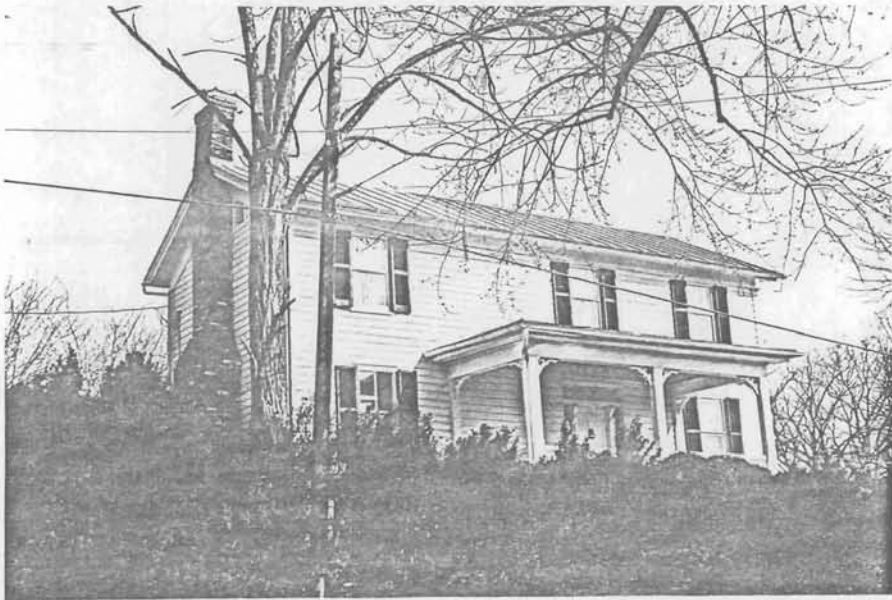
Turn of the Century Two story Frame Dwelling. Original sash and shutters. Good one story entrance porch with sawn brackets. 53-533 (3497)
