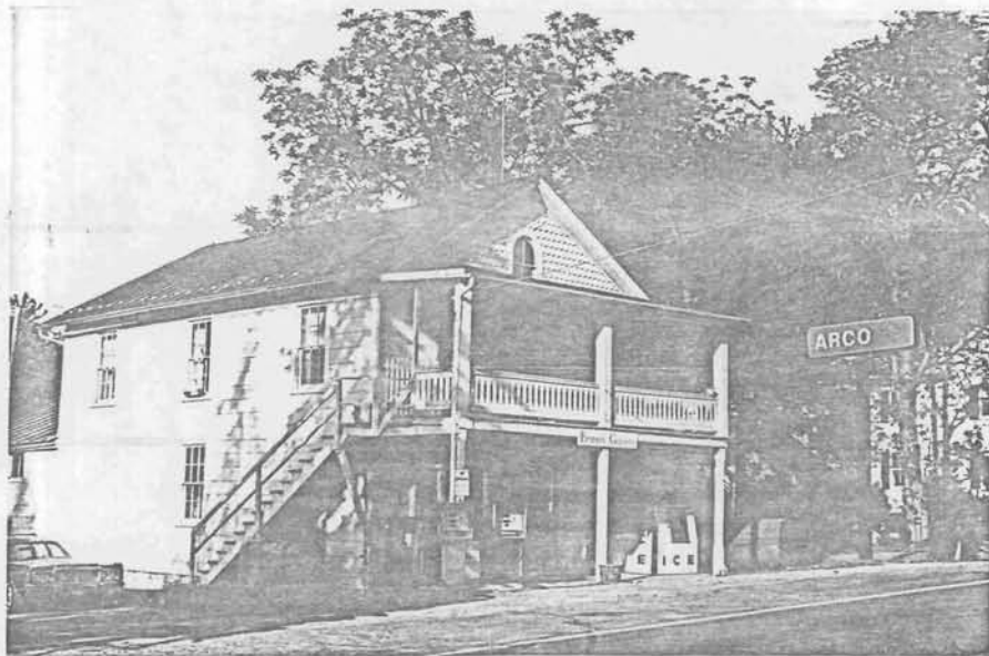
PARTLOW'S GROCERY. Turn of the Century Two Story Frame Gable Front Store and Dwelling with Shingled gable. Two story front gallery adds visual interest. 53-551 (3503)
