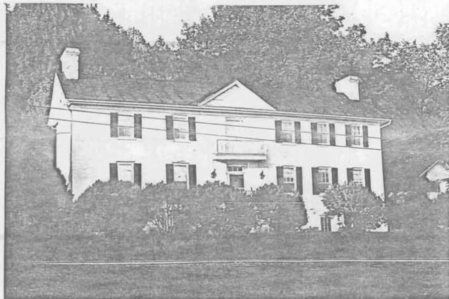
Early 1800's two story, probably Brick dwelling house now stuccoed. East end appears to have been added. Overall quality worthy of preservation. Important element to the east end approach of the village. 53-540 (3504)
