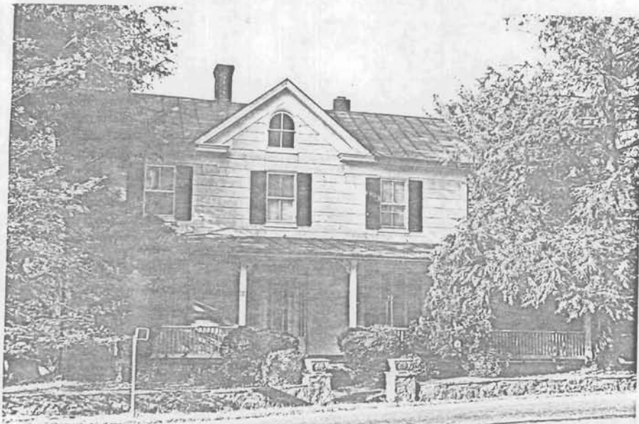
Turn of the Century Two Story Frame Dwelling with Cross Gable. Original Entrance Door and sidelights, as well as sash and shutters. In good state of preservation. 53-550 (3503)
