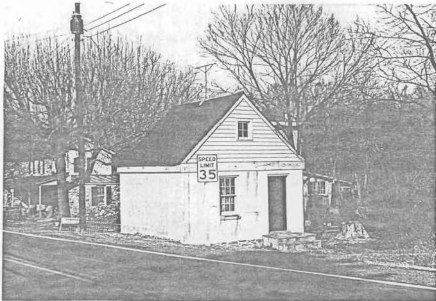
Good one story rural Village Wayside shop or office structure. Well preserved and maintained. Early to mid 1800's. 53-522 (3496)
