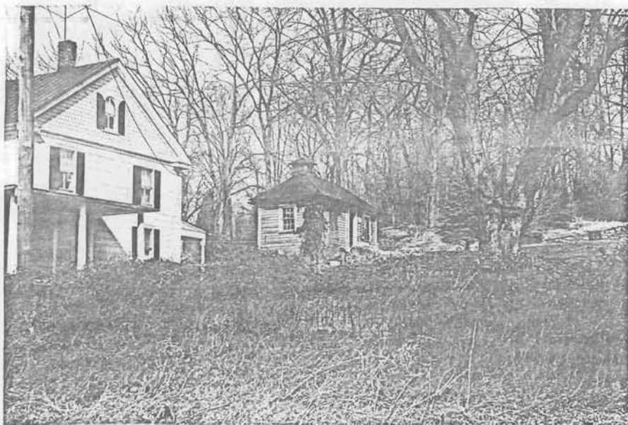
Interesting one story Frame outbuilding. Should be preserved for a suitable use and to retain visual interest. 53-538 (3497)
