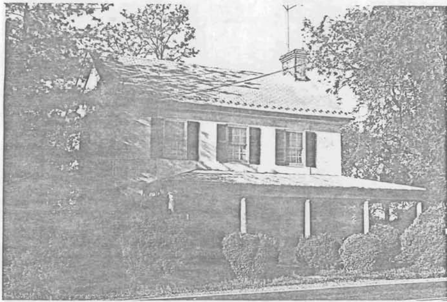
Early to mid 1800 Two Story Brick Dwelling. Good overall design and scale. First floor windows have been modified. 53-549A (3503)
