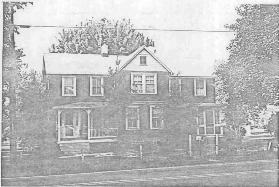
Two story Frame Residence on Rubble Stone foundation. Shingled Cross Gable. Pleasant entrance porches with Turned Posts. 53-545B (3503)
