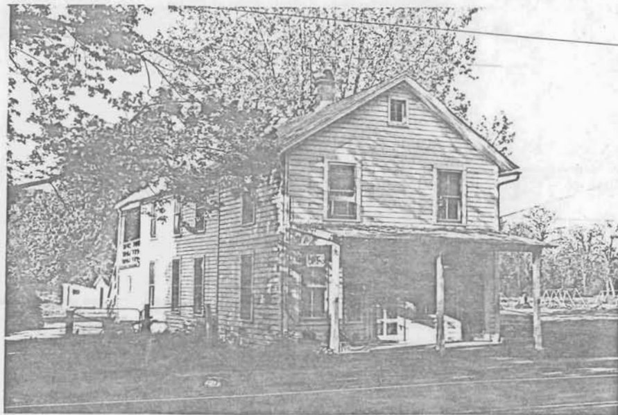
Two Story Frame Gable End Dwelling and Store. At one time used as a Drug Store. Built at the turn of the Century. 53-545C (3503)
