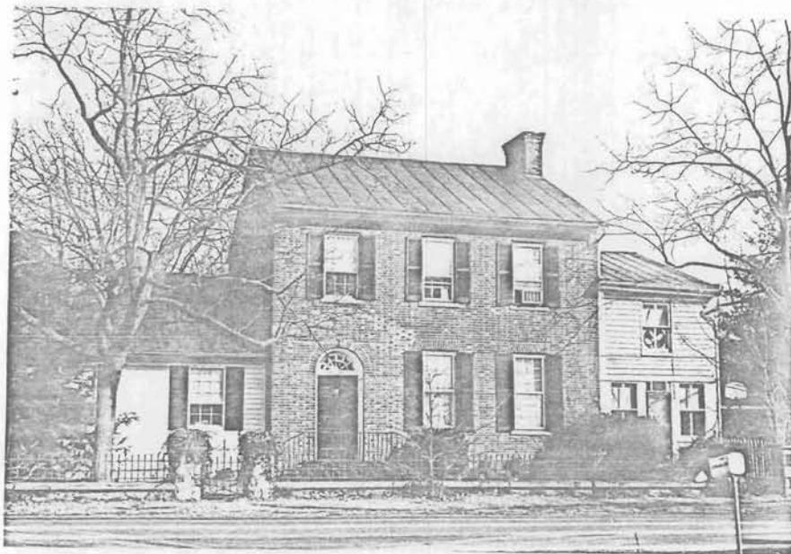
NARROW GATE. Early 1800 two story brick dwelling, with Flemish Bond Brickwork on the front facade. Later frame additions distract somewhat from the original, but the overall quality is good. 53-529 (3496)
