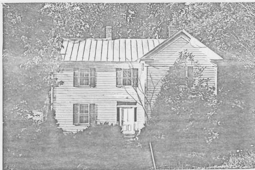
Two Story Frame Dwelling, built in the late 1800's. West section may have been built on the foundation of an earlier structure. Good scale and proportion, in good state of preservation. 53-552B (3503)
