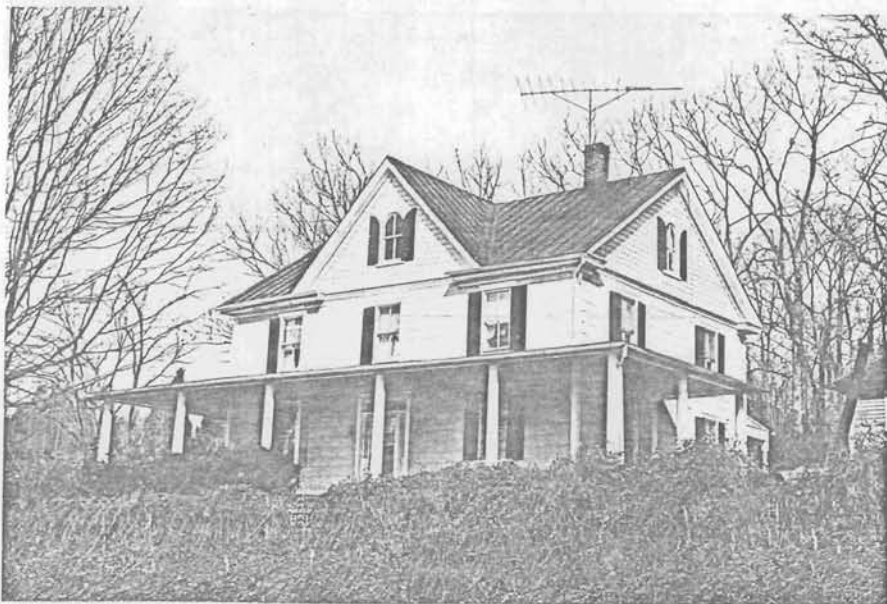
Excellent Two Story turn of the Century Frame Dwelling with predominate Cross Gable. Original sash, shutters, cornice and projecting gable design. Full wrap around one story porch. 53-538 (3497)
