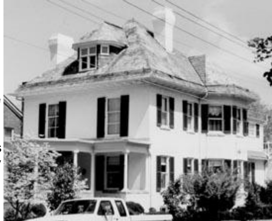
Owners of this Winchester home are replacing the slate roof a few pieces at a time over a number of years.
