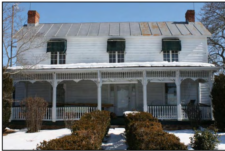
Figure 7- A two-story center-passage-plan form and a Victorian porch decorated with sawn and turned ornament are features of the house at 1770 Boxwood Farm Road (005-5138)
