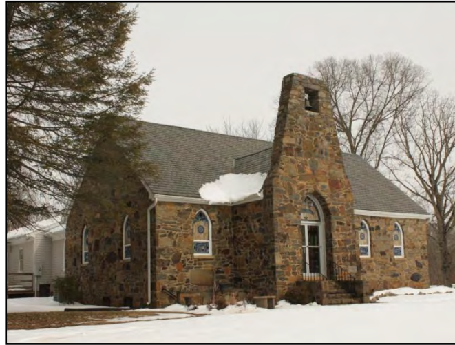
Figure 26- The architecturally sophisticated 1945 Poplar United Methodist Church (005-5140) features artistic stonework and an unusual bell tower.
