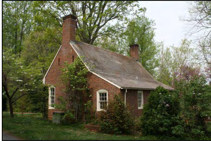
Figure 8- The Patch, a Colonial Revival style house (005-5315)
