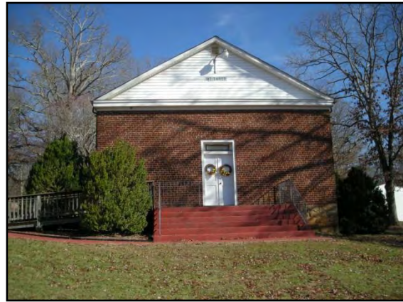
Figure 25- The antebellum Mt. Tabor United Methodist Church (005-5008) illustrates locally progressive brick construction of the era but retention of a simple gable-fronted nave form.
