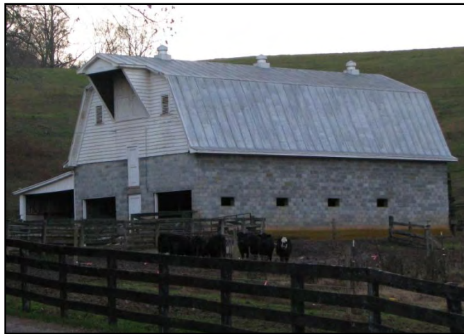
Figure 13- A gambrel-roofed barn (005-5075)
