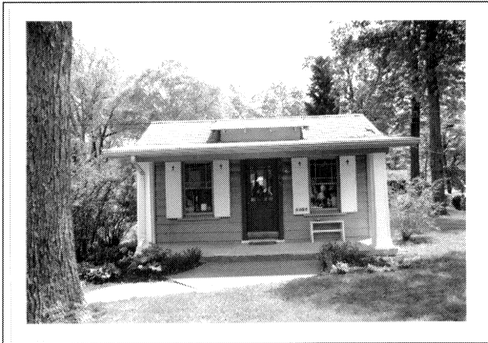
Figure 72: Real Estate Office at 2303 South Oakcrest Road (00-1199)
