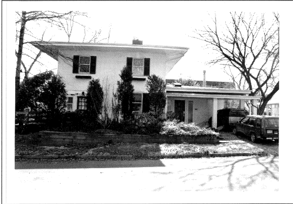
Figure 36: House at 722 South 22nd Street (00-610)
