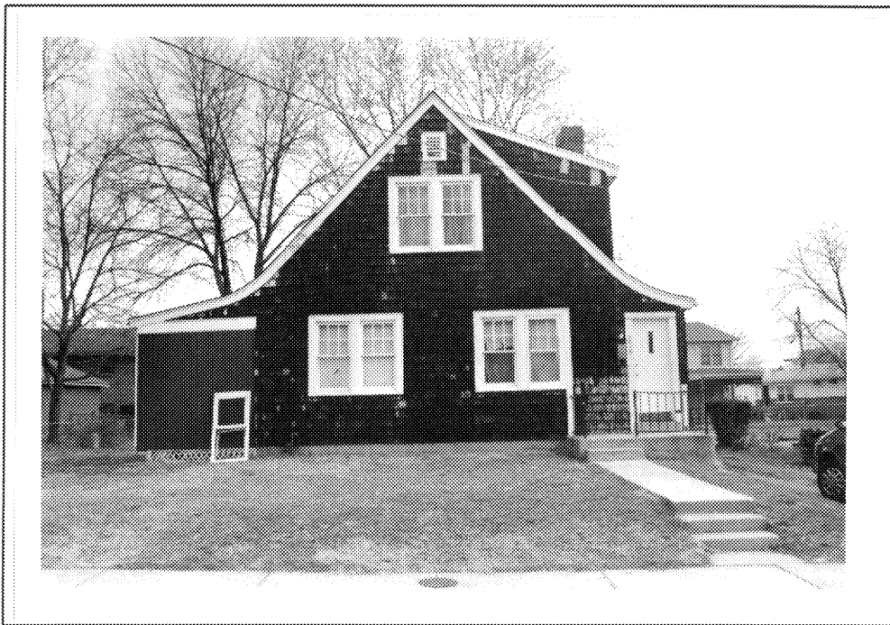
Figure 87: House 1010 South Rolfe Street (00-518)
