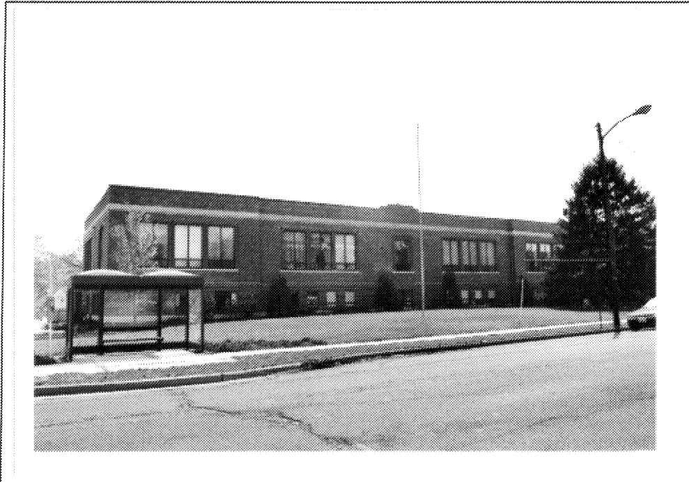
Figure 61: Nellie Custis School at 750 South 23rd Street (00-1133)
