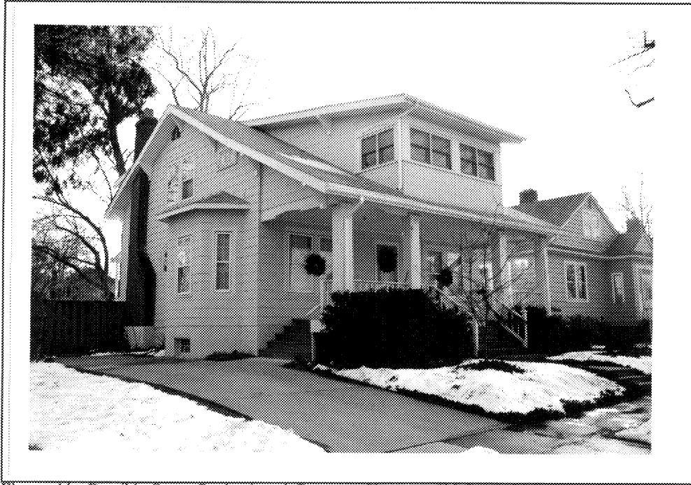
Figure 44: Possible Sears, Roebuck and Company House at 620 South 24th Street (00-586)
