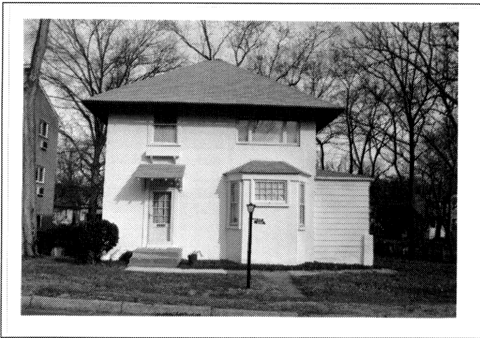
Figure 95: House at 633 South 22nd Street (00-595)
