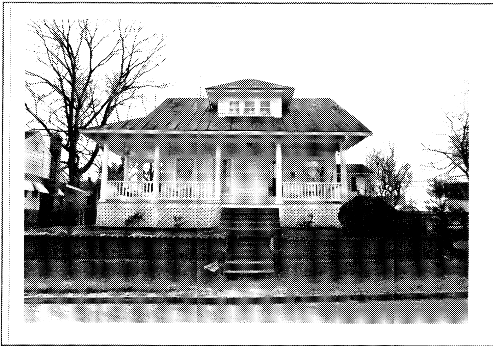
Figure 30: House at 640 South 22nd Street (00-594)
