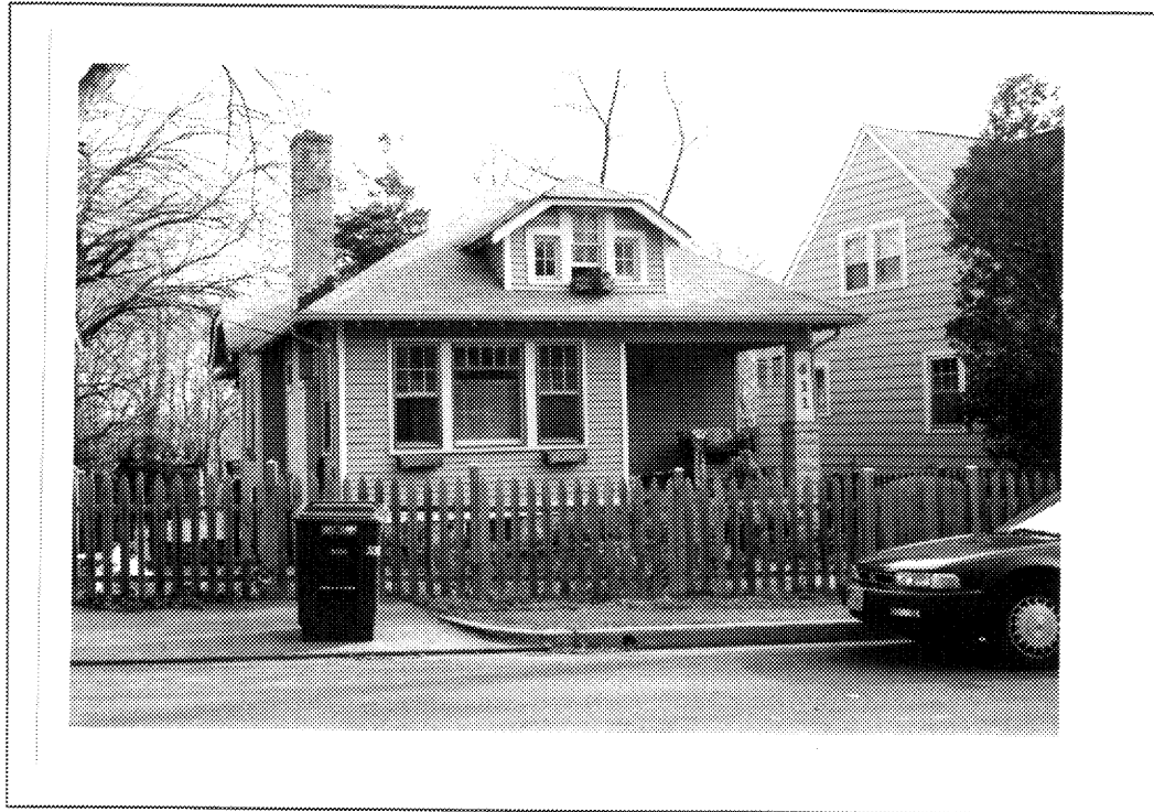
Figure 34: House, 411 North Cleveland Street (000-5092)
