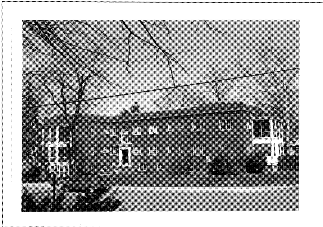
Figure 9: The Irving Apartment Building, 605 North Irving Street (000-5603)
