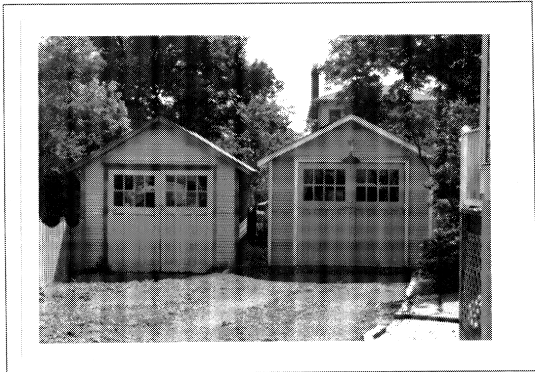
Figure 17: Garages at 803 and 805 North Danville Street (000-5219 and 000-5221)
