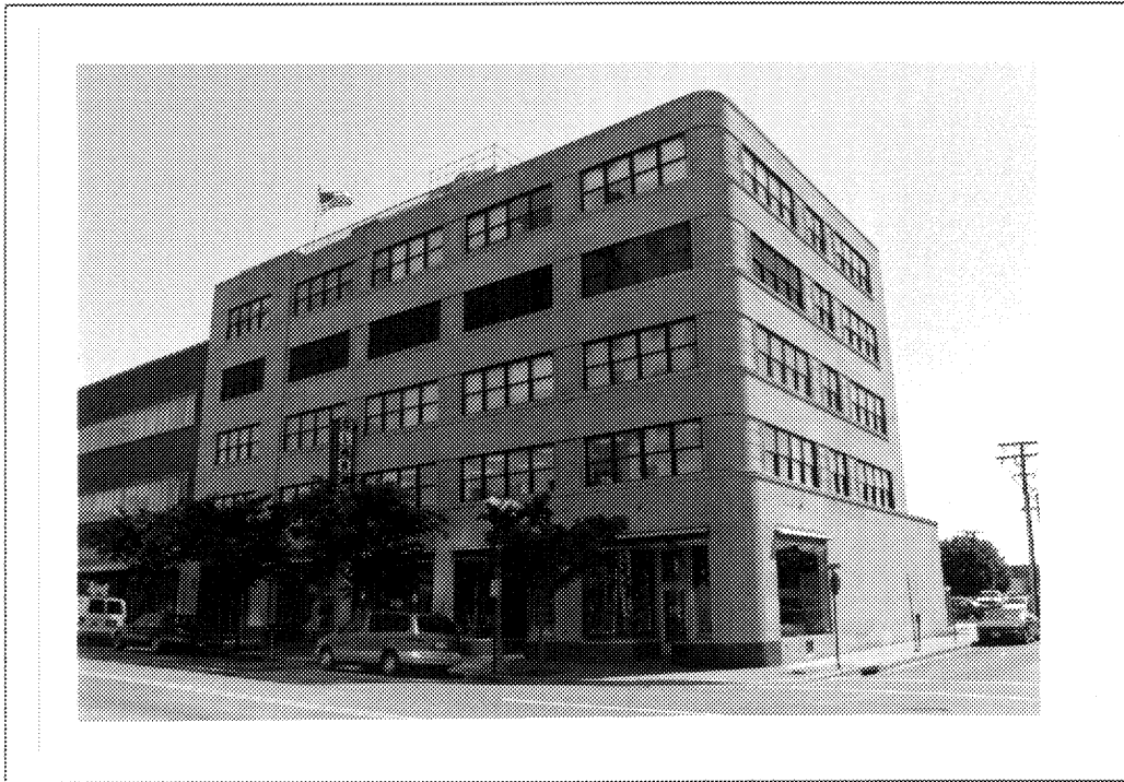
Figure 12: Old Dominion Building, 1101 North Highland Street (000-023-0005)
