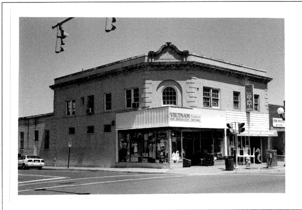
Figure 11: The Rees Building, 3153-3157 Wilson Boulevard (000-023-0022)
