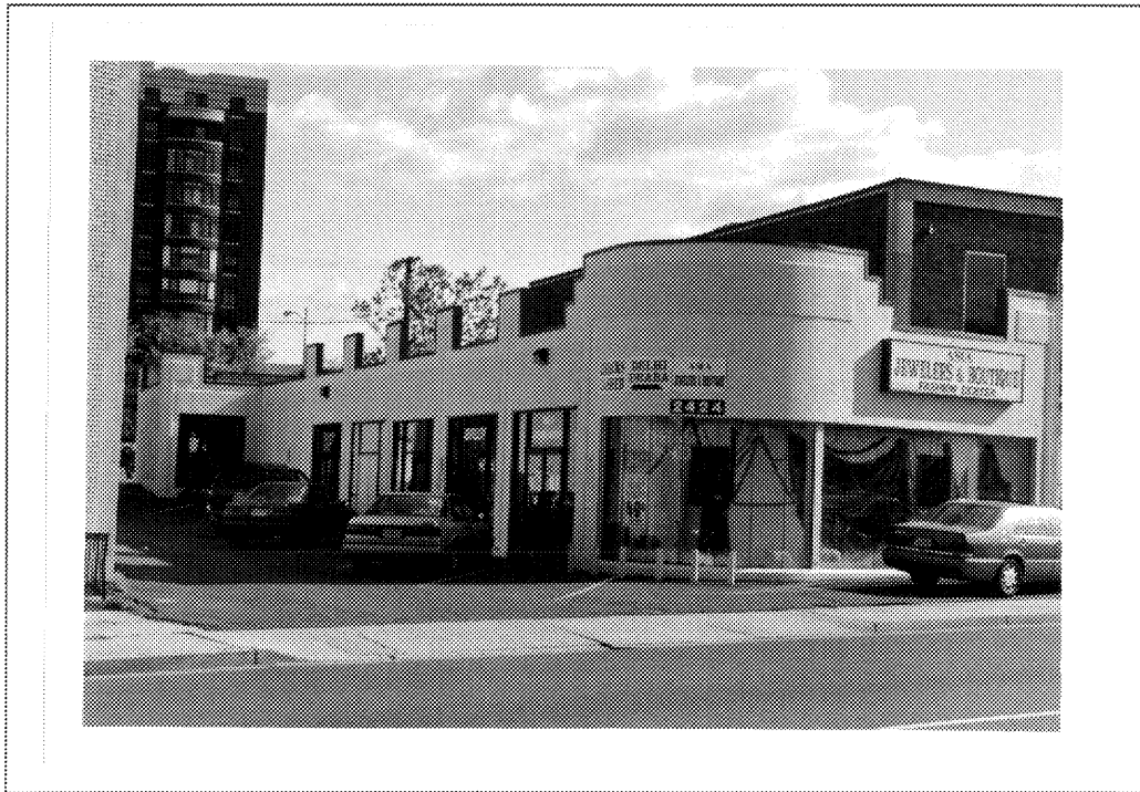
Figure 7: Commercial Building, 2424 Wilson Boulevard (000-6444)
