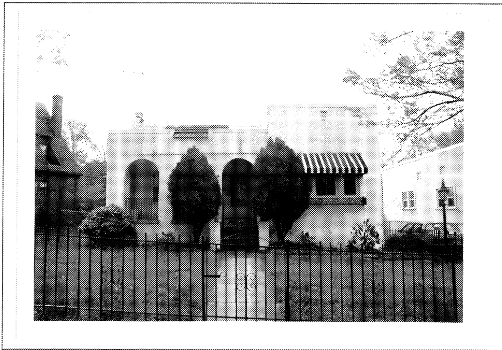
Figure 5: House, 3108 Key Boulevard (000-6283)
