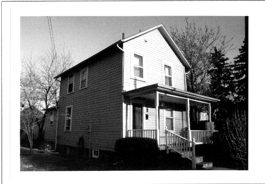
Figure 13: House at 1201 North Danville Street (000-5942)
