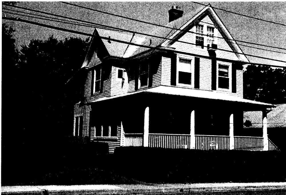
Figure 3: House at 1414 North Jackson Street (000-7305)
