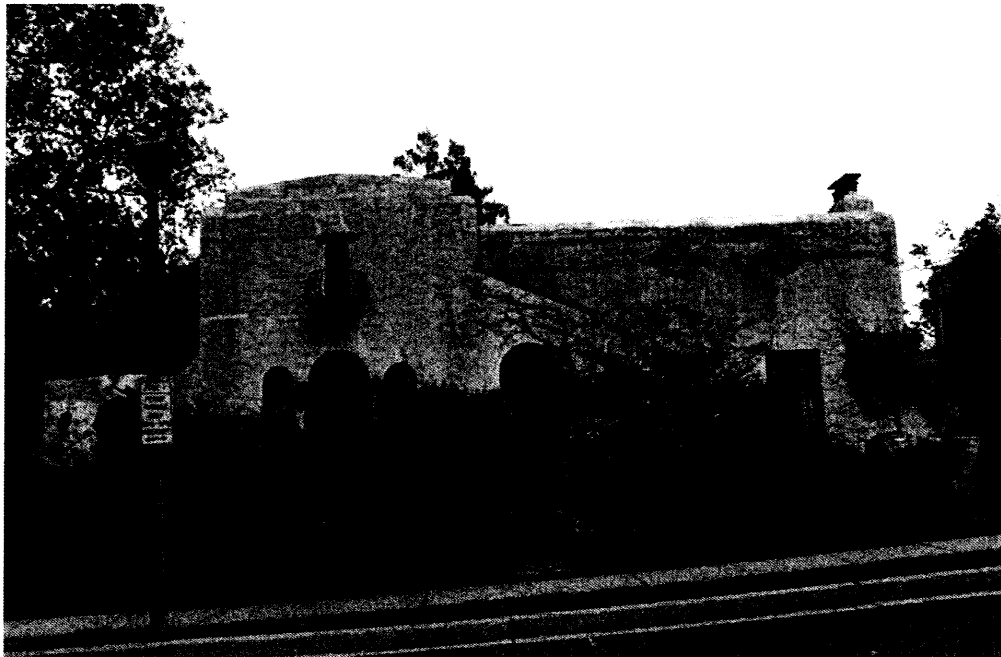
Figure 10: House at 1611 North Highland Street (000-7095)
