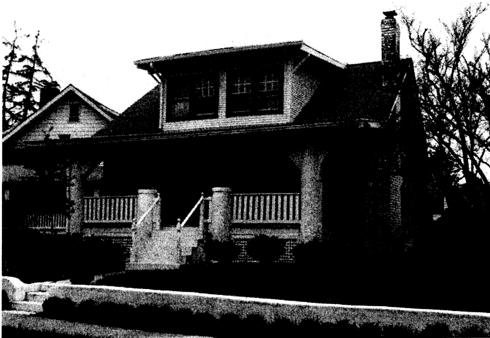
Figure 9: House at 264 North 18 th Street (000-7030)
