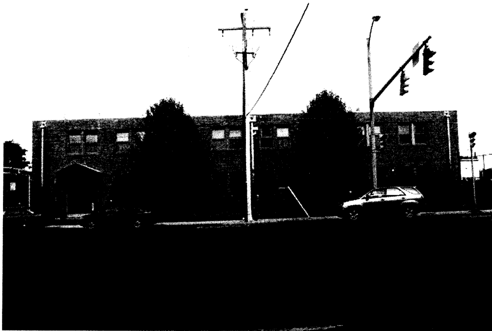
Figure 37: Washington Metropolitan Area Transit Authority Complex (000-7368)
