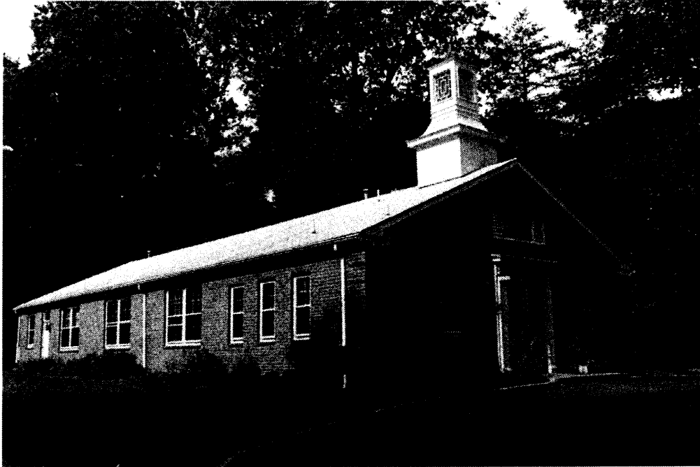
Figure 36: Lyon Village Community House (000-7124)
