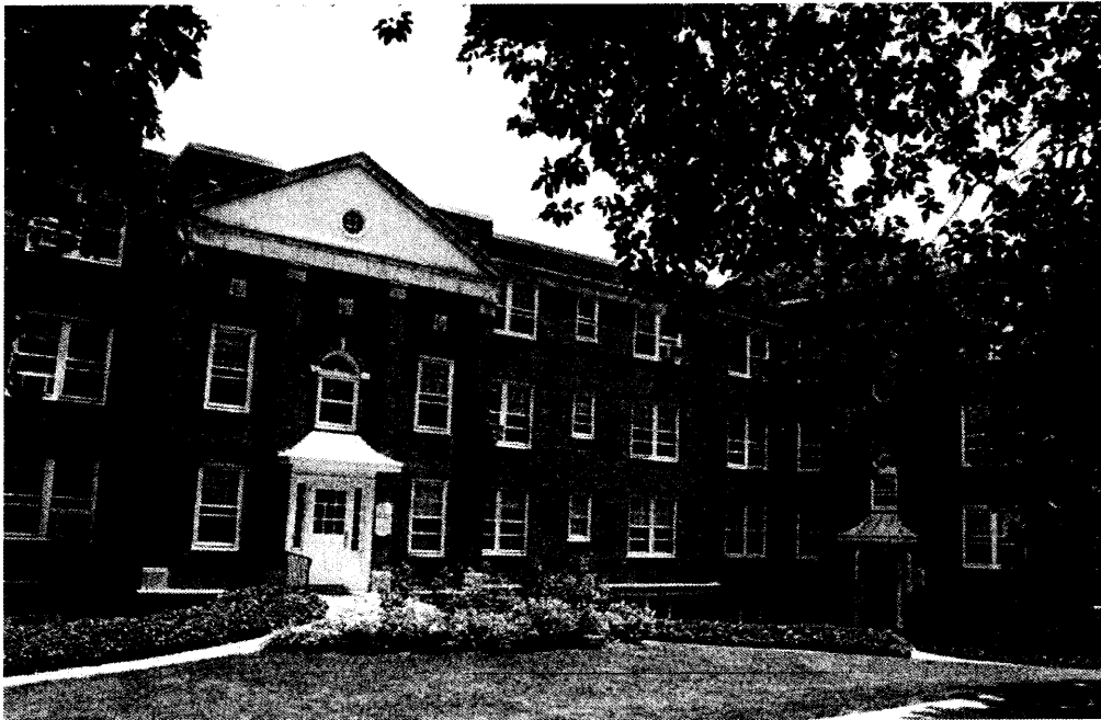
Figure 29: Lyon Village Apartments (000-7289)
