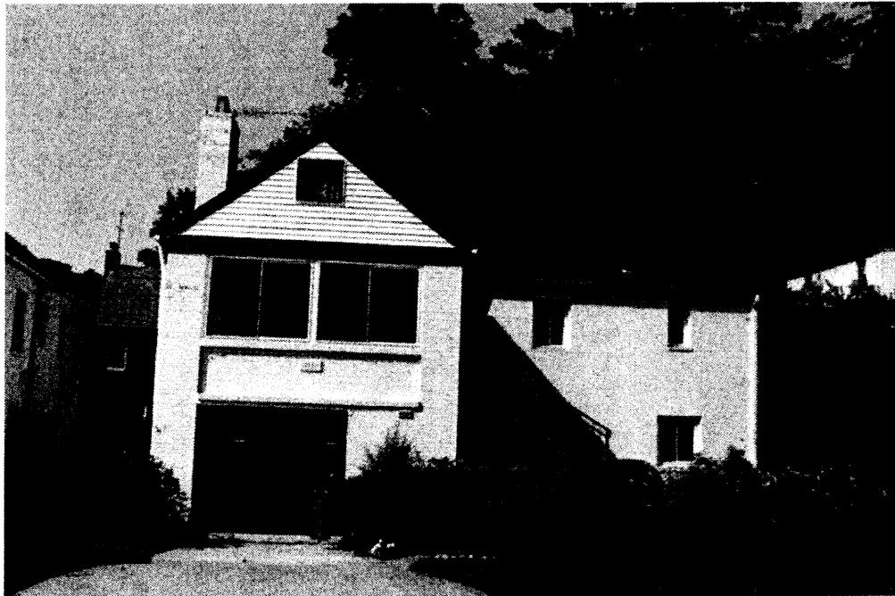
Figure 14: House at 3211 North 19 th Street (000-7298)
