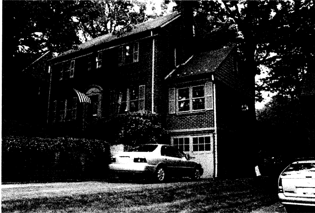
Figure 24: House at 3170 North 18 th Street (000-7237)
