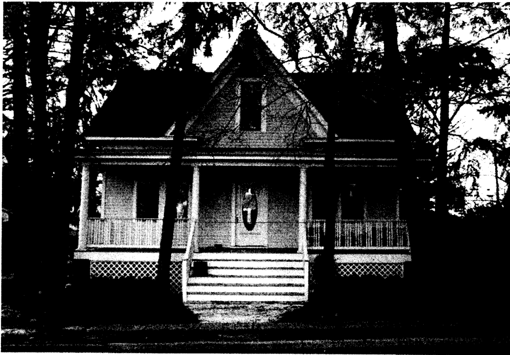
Figure 1: House at 812 North Jackson Street (000-6687)
