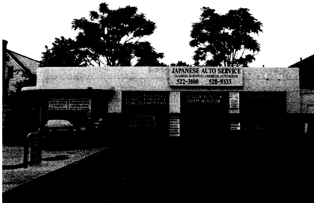
Figure 18: Gas Station at 3413 Wilson Boulevard (000-7391)
