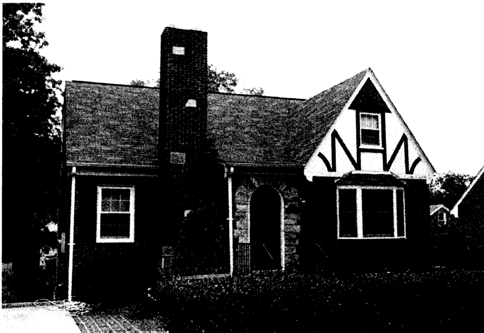
Figure 8: House at 3107 North 18 th Street (000-7113)
