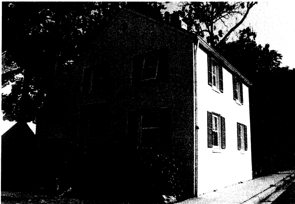
Figure 25: House at 3214 North 19 th Street (000-7300)
