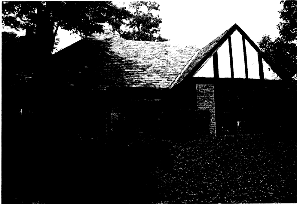
Figure 7: House at 1622 North Highland Street (000-7099)
