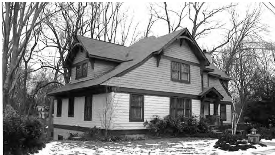
Figure 8: House, 4507 37th Place, North, 000-9207 (EHT Tracerics, 2004)
