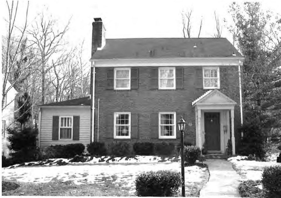
Figure 3: House, 4460 38th Street, North, 000-9199 (EHT Tracerics, 2004)
