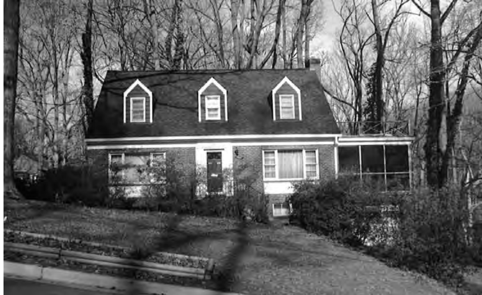
Figure 15: House, 3882 30th Street, North, 000-9510 (EHT Tracerics, 2004)
