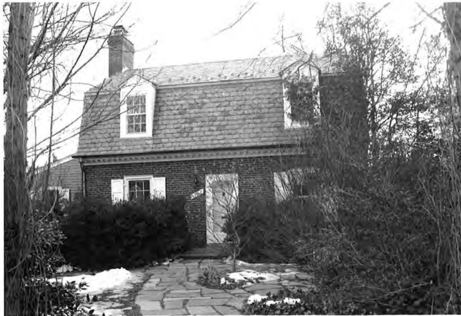
Figure 5: House, 3822 North Vernon Street, 000-9238 (EHT Tracerics, 2004)
