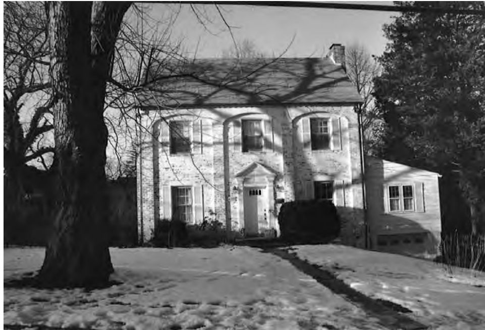
Figure 16: House, 4701 37 th Street, North, 000-9120 (EHT Tracerics, 2004)
