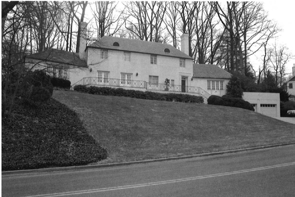
Figure 8: House, 3323 North Woodrow Street, 000-2440 (EHT Tracerics, 2004)
