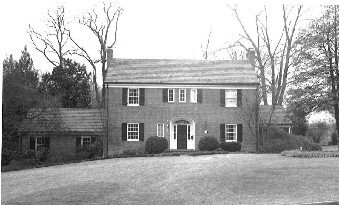
Figure 22: House, 3401 North Albemarle Street, 000-2816 (EHT Tracerics, 2004)
