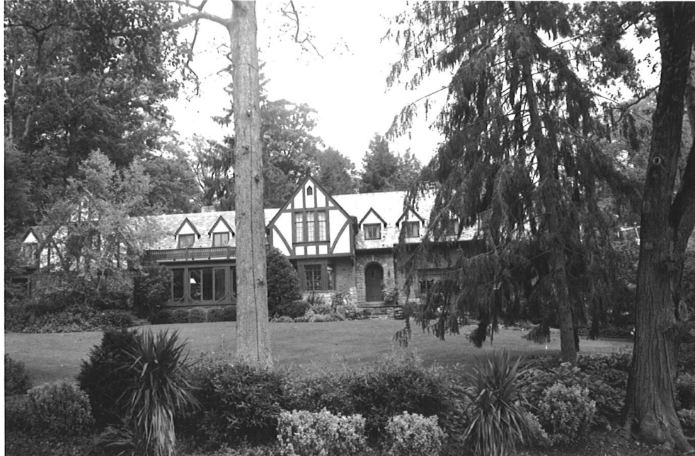
Figure 10: House, 4605 Rock Spring Road, 000-3306 (EHT Tracerics, 2004)
