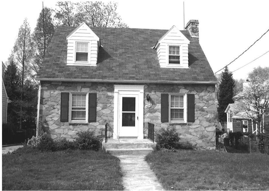
Figure 21: House, 1676 North Longfellow Street, 000-3079 (EHT Tracerics, 2004)
