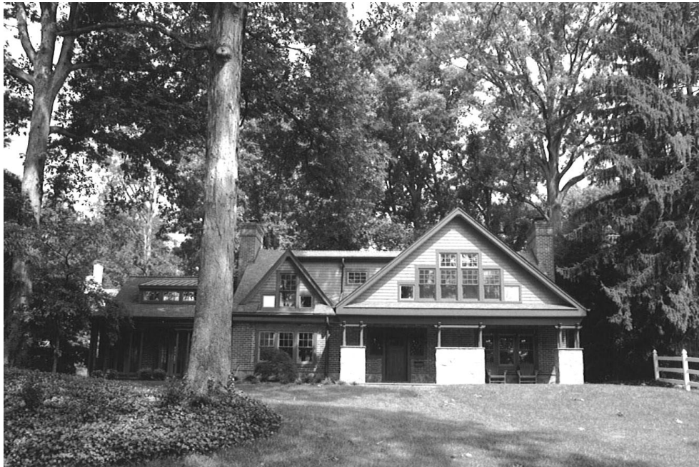
Figure 13: House, 4511 Rock Spring Road, 000-3308 (EHT Tracerics, 2004)
