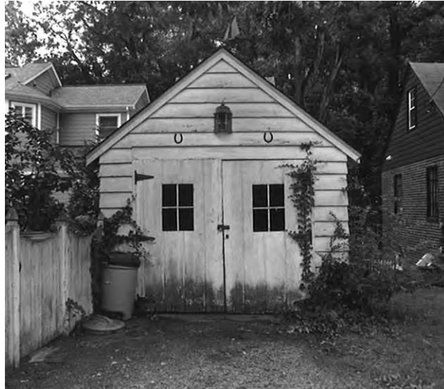
Figure 37: Garage, 4910 25 th Street North, 000-3806 (EHT Tracerics, 2006)
