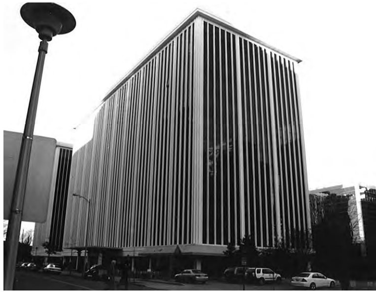
Figure 19: Oakhill Office Building, 1401 Wilson Boulevard, 000-3422 (EHT Tracerics, 2006)
