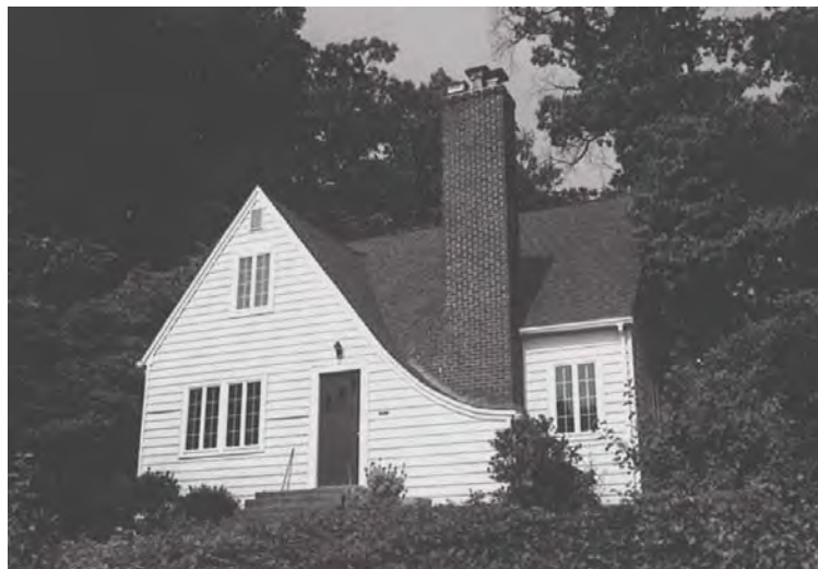
Figure 11: Single Dwelling, 2370 North Oakland Street, 000-3750 (EHT Tracerics, 2006)
