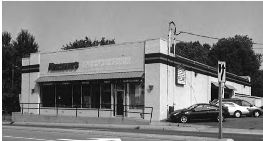
Figure 23: Commercial Building, 4801 Lee Highway, 000-3389 (EHT Tracerics, 2006)
