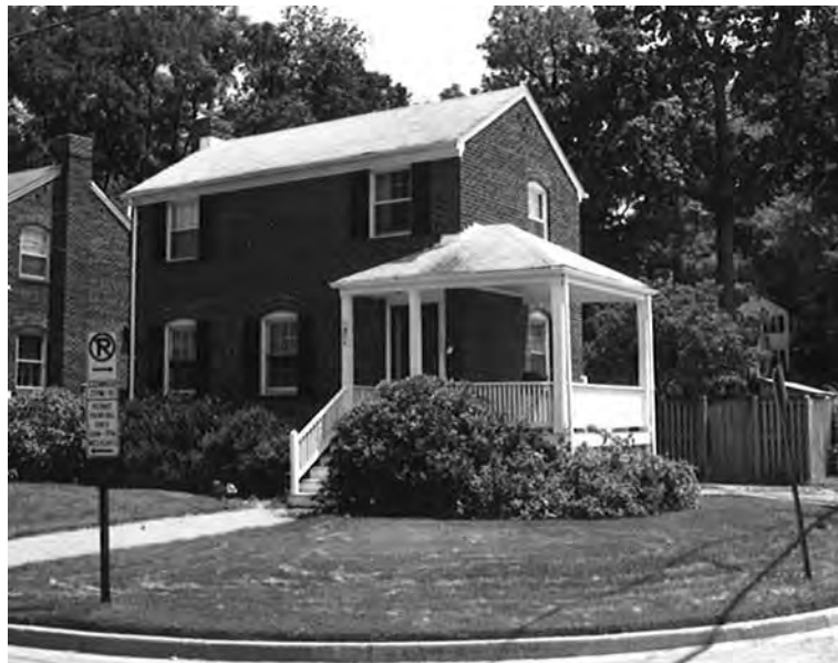
Figure 30: Single Dwelling, 5222 27th Road North, 000-4011 (EHT Tracerics, 2006)
