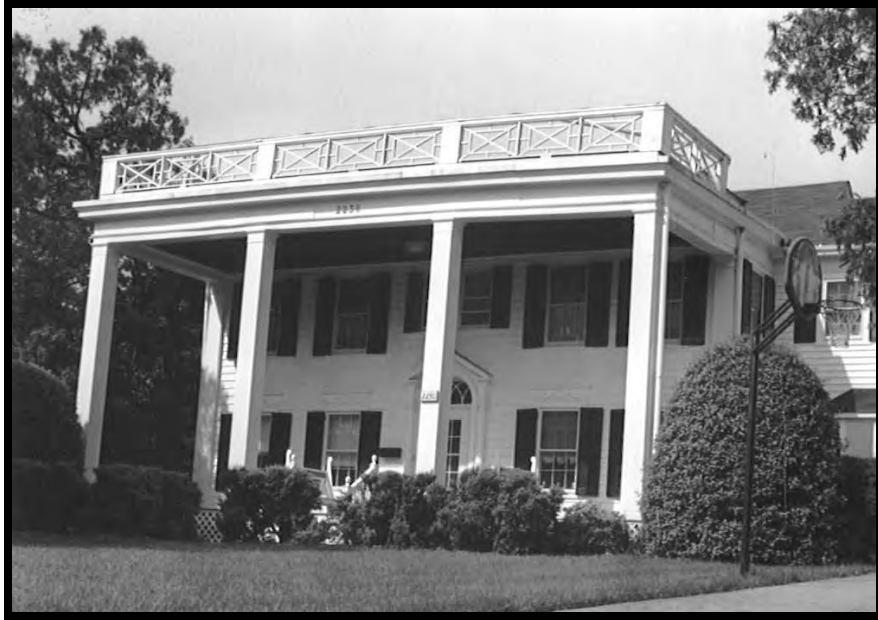
Figure 2: Single Dwelling, 2230 North Powhatan Street, 000-4209-0012 (EHT Tracerics, 2008)
