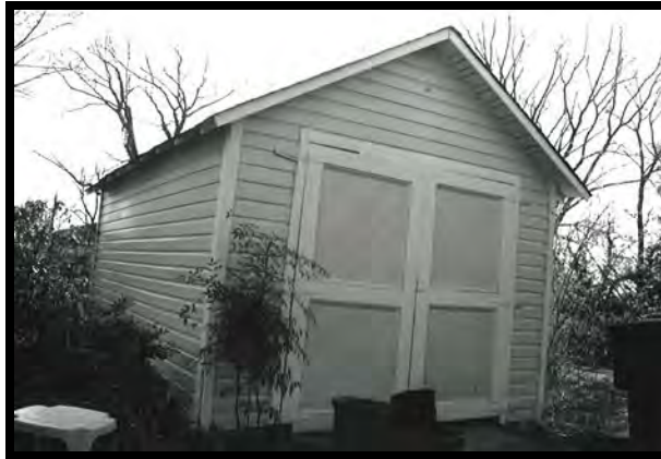
Figure 53: Garage, 3416 North Glebe Road, 000-4206-0091 (EHT Tracerics, 2008)
