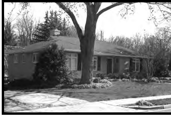
Figure 20: Single Dwelling, 3401 North George Mason Drive, 000-4206-0017 (EHT Tracerics 2008)
