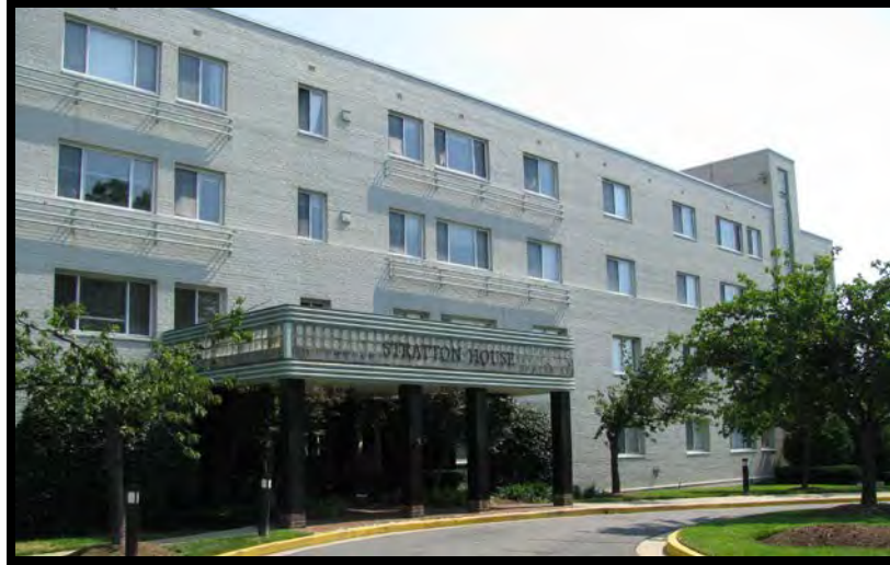
Figure 51: Apartment Building, 3601 5th Street South, 000-4216 (EHT Tracerics, 2008)
