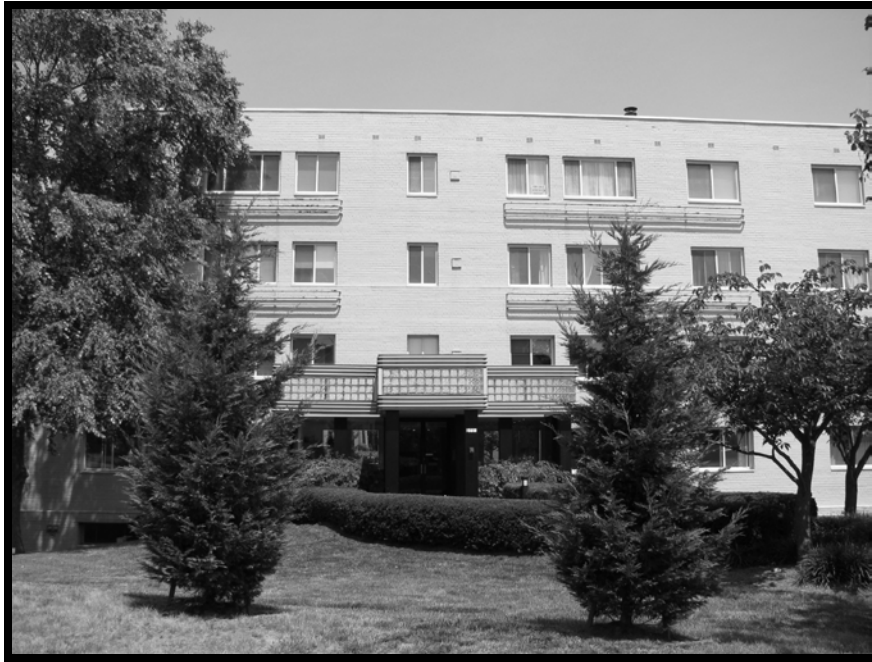
Figure 19: Apartment Building, 3701 5th Street South, 000-4217 (EHT Tracerics, 2008)
