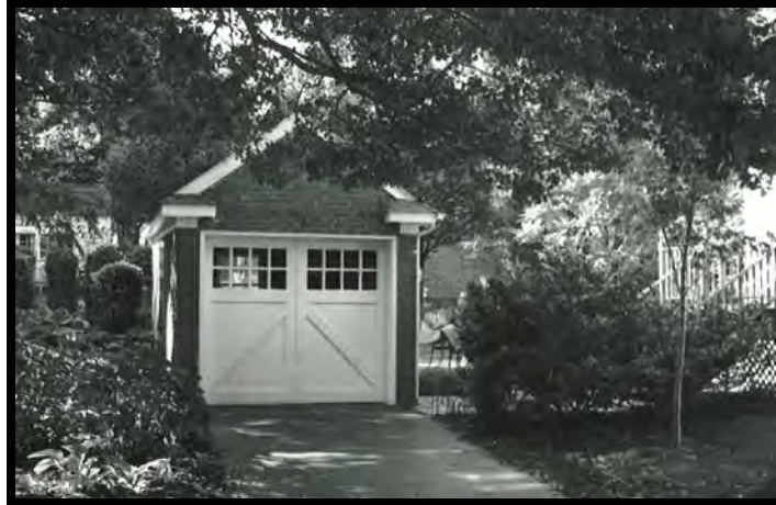
Figure 54: Garage, 2302 North Powhatan Street, 000-4209-0018 (EHT Tracerics, 2008)
