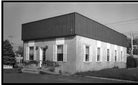
Figure 30: Commercial Building, 5800 Lee Highway, 000-4209-0060 (EHT Tracerics, 2008)
