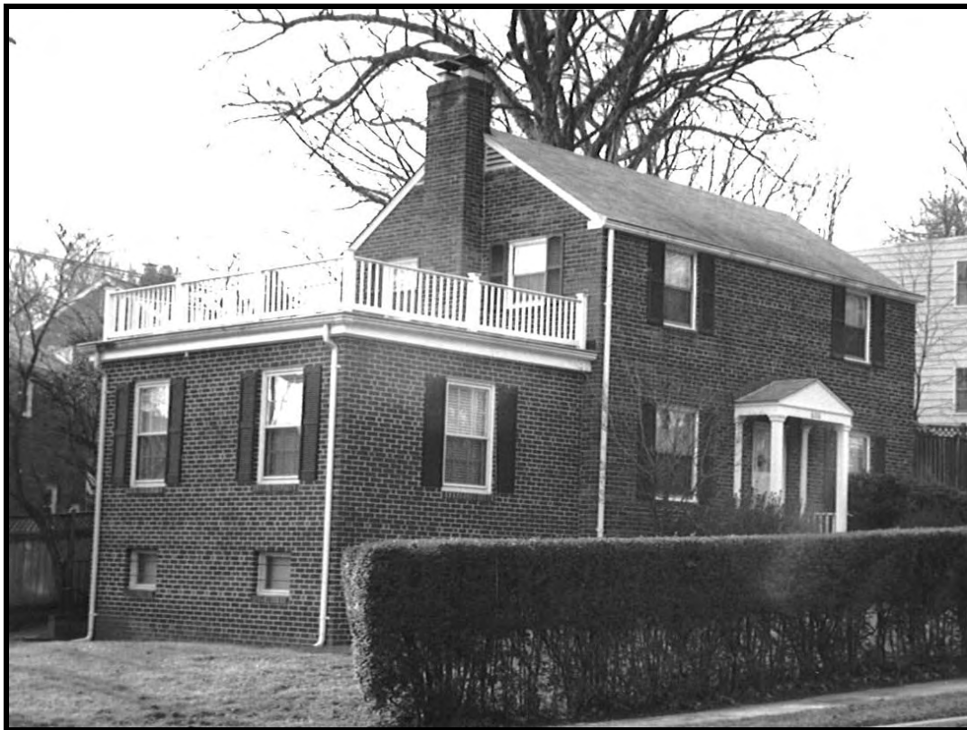
Figure 8: Single Dwelling at 6100 11 th Road North, 000-4212-0056 (EHT Tracerics, 2009)
