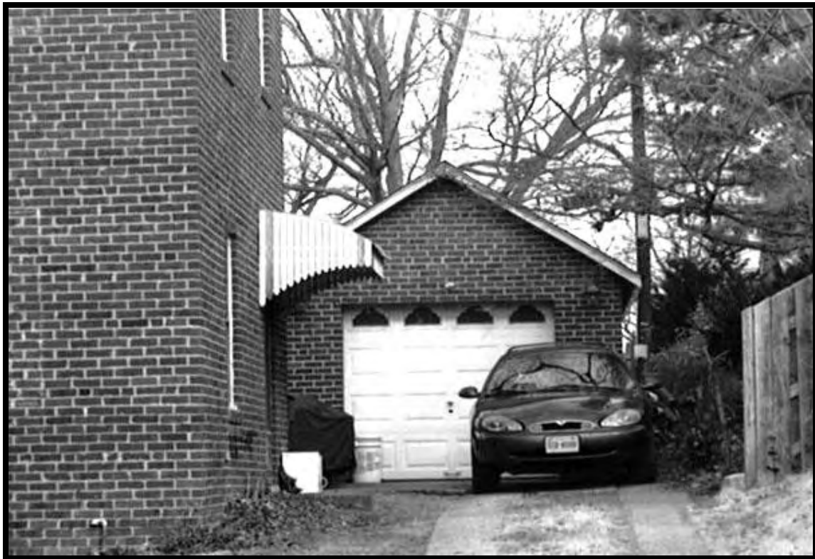
Figure 43: Garage, 6157 11 th Road North, 000-4211-0013 (EHT Tracerics, 2009)
