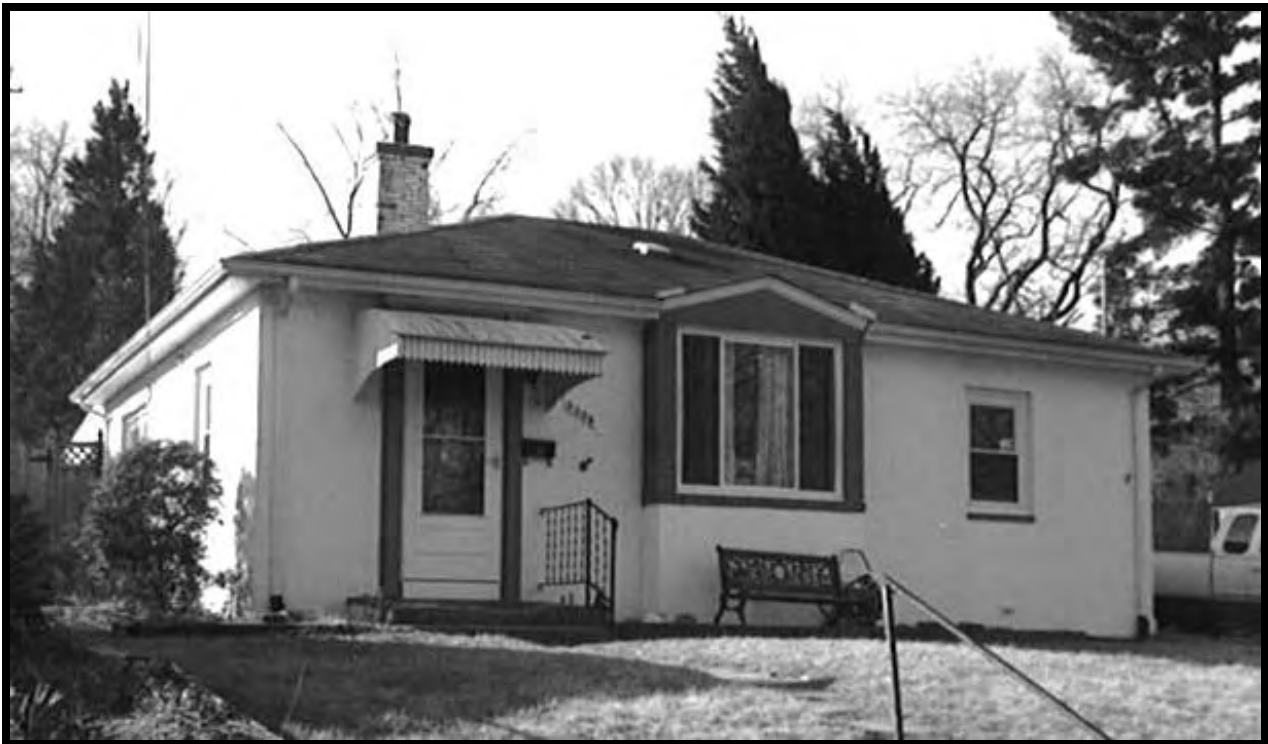
Figure 34: Single Dwelling, 6604 16 th Street North, 000-4208-0032 (EHT Tracerics, 2009)
