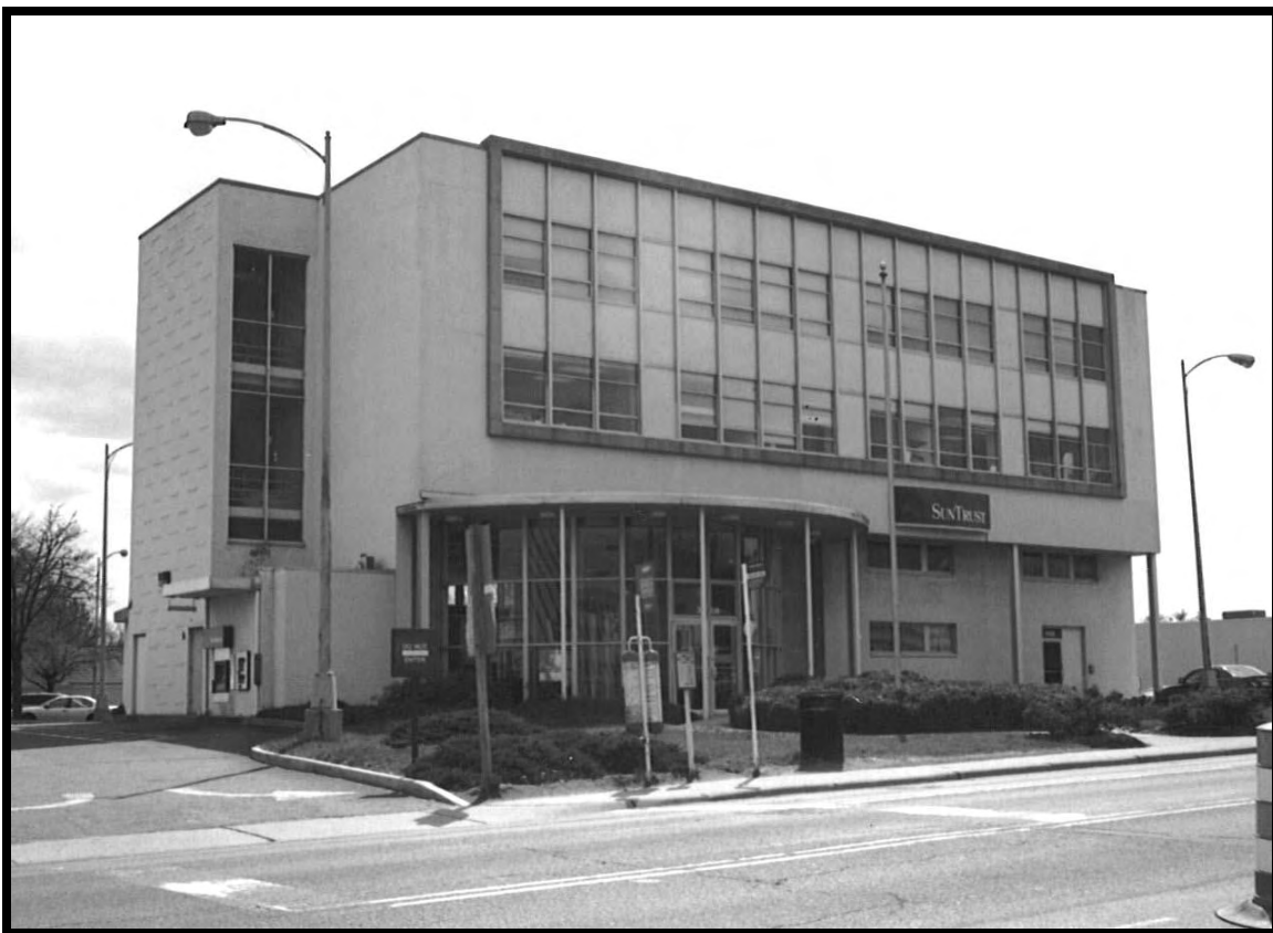
Figure 47: First Federal Savings & Loan Association Building, 3108 Columbia Pike, 000-4213 (EHT Tracerics, 2009)
