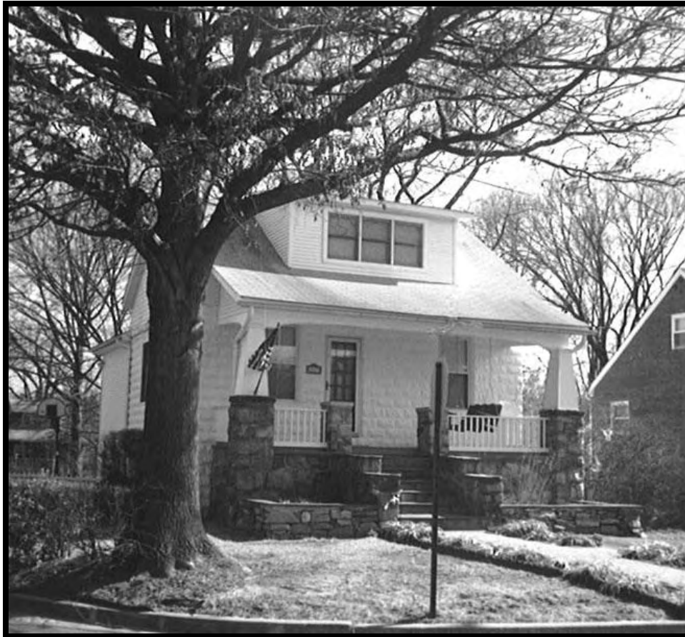
Figure 23: Single Dwelling, 1827 North Underwood Street, 000-4208-0058 (EHT Tracerics, 2009)
