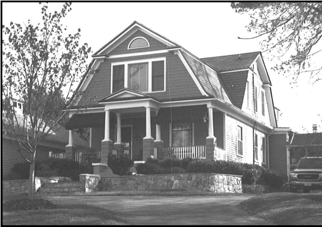
Figure 14: Single Dwelling, 2415 North Underwood Street, 000-4208-0203 (EHT Tracerics, 2009)
