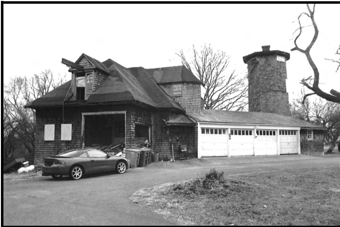
Figure 54: Barn, façade, 6407 Wilson Boulevard, 000-5796 (EHT Tracerics, 2009)
