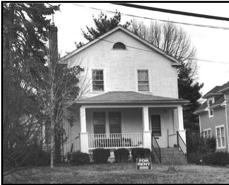
Figure 30: Single Dwelling, 6311 Washington Boulevard, 000-4208-0180 (EHT Tracerics, 2009)
