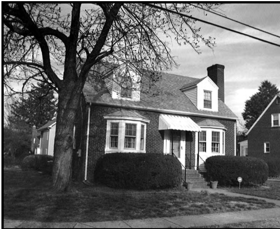
Figure 33: Single Dwelling, 743 North Edison Street (1942), 000-4214-0299 (EHT Tracerics, 2009)
