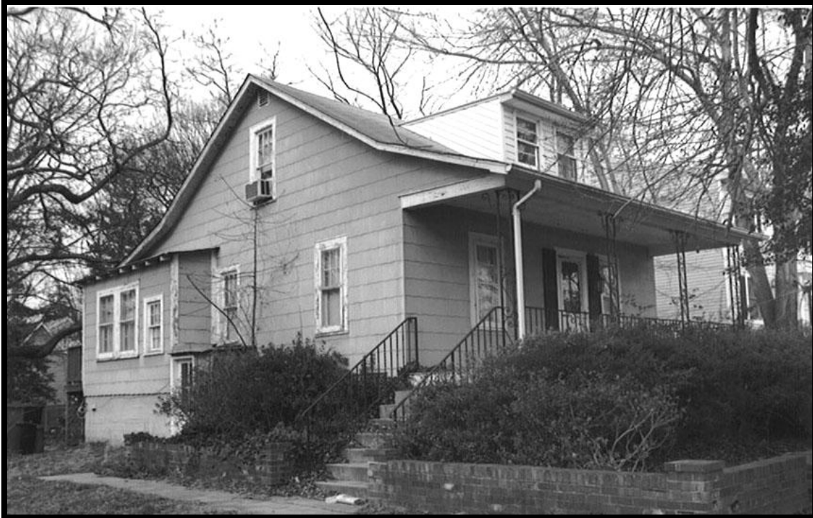
Figure 20: Single Dwelling, 1800 North Tuckahoe Street, 000-4208-0052 (EHT Tracerics, 2009)
