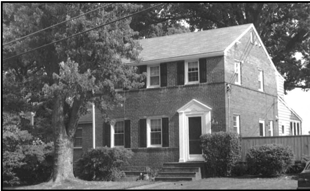
Figure 5: Single Dwelling at 5998 9 th Street North, 000-4212-0310 (EHT Tracerics, 2009)
