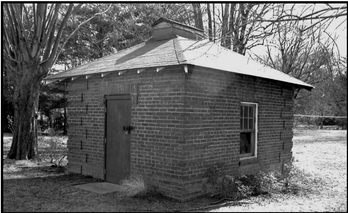
Figure 56: Pump House, 6700 18th Street North (000-4208-0055) (EHT Tracerics, 2009)
