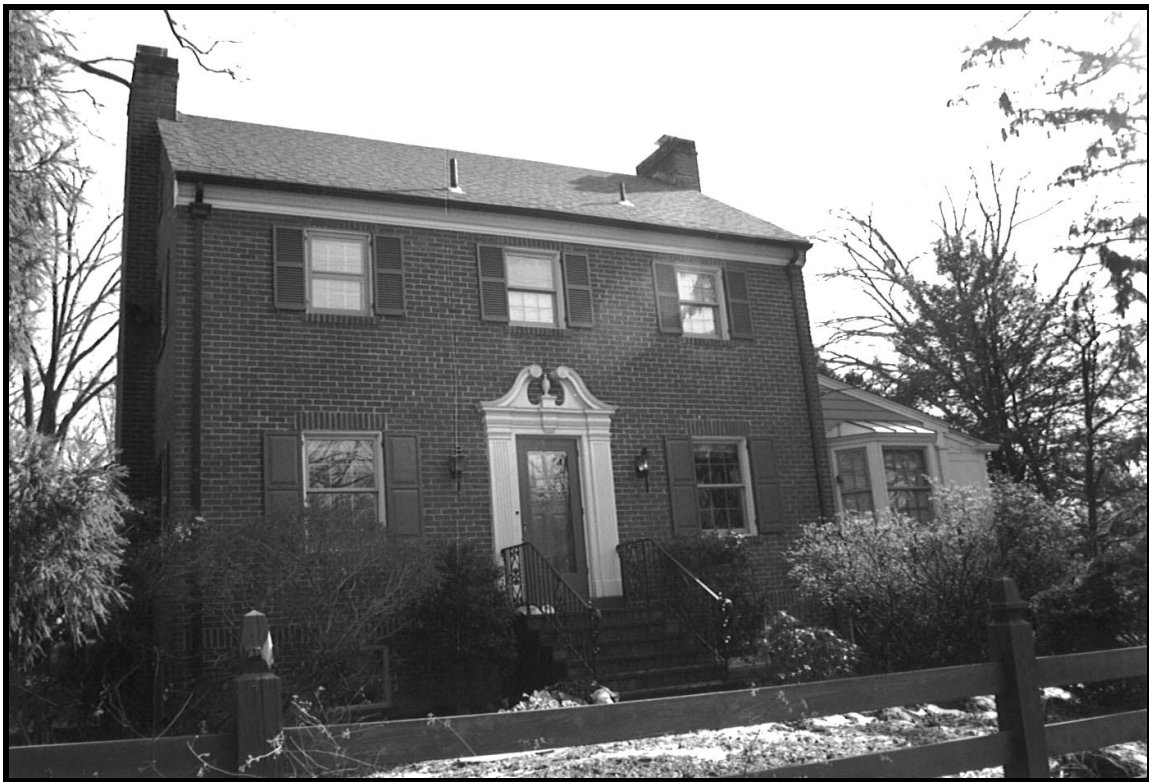
Figure 11: Single Dwelling, 5416 Washington Boulevard, 000-4214-0046 (EHT Tracerics, 2009)
