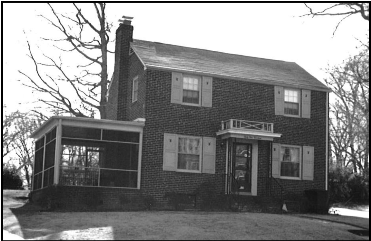
Figure 9: Single Dwelling at 6114 11 th Road North, 000-4212-0059 (EHT Tracerics, 2009)
