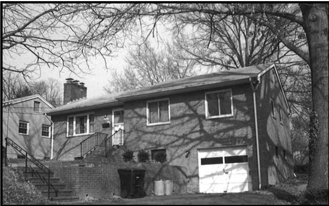
Figure 24: Single Dwelling, 2207 North Nottingham Street, 000-9703-0682 (EHT Tracerics, 2009)
