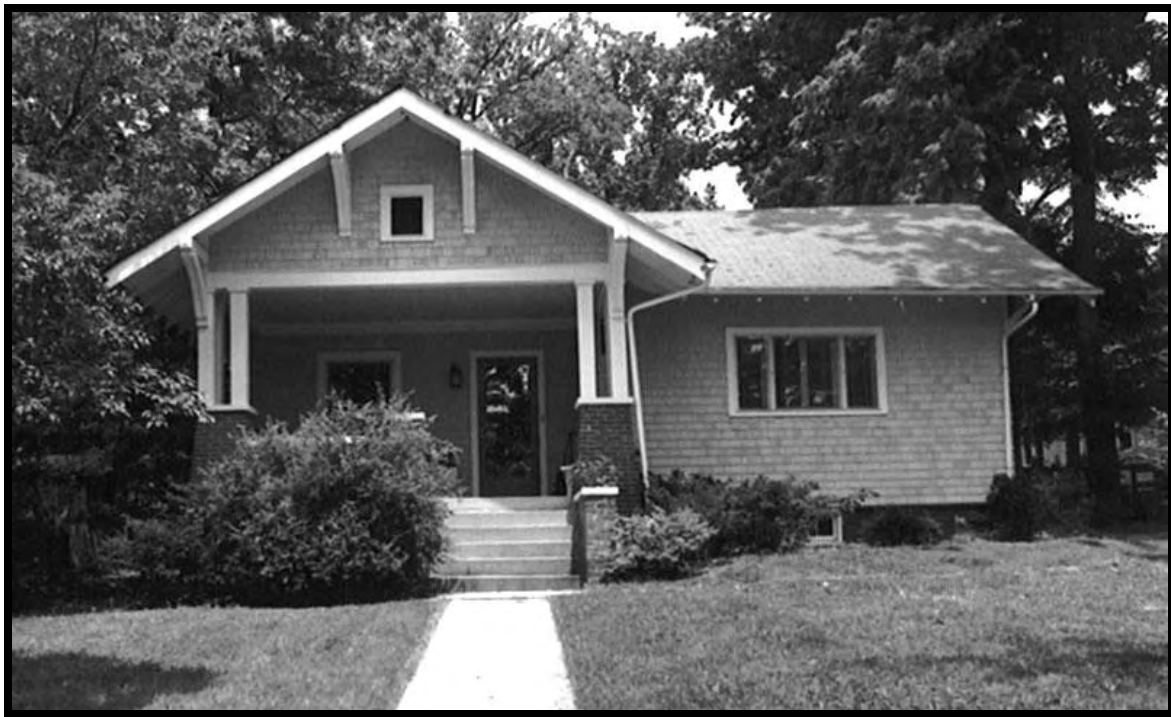
Figure 21: Single Dwelling, 6871 Washington Boulevard, 000-4208-0302 (EHT Tracerics, 2009)
