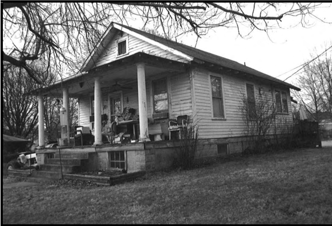
Figure 19: Single Dwelling, 1910 North Tuckahoe Street, 000-4208-0044 (EHT Tracerics, 2009)
