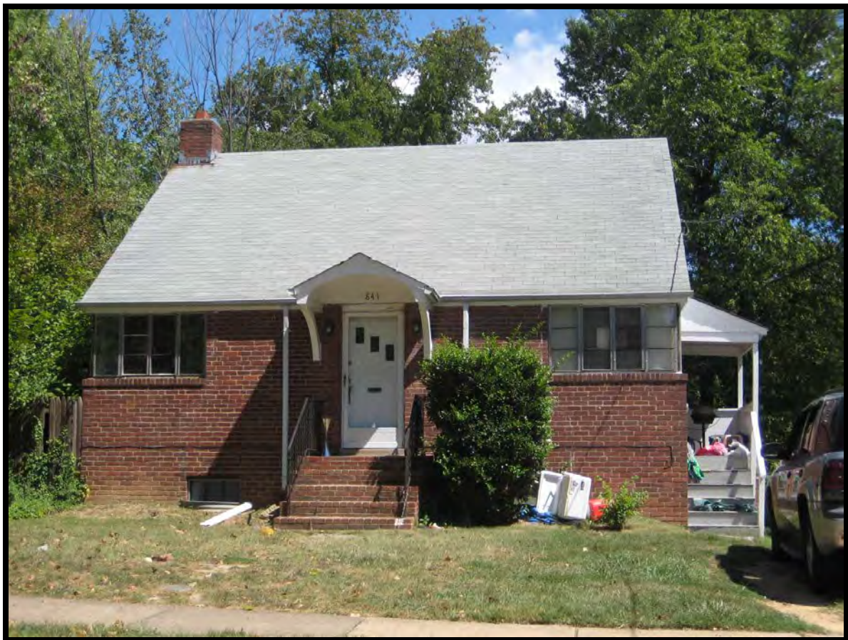
Figure 10: Single Dwelling, 847 North Jefferson Street, 000-4214-0372 (EHT Tracerics, 2010)
