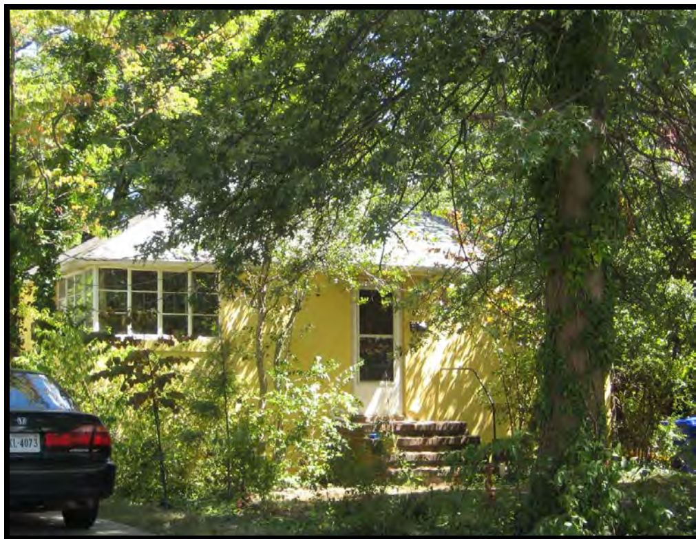
Figure 17: Single Dwelling, 851 North Jefferson Street, 000-4214-0373, (EHT Tracerics, 2010)
