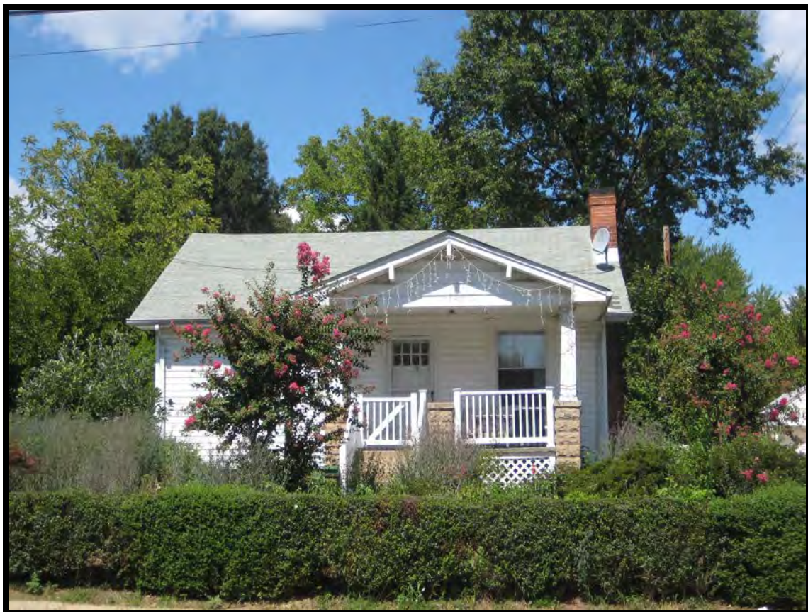
Figure 8: Single Dwelling, 5503 Wilson Boulevard, 000-4214-0369 (EHT Tracerics, 2010)
