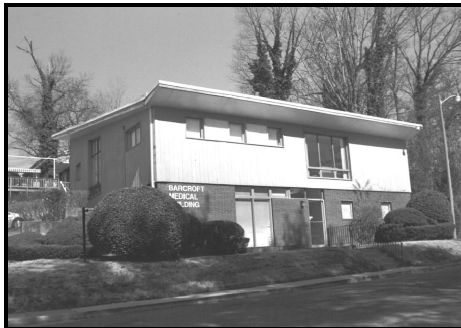
Figure 23: Barcroft Medical Building, 939 South Wakefield Street, 000-7818-0420 (EHT Tracerics, 2012)
