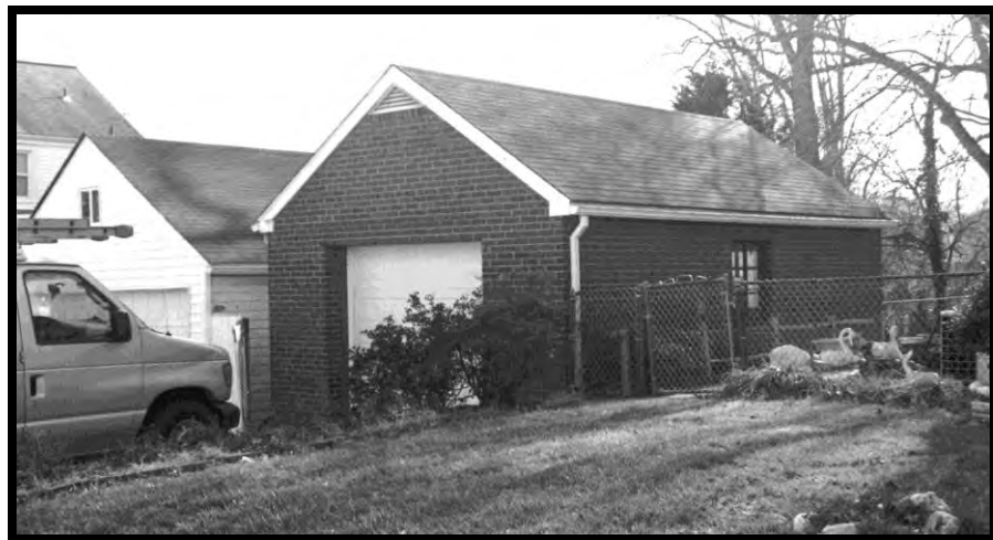
Figure 20: Garage, 700 South Wakefield Street, 000-4229-0388 (EHT Tracerics, 2012)
