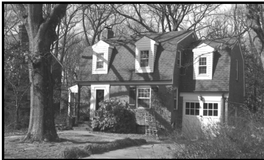
Figure 6: Single Dwelling, 304 South Abingdon Street, 000-7818-0211 (EHT Tracerics, 2012)
