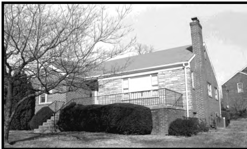
Figure 9: Single Dwelling, 1415 North George Mason Drive, 000-4229-0203 (EHT Tracerics, 2012)
