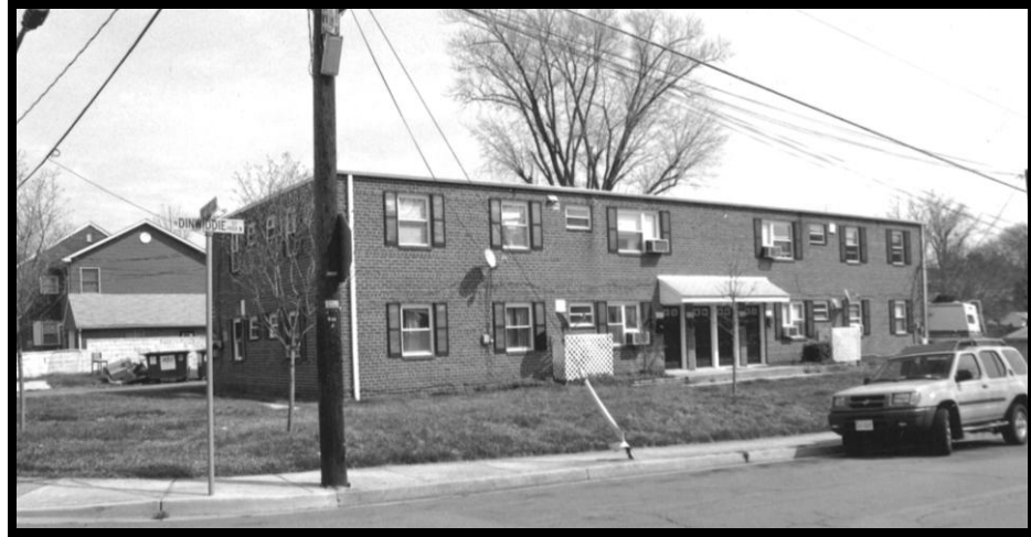
Figure 19: Multiple Dwelling, 4940-4946 19 th Street North, 000-4780 (EHT Tracerics, 2011)
