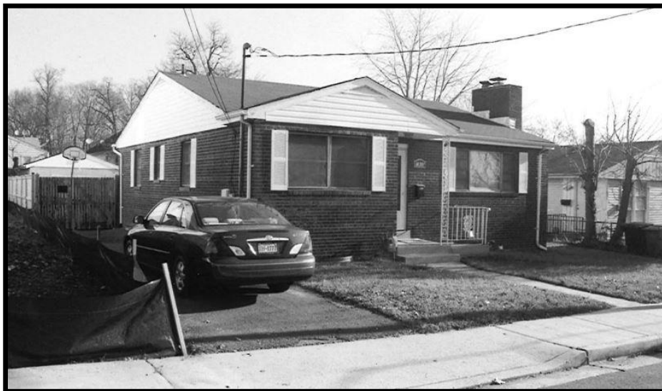
Figure 18: Single Dwelling, 1905 North Cameron Street, 000-4810 (EHT Tracerics, 2012)
