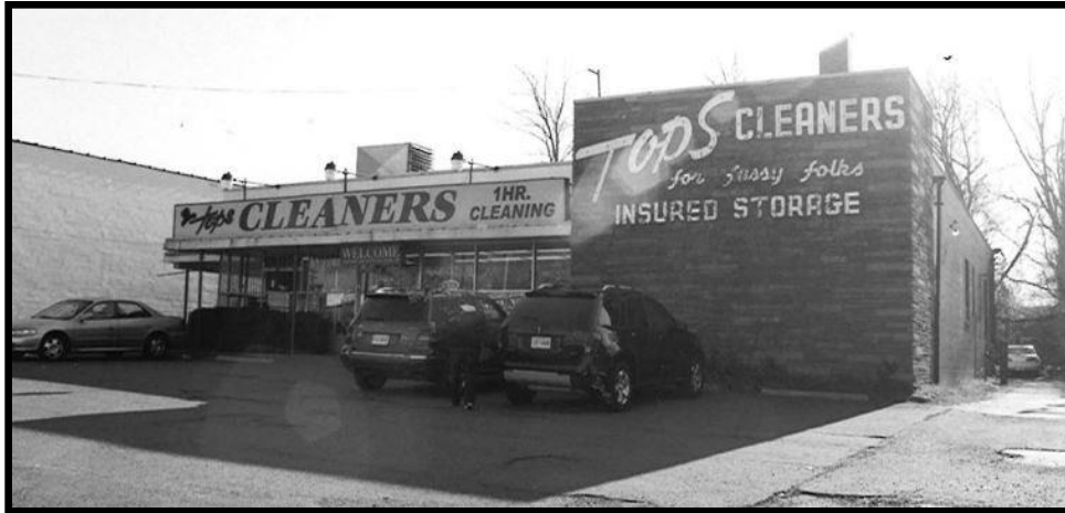
Figure 30: Commercial Building, 5210 Lee Highway, 000-4820 (EHT Tracerics, 2012)
