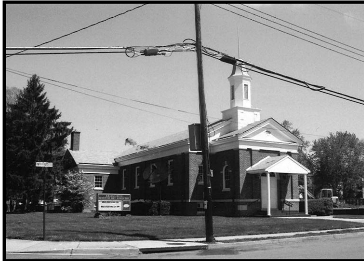
Figure 35: Church, 3425 9 th Street South, 000-4867-0178 (EHT Tracerics, 2012)
