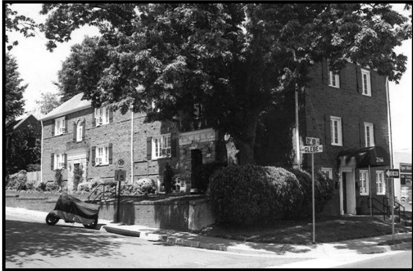
Figure 27: Apartment Building, 4751-4753 21 st Road North, 000-4887 (EHT Tracerics, 2013)
