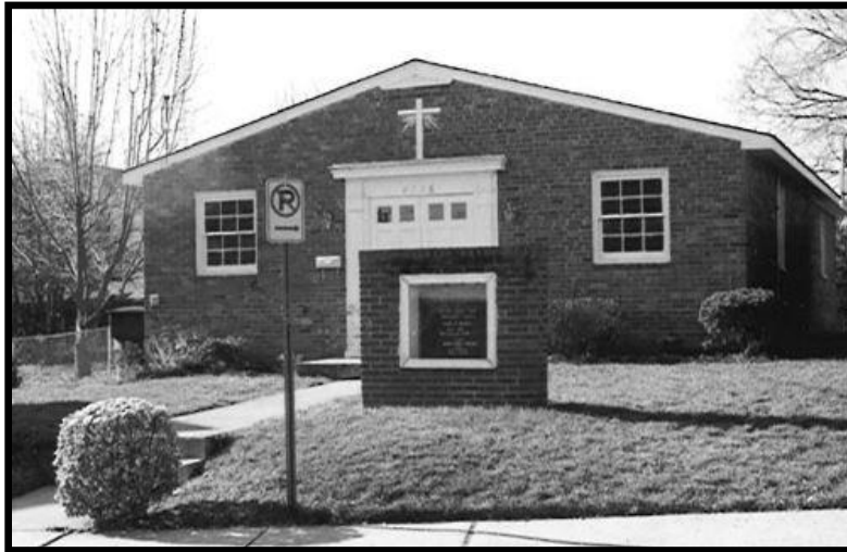
Figure 34: Church, 2118 North Cameron Street, 000-4809 (EHT Tracerics, 2012)
