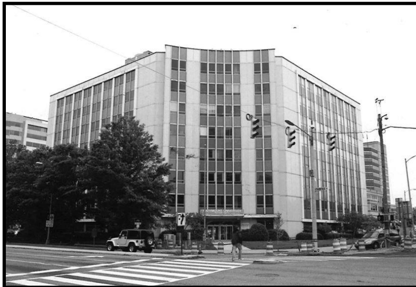
Figure 33: Office Building, 1000 North Glebe Road, 000-4892 (EHT Tracerics, 2013)
