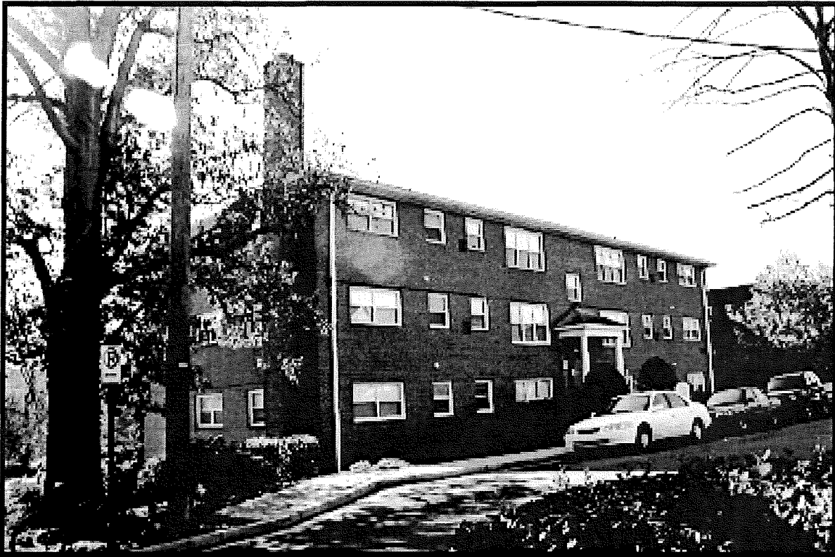
Figure 27: The Taylor, 1660-1670 21 st Road North, 000-4699 (EHT Tracerics, 2011)
