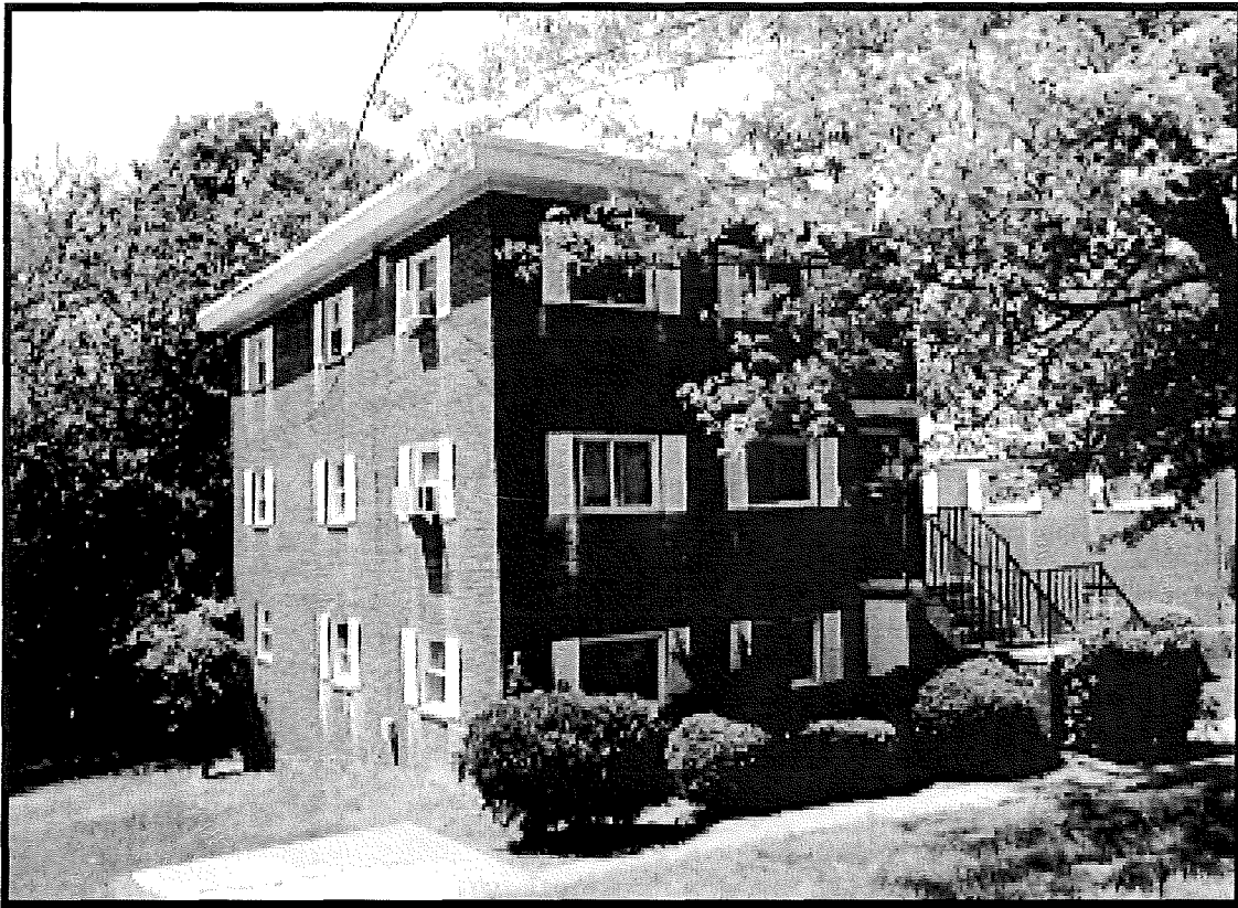
Figure 28: Multiple Dwelling, 1321 South Rolfe Street, 000-4693 (EHT Tracerics, 2011)
