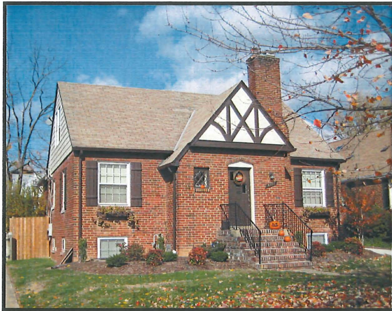
Single Dwelling, 4721 16 th Road North, 000-4229-0003 (EHT Traceries, 2011)
