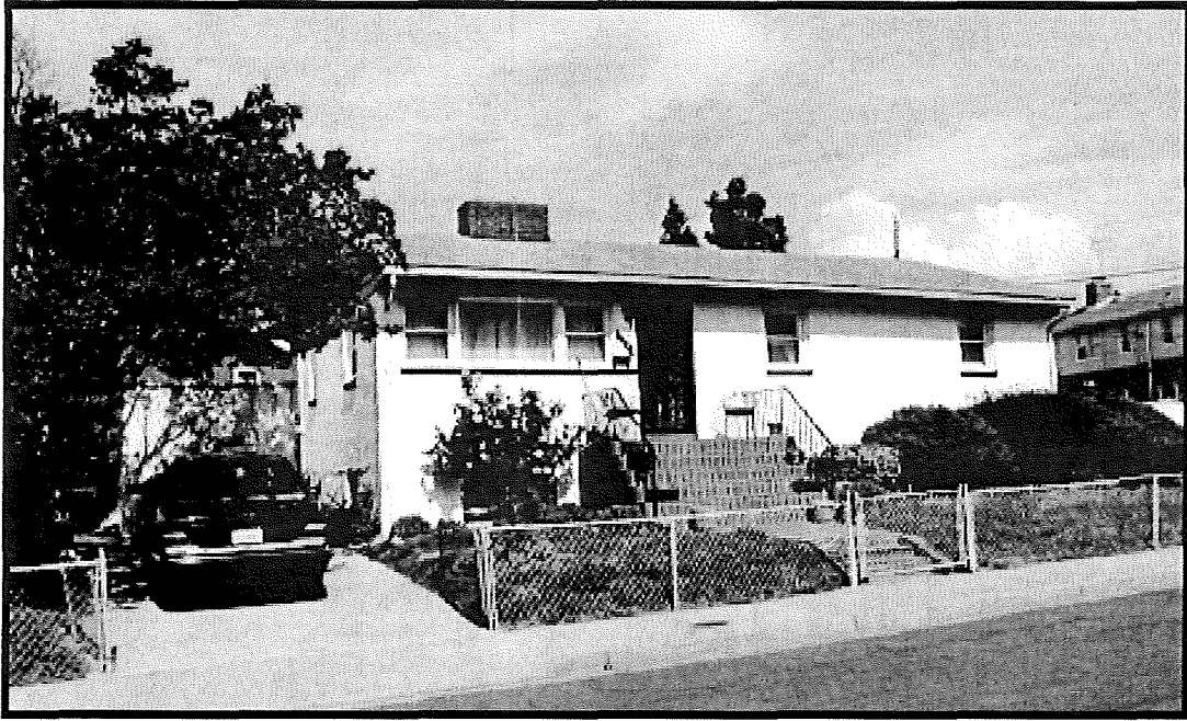
Figure 13: Single Dwelling, 1201 South Rolfe Street, 000-4685 (EHT Tracerics, 2011)
