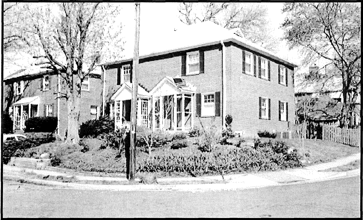
Figure 23: Twin Dwelling, 2003-2005 20 th Road North, 000-0433 (EHT Tracerics, 2011)
