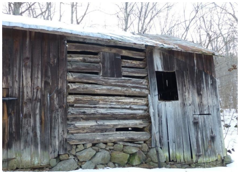
Figure 15. The nineteenth-century log core of the barn on the Elliott Farm (009-5272).
