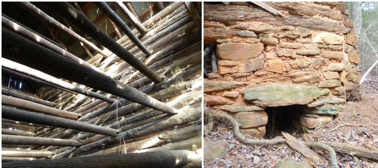
Figure 34. Tier poles inside a tobacco barn on the Martin Farm (009-5359).
