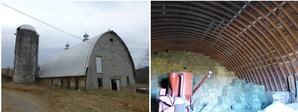
Figure 10. The Gothic Arch roof of the dairy barn on the Parkdale Farm (009-5107).
