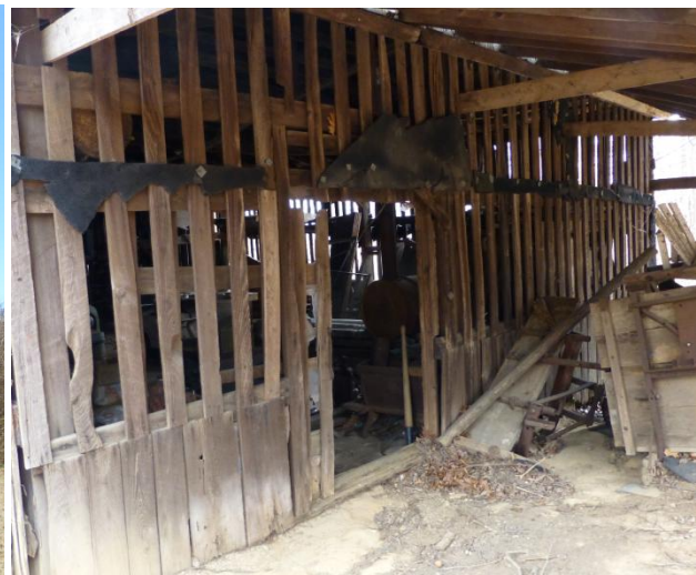
Figure 37. The slatted wall of the tomato cannery on the Arrington-Gross Farm (009-5112).
