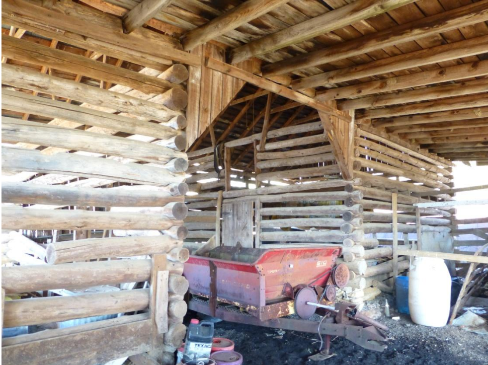
Figure 16. The double-crib log barn on the Key-Shackford Farm (009-5377).
