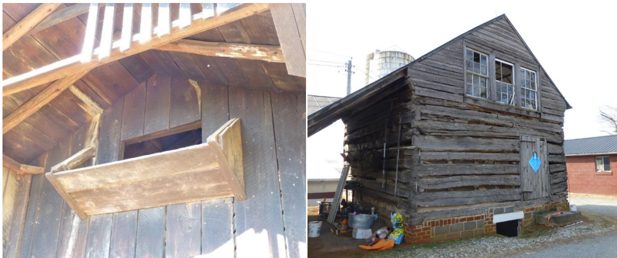
Figure 28. The hopper in the gable of the corncrib on the Anderson Farm (009-5399).
