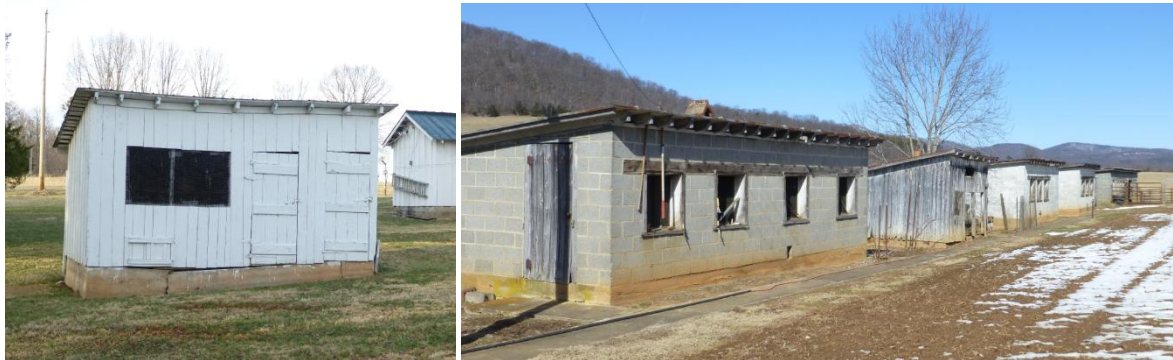
Figure 31. A frame chicken house of standard shed-roofed form on the Updike Farm (009-5394). Figure 32. A row of chicken houses on the Markham Farm (009-5372).
