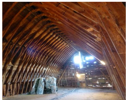
Figure 9. The self-supporting structure of the gambrel roof on the County Farm Barn (009-5031).
