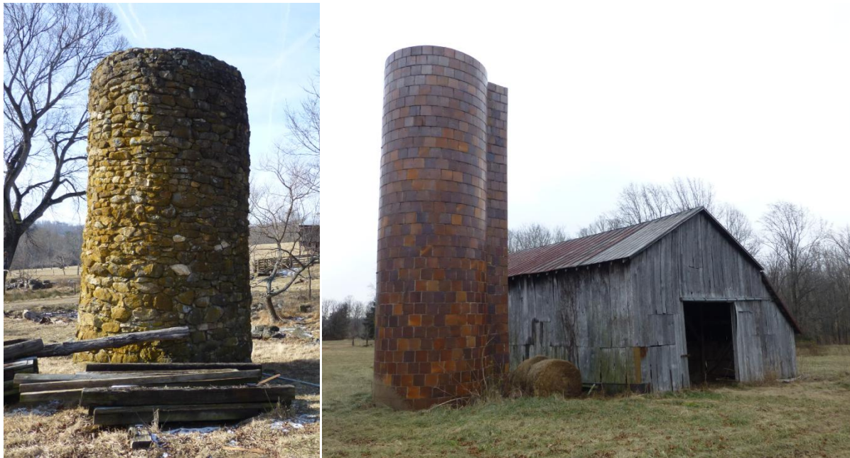
Figure 22. The stone silo on the Arrington Farm (009-5355).
