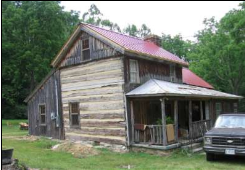
Figure 22: Munford Post Office (011-0123). The log constructed Munford Post Office (011-0123) with a ca. 1850 one-story section and a ca. 1873 two-story section.
