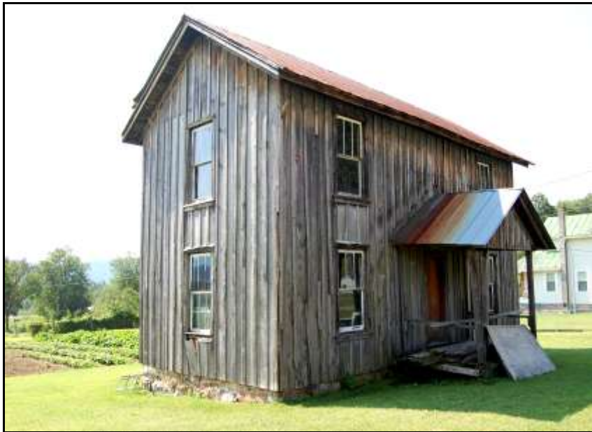
Figure 34: Worker's House, 8 Quarry Drive (Glen Wilton) (011-5357). The only intact example of several identical ca. 1890 houses built for Princess Iron Furnace workers in Glen Wilton. The other remaining workers' houses have been altered with vinyl siding, replacement windows, or additions.
