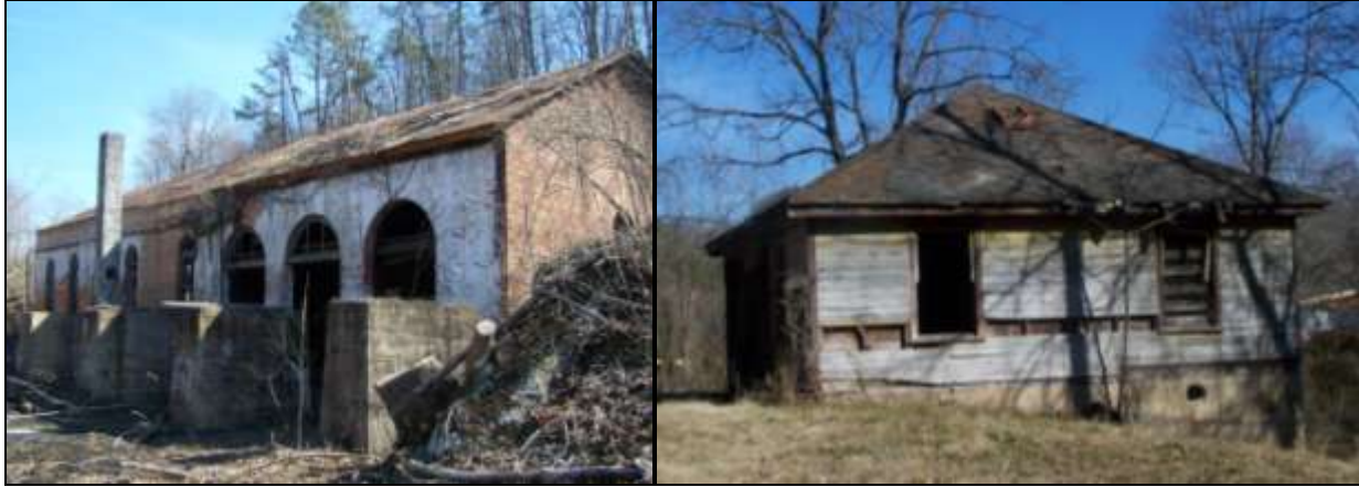
Figure 26: The Spec Mining Power Plant (011-5143) and its Company Housing (011-5197)
