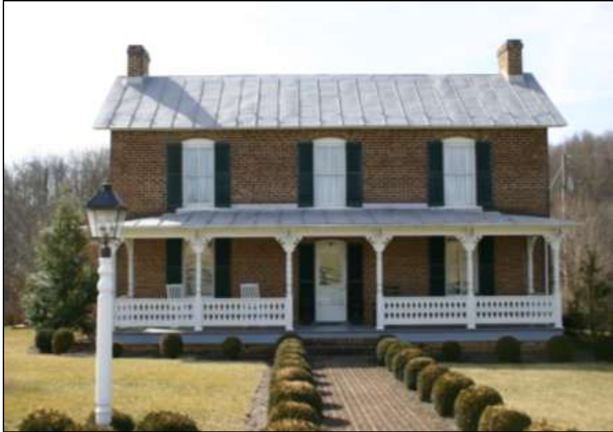
Figure 32: House, 1819 Wheatland Road (011-5177). This two-story, symmetrical three-bay brick house (011-5177) with interior-end brick chimneys is a good example of a more prosperous house-type built in Botetourt County ca. 1875.
