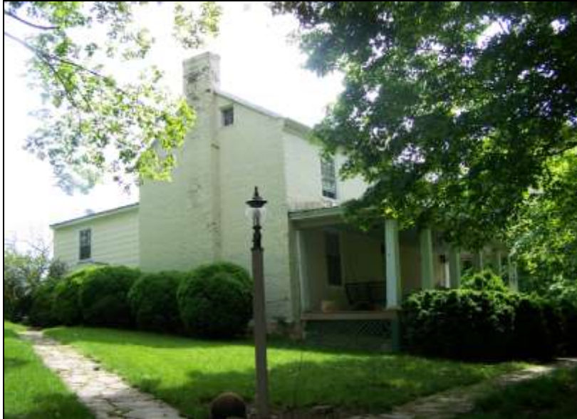
Figure 20: James Hogshead House (011-0059). The resurveyed, ca. 1846 James Hogshead House (011-0059) sits off the east side of Catawba Road on a five acre parcel near Tinker Creek. The two-story, symmetrical three-bay, single-pile brick dwelling features a Flemish bond façade and a hounds-tooth brick cornice. The original owner, James Hogshead, hired local contractor Samuel Rader to “build a kiln to produce 50,000 brick for a 36’x 20’ 2/2 central-hall house with 13” thick walls.” (Description based on the original contract).
