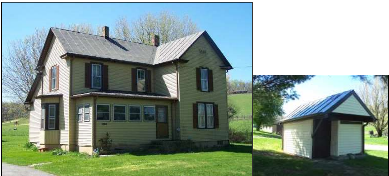
Figure 33: House, 5402 Roanoke Road (011-4257). A typical T-plan house common to Botetourt County for this time period is found in the house in the Trinity area off Roanoke Road/Route 220 (011-5257). Note the associated outbuilding, a possible springhouse.
