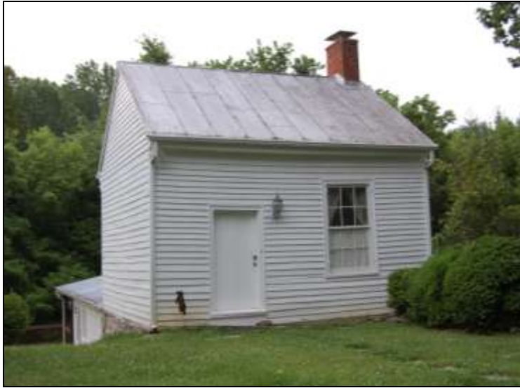
Figure 15: Houston School (outbuilding to 218-0051-0073). A good surviving example of a private one-room schoolhouse operated by a religious institution is located just south of the Presbyterian Parsonage House (218-0051-0073) in the Town of Fincastle. The ca. 1856 Houston School, which has a side-gabled standing seam metal roof, is clad in weatherboard siding, and rests upon a stone foundation.
