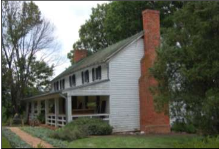
Figure 6: Rustic Lodge (011-0053). The previously surveyed ca. 1800 five-bay Rustic Lodge (011-0053) is a two-story, double-pen log house joined by a centered passage and clad with weatherboard siding. The house was once part of a large farm settled by the prosperous Burwell family that moved from Tidewater Virginia.
