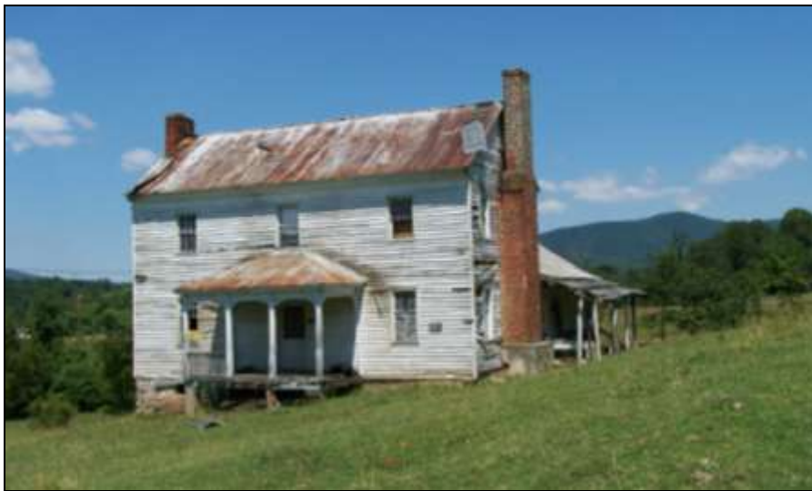
Figure 19: I-House (011-5333). This early ca. 1830-1850 I-house (011-5333) in the Blue Ridge community features a three-bay center-passage, single-pile plan on a limestone foundation. An exterior-end Flemish bond brick chimney heated the residence. Brick nogging is exposed in the right-side gable end.
