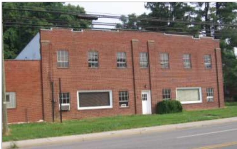
Figure 38: The ca. 1940 Troutville Poultry Plant (315-5021) located on Route 11 in Troutville
