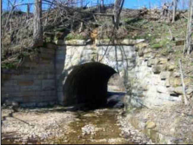
Figure 24: Norfolk & Western railroad underpass (011-5201), constructed ca. 1910 of coursed ashlar.
