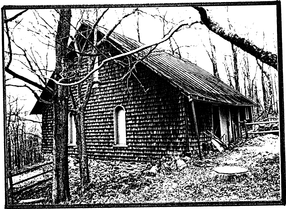
Fig. 5 Barn at House off of Rt. 601N (21-927) (J.Perkins)
