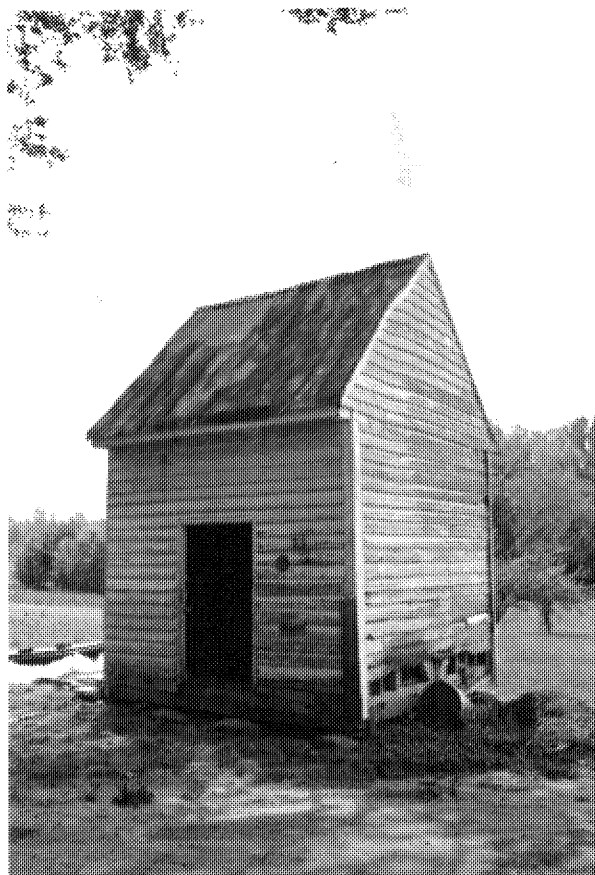
Figure 47: Photograph of Icehouse at Millview (24-114)
