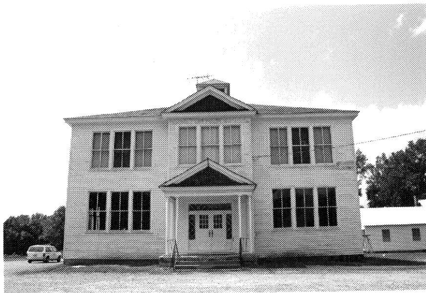
Figure 107: Photograph of Hamilton High School (24-105)
