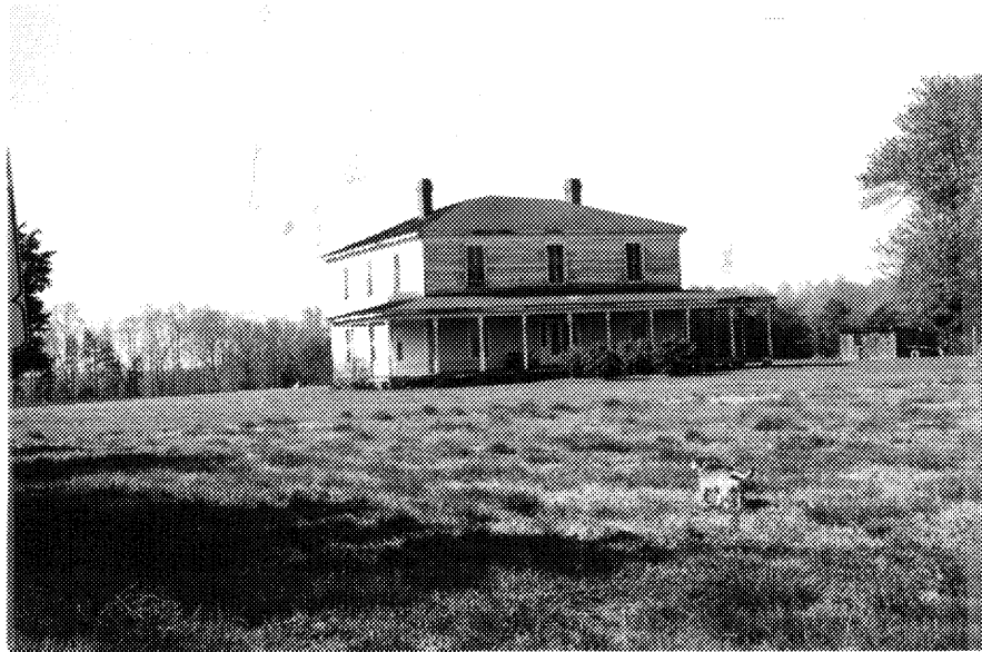
Figure 62: Photograph of Sunny Side Post Office (24-211)
