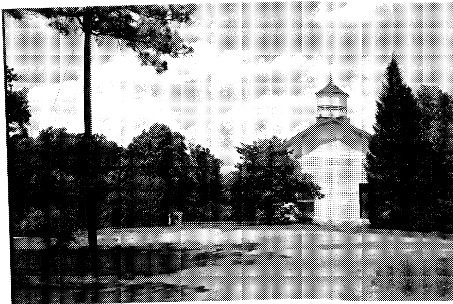
Figure 86: Photograph of Methodist-Episcopal Church South (24-126-13)
