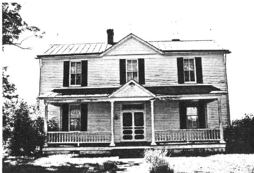
Figure 28: Photograph of High Bridge Farm (24-311)
