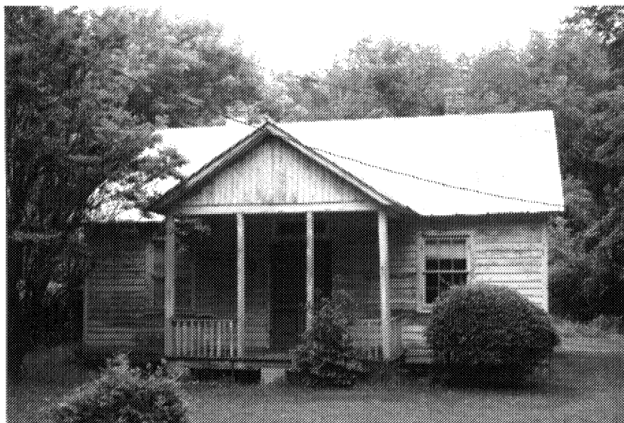
Figure 103: Photograph of Millworker's Residence (24-357)
