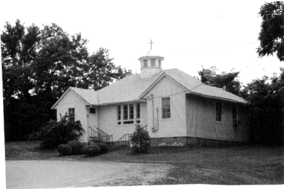
Figure 85: Photograph of Saint Catherine's Catholic Church (24-126-21)
