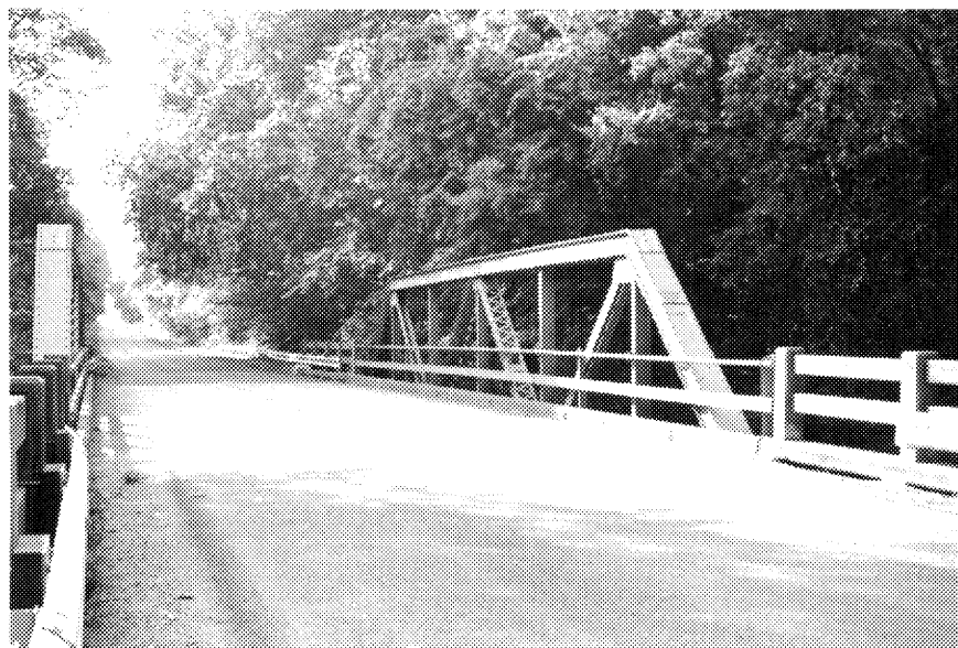
Figure 111: Photograph of Willis River Bridge (24-71)
