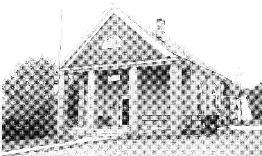
Figure 63: Photograph of Cartersville Post Office (24-126-32)
