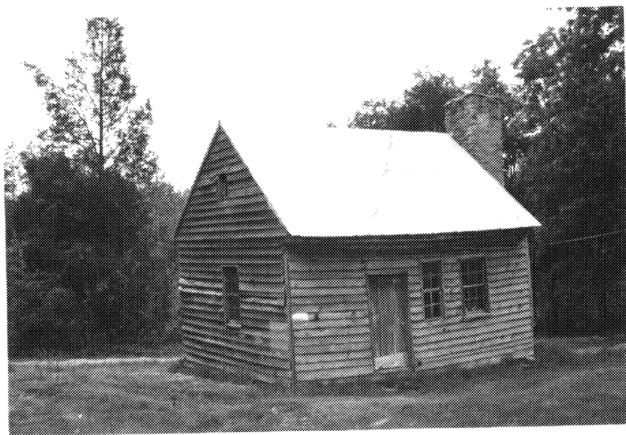
Figure 40: Photograph of Kitchen at Locust Grove (24-104)
