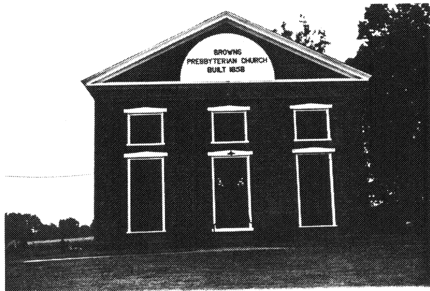
Figure 76: Photograph of Brown's Presbyterian Church (24-2)
