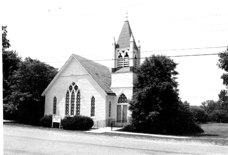
Figure 84: Photograph of Cartersville Baptist Church (24-126-20)
