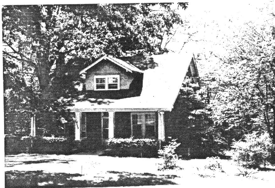
Figure 33: Photograph of House on Osborn Road (24-406)
