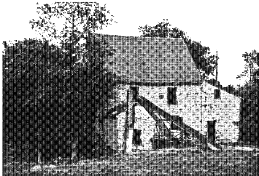
Figure 102: Photograph of Trent's Mill (24-50)
