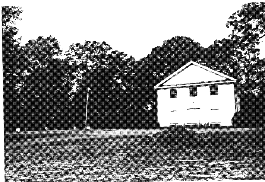
Figure 80: Photograph of Fork of Willis Church (24-6)
