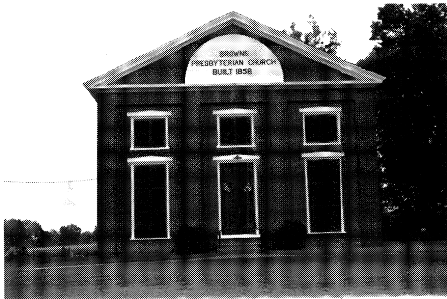
Figure 76: Photograph of Brown's Presbyterian Church (24-2)
