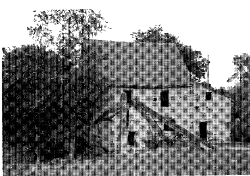
Figure 102: Photograph of Trent's Mill (24-50)
