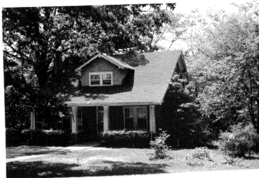
Figure 33: Photograph of House on Osborn Road (24-406)
