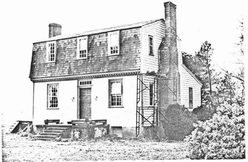
The Sanderson/Hathaway house on Battlefield Boulevard near the North Carolina Line, showing gambrel roof with steep lower slope and nearly flat upper slope.
