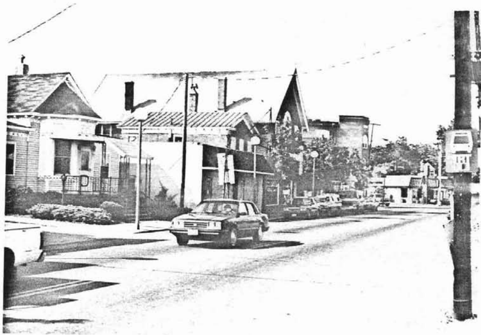
The commercial section of Poindexter Street in the South Norfolk Historic District
