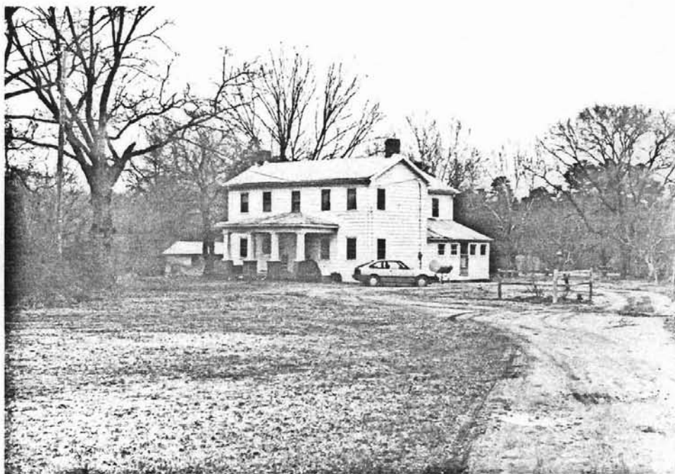
457 Great Bridge Road, farmhouse that was once a part of the Upton Farm which previously belonged to the Williamson family who owned many acres on both sides of the road.
