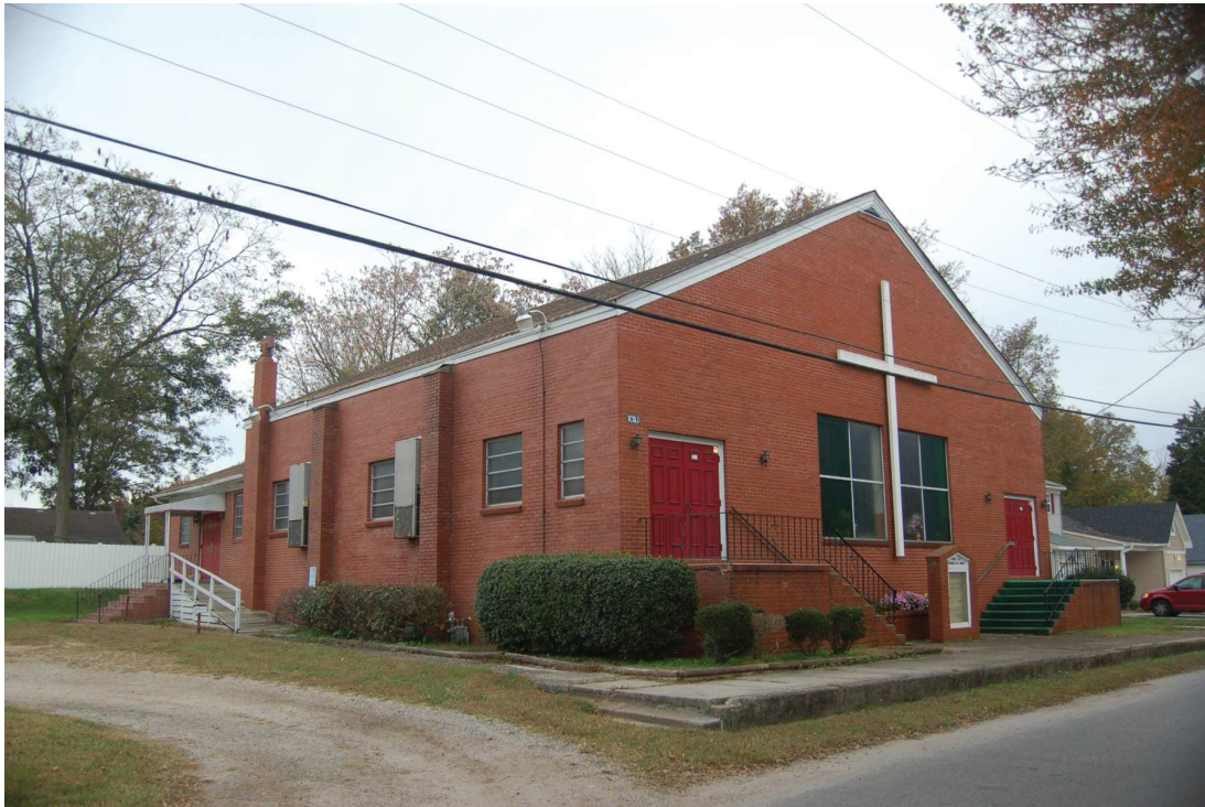
Figure 41. Strait Gate Evangelistic Church (131-5402), north and east elevations.
