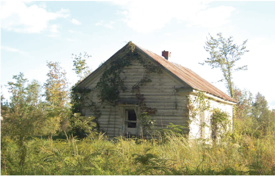
Figure 15. Cornland School (131-0111), north and west elevations.
