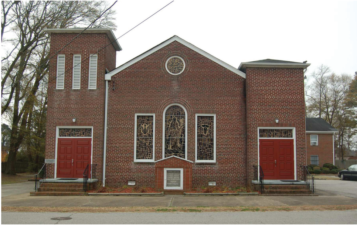
Figure 43. Divine Baptist Church (131-5397), north elevation.
