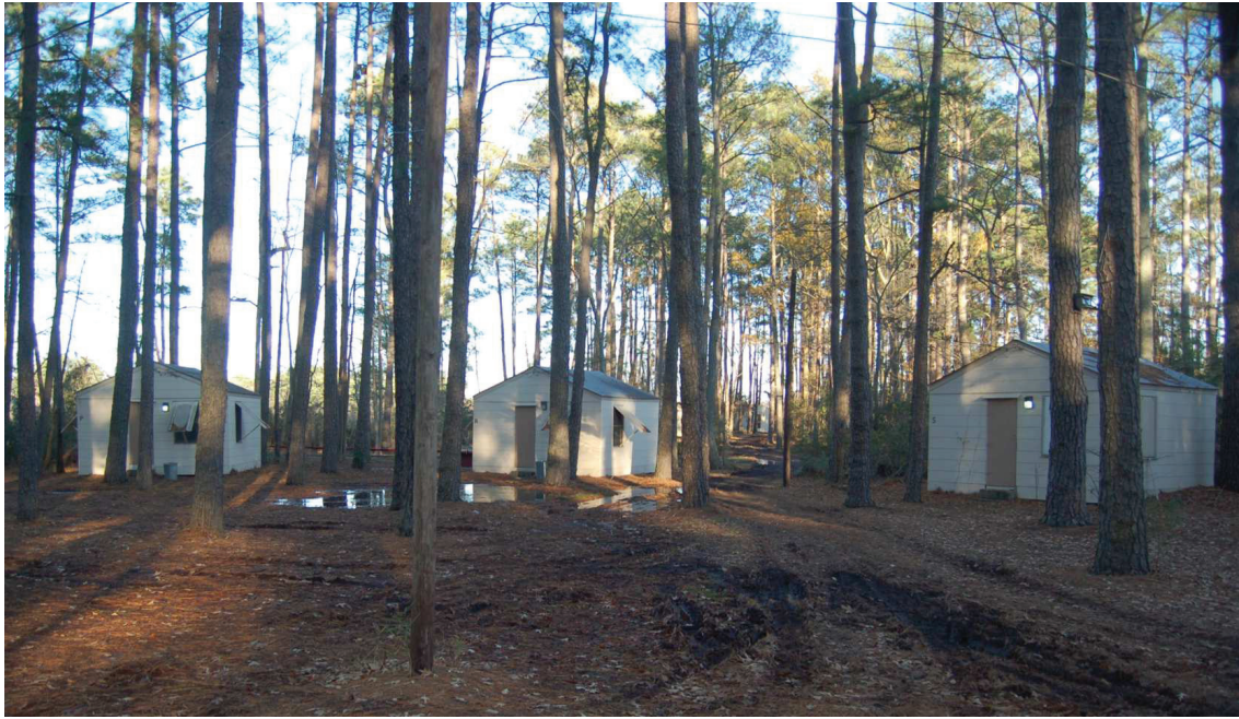
Figure 32. Camp E. W. Young (131-5388), cabins P, R, and S, looking northeast.
