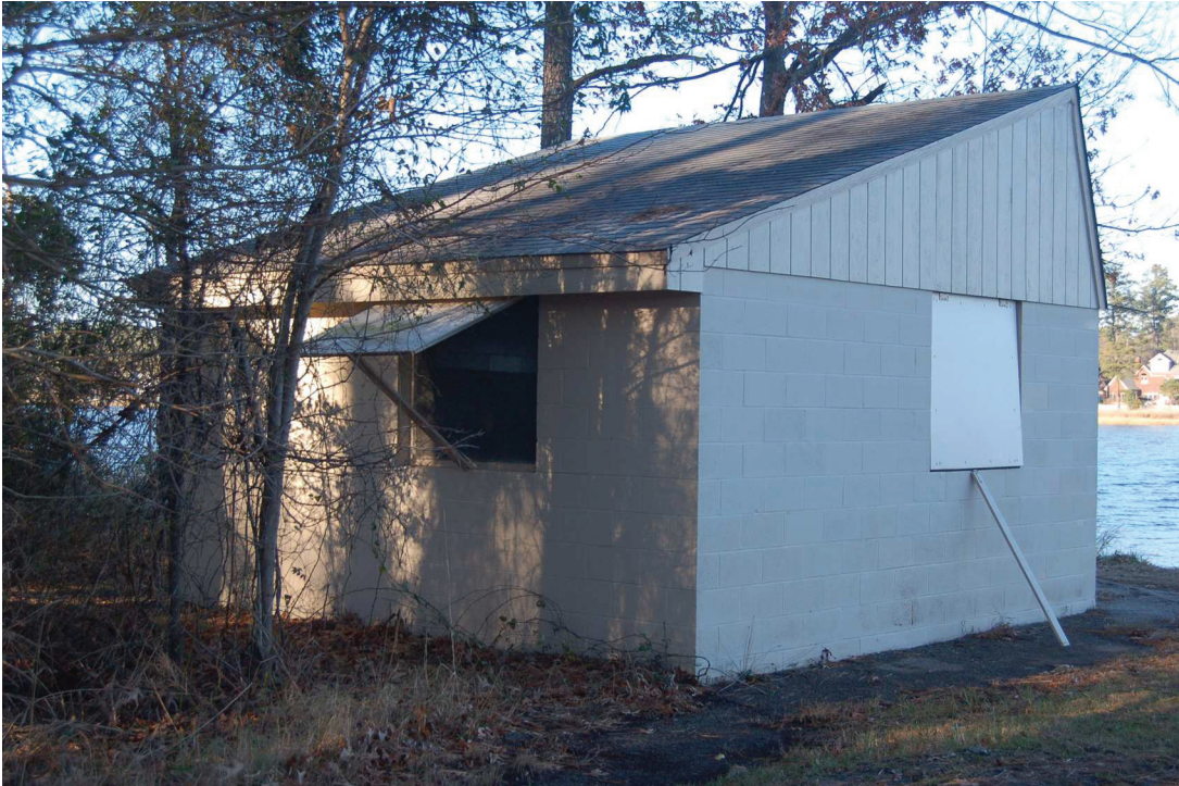
Figure 34. Camp E. W. Young (131-5388), cabin EE, south and west elevations.
