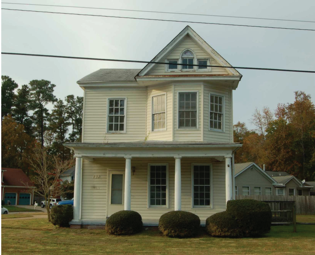
Figure 7. Dr. Hugo Owens, Sr. House (131-0501), south elevation.
