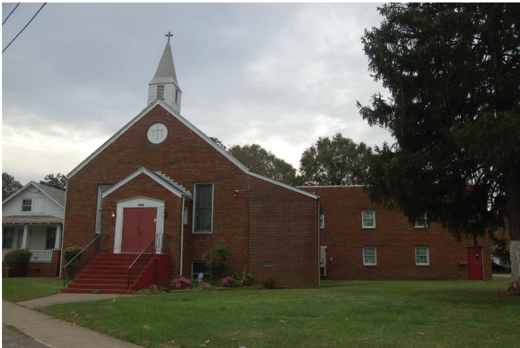
Figure 40. Mount Zion Baptist Church (131-5399), north and east elevations.
