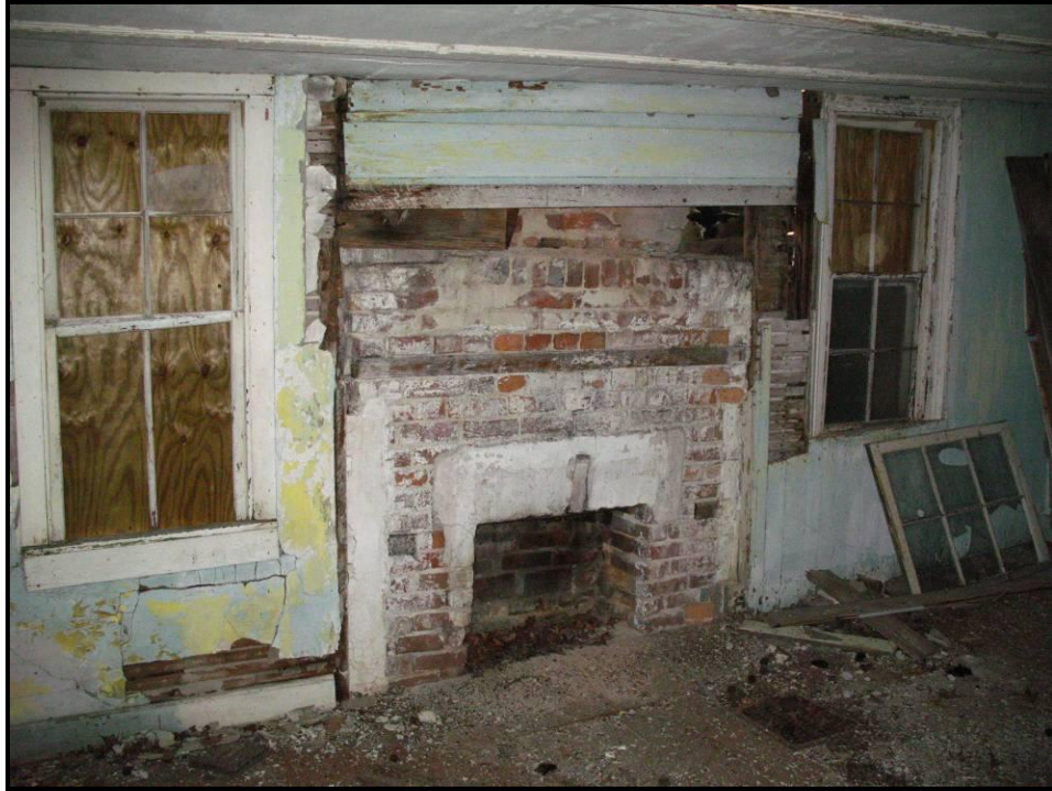
Figure 160. Second Floor Fireplace Wall, View Looking Southwest.
