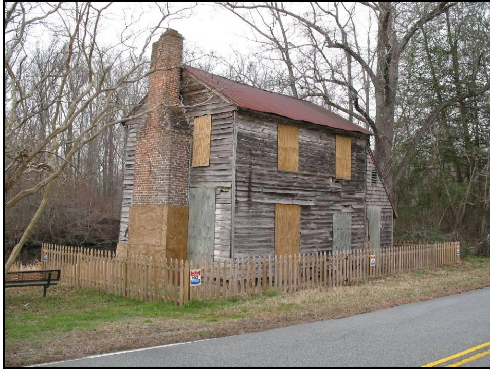
Figure 158. Superintendent's House (VDHR #131-0380), Dismal Swamp Canal Trail, View Looking North.
