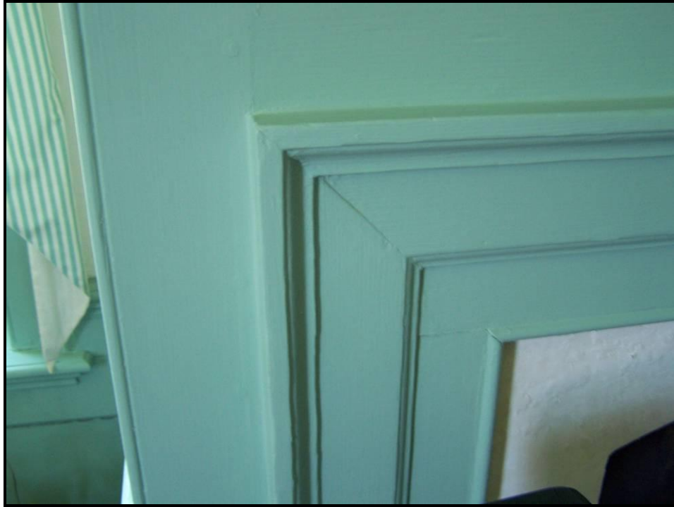
Figure 94. Detail of Fireplace Surround Molding in Dining Room, View Looking Southwest.
