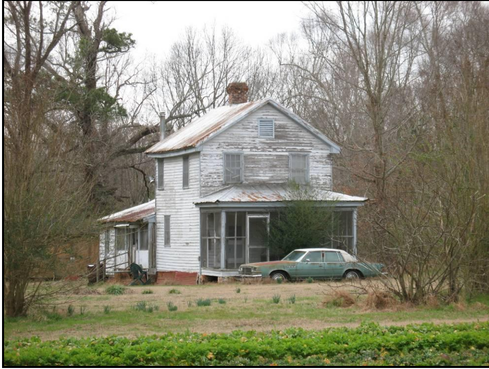
Figure 25. Example of Two-Story Front Gable Dwelling (VDHR #131-0091), 435 Gallbush Road, View Looking Southwest.
