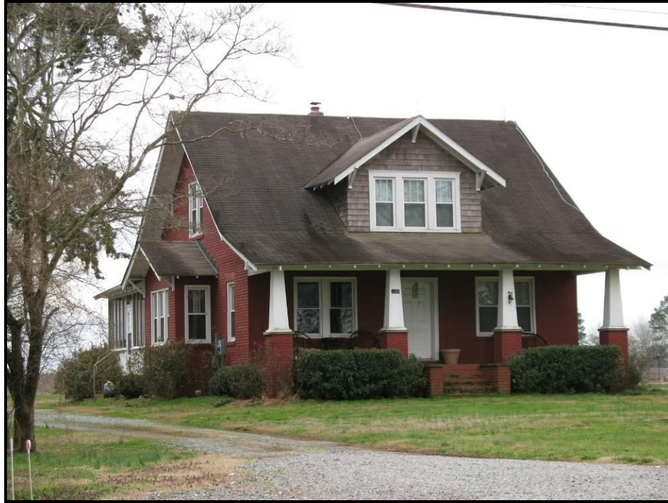
Figure 13. Craftsman-Style Bungalow (VDHR #131-5435), 2201 Mt. Pleasant Road, View Looking Southwest.
