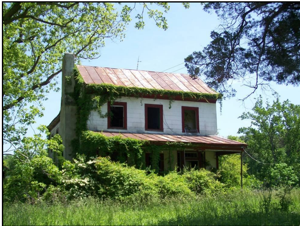
Figure 109. Etheridge House (VDHR #131-0089), 635 John Etheridge Road, View Looking Northeast.
