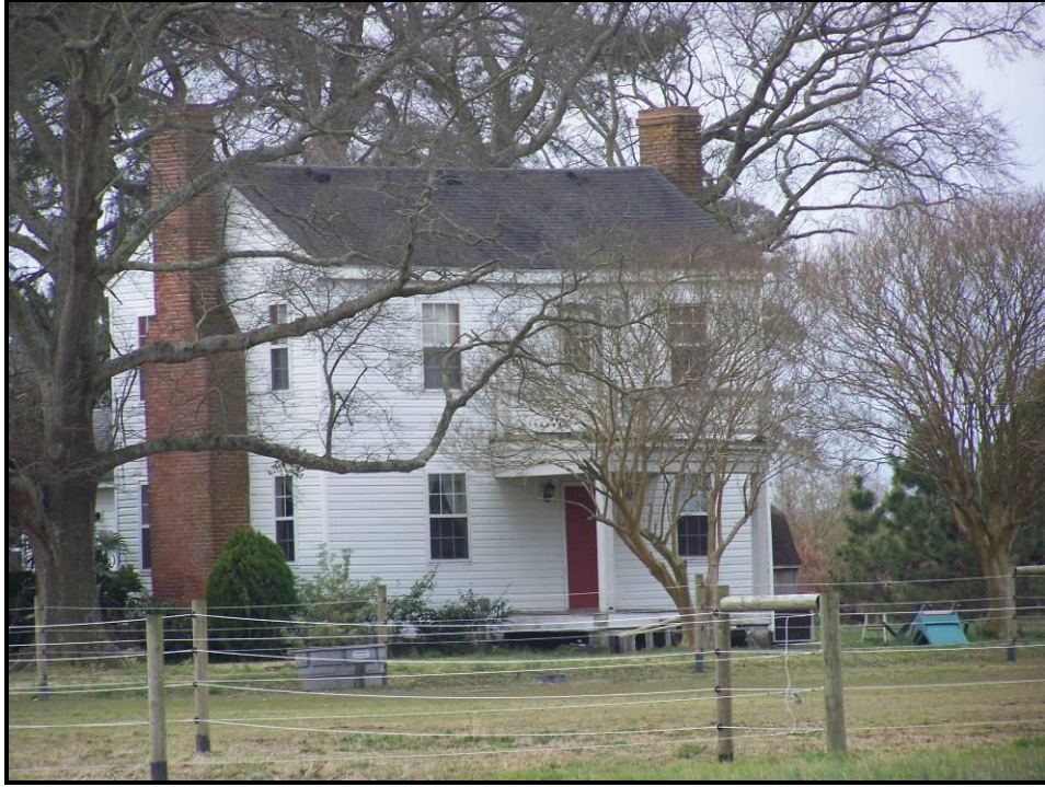
Figure 41. Example of Two-Story Center Hall Plan Dwelling (VDHR #131-0188), 620 Carter Road, View Looking Southwest.
