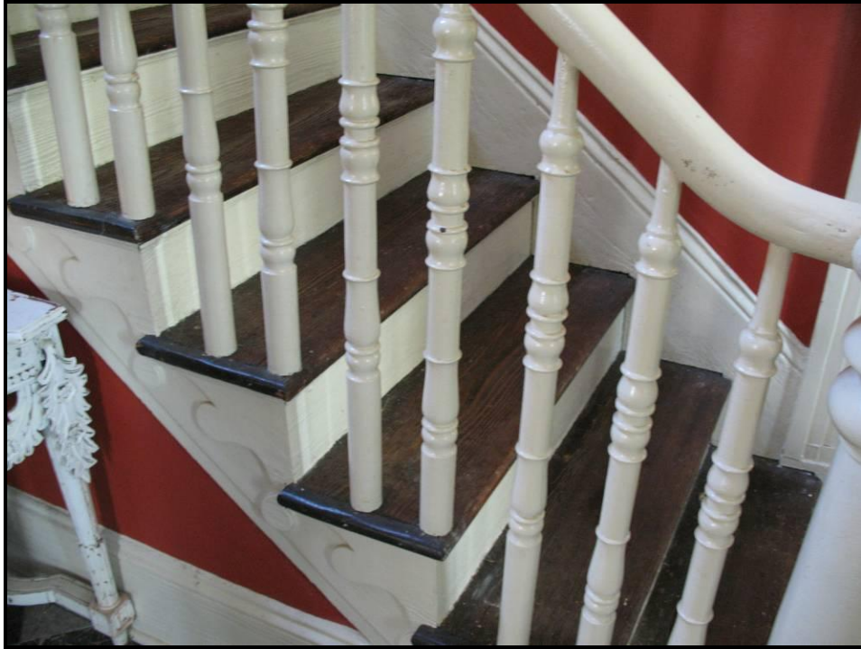
Figure 138. Detail of First Floor Hallway Staircase, View Looking North.
