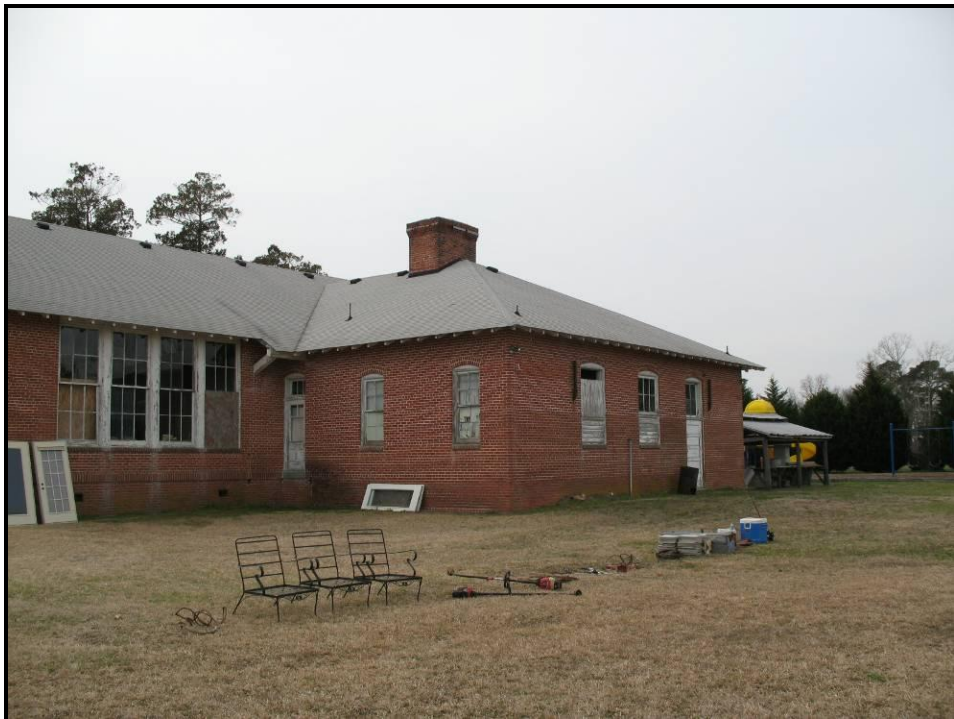
Figure 101. Gertie School (VDHR #131-0068), 4032 Bunch Walnuts Road, View Looking West.
