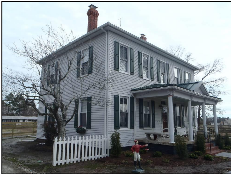
Figure 44. Example of Two-Story, Five-Bay Center Hall Plan Dwelling (VDHR #131-0143), 1004 Head of River Road, View Looking Northeast.
