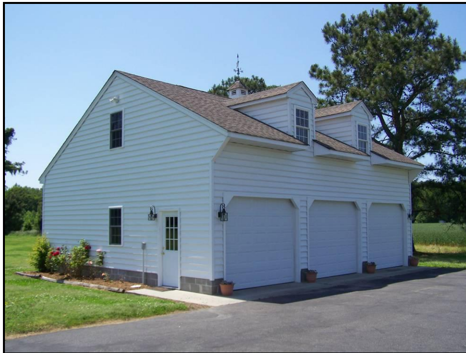
Figure 90. Garage, View Looking Northwest.
