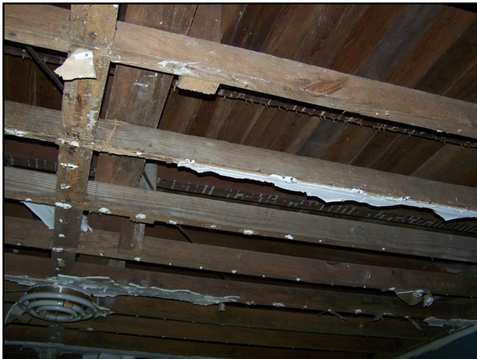
Figure 114. Detail of Ceiling in Kitchen, View Looking Southeast.
