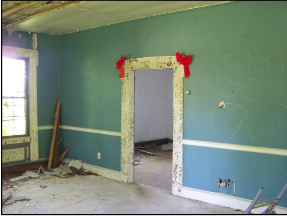
Figure 111. First Floor Room of Main Block, View Looking North.
