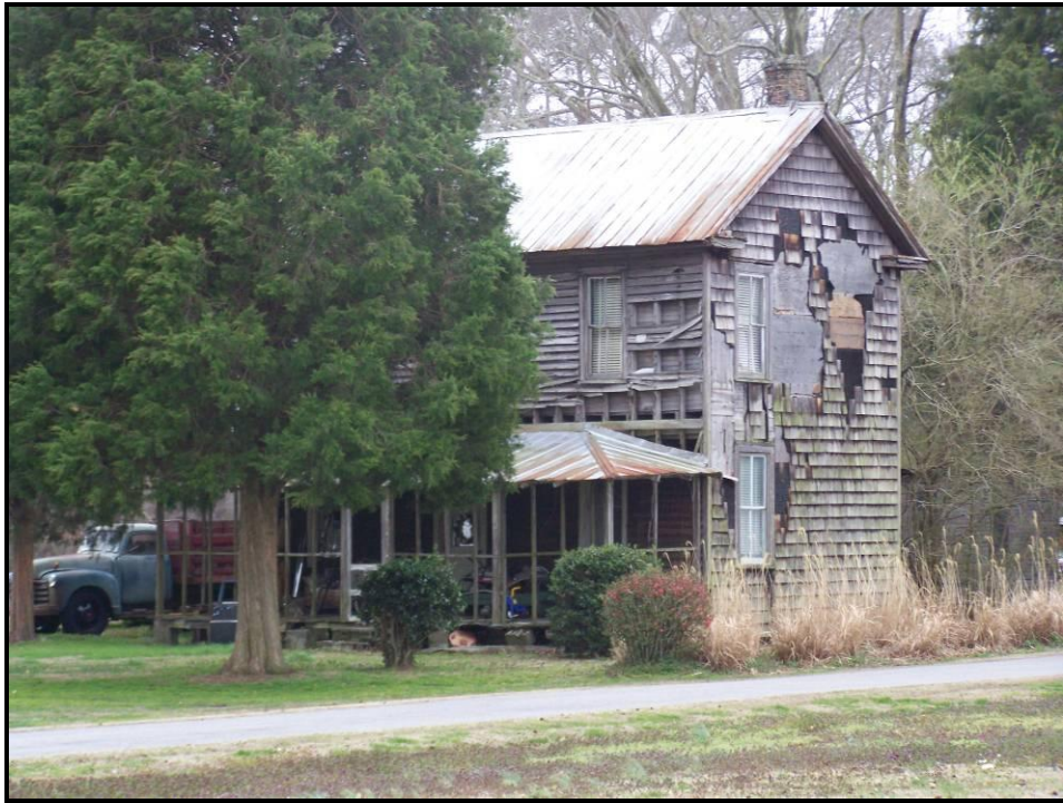
Figure 42. Example of Two-Story Center Hall Plan Dwelling (VDHR #131-0192), 1645 Blue Ridge Road, View Looking Southwest.
