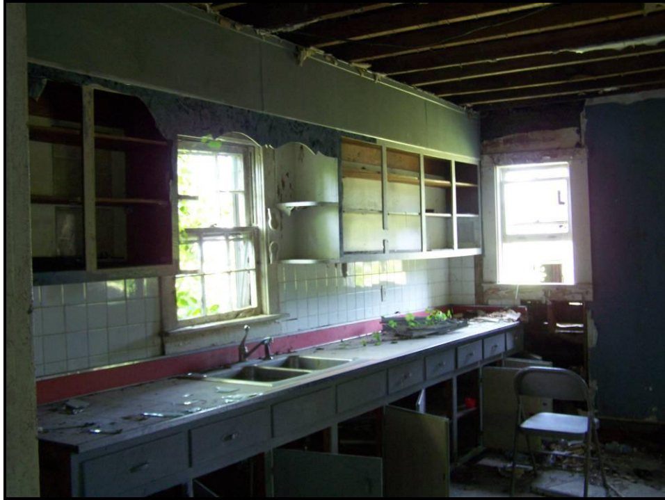
Figure 113. Kitchen in Ell, View Looking Northeast.
