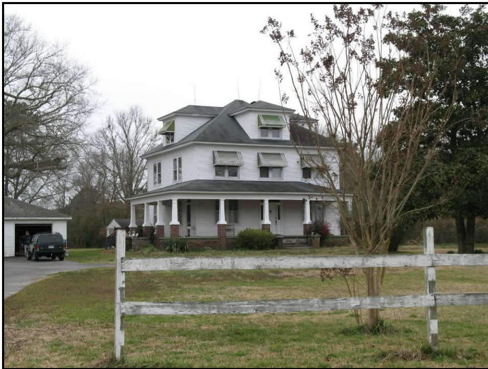
Figure 38. Example of American Four-Square (VDHR #131-0315), 4504 Old Battlefield Blvd, View Looking Southwest.
