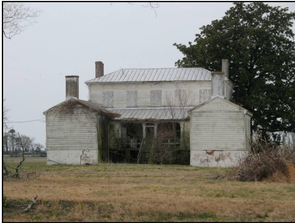
Figure 86. Beechwood (VDHR #131-0008), 3728 Belle Haven Road, View Looking West.
