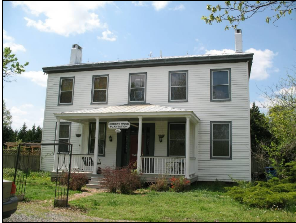
Figure 132. Ives-Wilson House (VDHR #131-0226), 2410 Centerville Turnpike, View Looking West.
