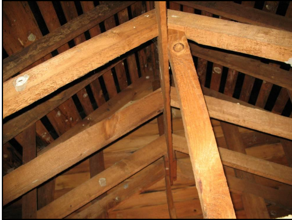
Figure 123. Detail of Attic Framing of Original 1871 Church (VDHR #131-0107), View Looking West.
