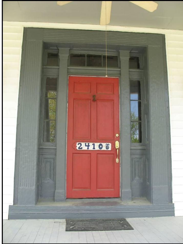
Figure 134. Front Entry Detail of the Ives-Wilson House (VDHR #131-0226), 2410 Centerville Turnpike, View Looking West.
