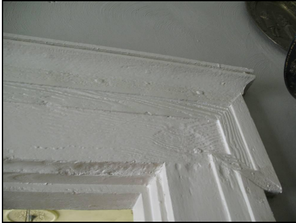
Figure 143. Detail of Dining Room Door Surround, View Looking Northwest.
