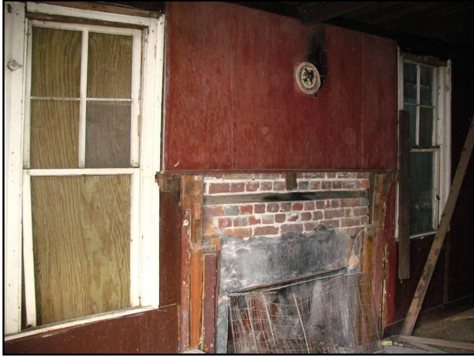
Figure 159. First Floor Fireplace Wall, View Looking Southwest.
