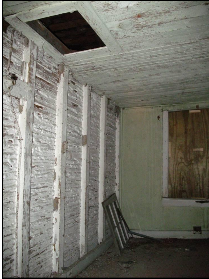
Figure 161. Second Floor Hallway, View Looking West.
