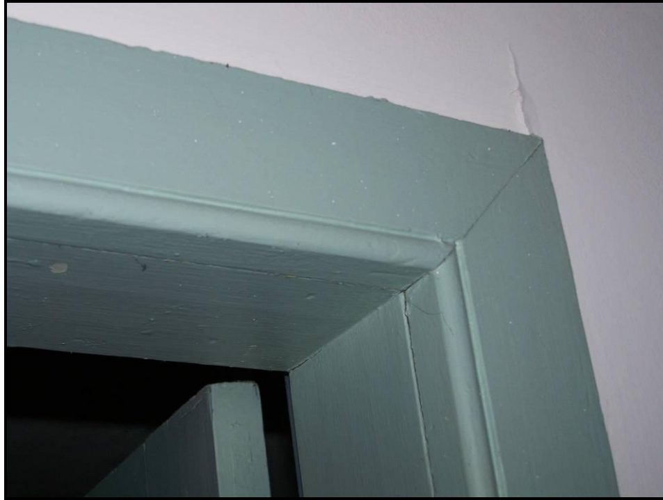
Figure 98. Detail of Beaded Door Surround, Second Floor Hallway, View Looking Southeast.
