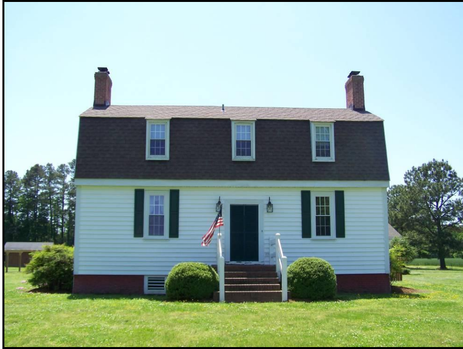
Figure 24. Holstead-Butts House (VDHR #131-0034), 1200 Taft Road, View Looking Southwest.
