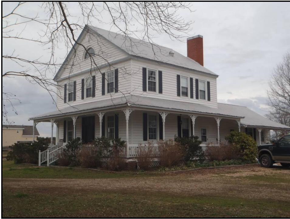
Figure 26. Example of Two-Story Front Gable Dwelling (VDHR #131-0084), 1902 Indian Creek Road, View Looking Northwest.
