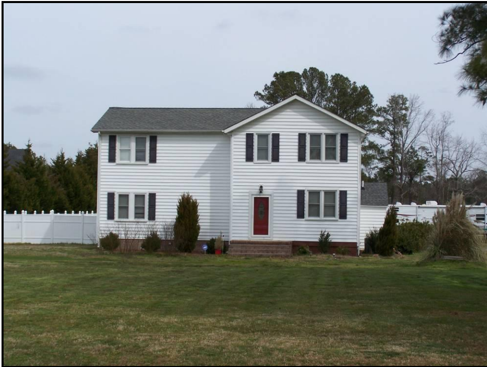
Figure 28. Example of Two-Story Front Gable Dwelling (Heavily Altered; VDHR #131-0128), 1201 Taft Road, View Looking Northeast.
