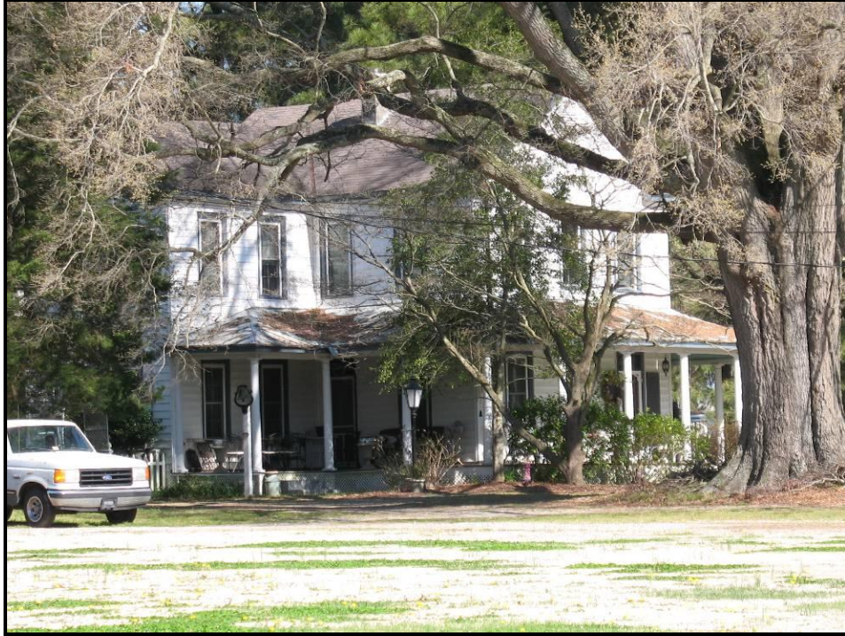
Figure 129. Riddick House (VDHR #131-0225), 2328 Centerville Turnpike, View Looking North.
