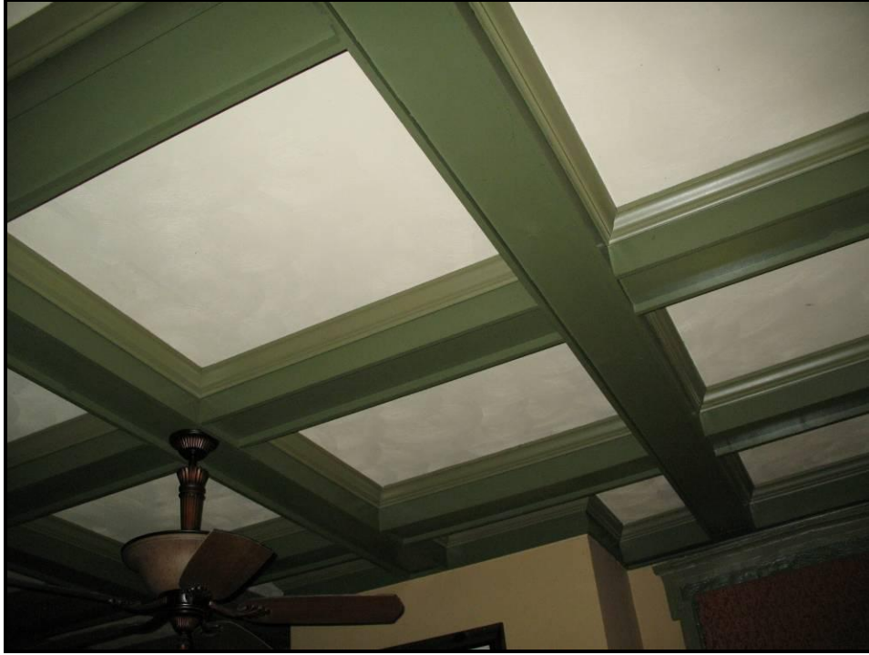
Figure 136. "Boxed Beams" added to Parlor Ceiling, View Looking North.
