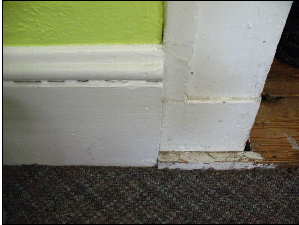
Figure 152. Detail of Baseboard in Ell, View Looking Northwest.
