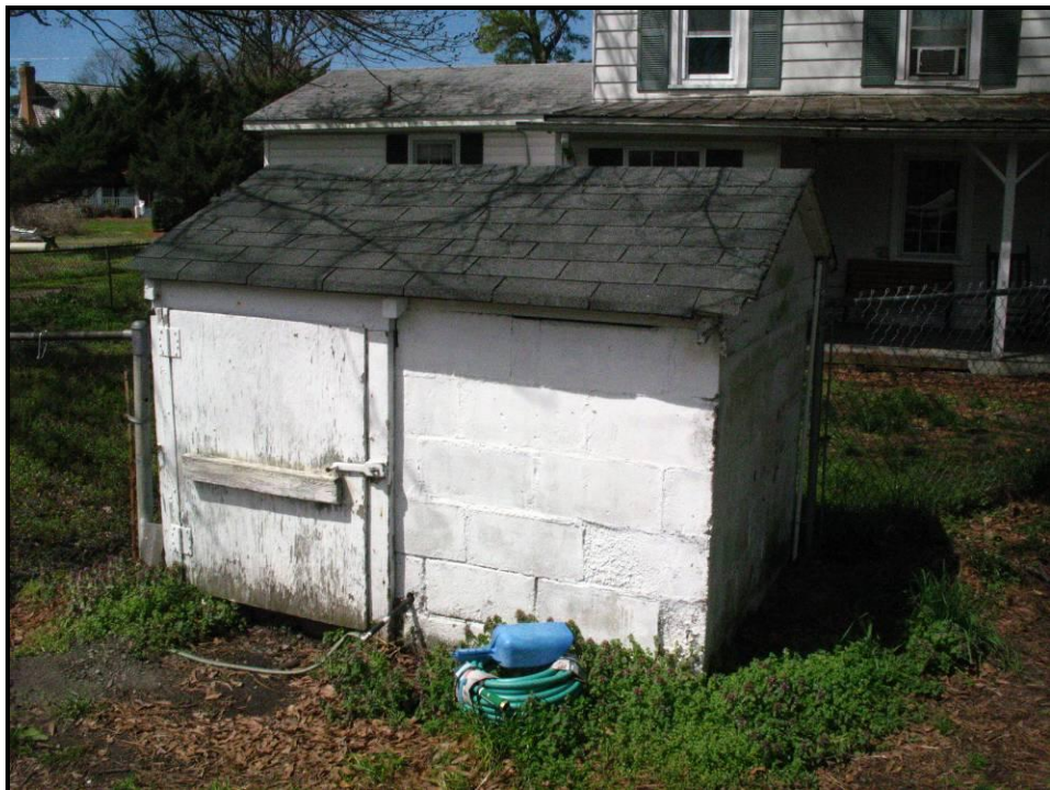
Figure 156. Pump House (VDHR #131-0234), 2261 West Road, View Looking West.
