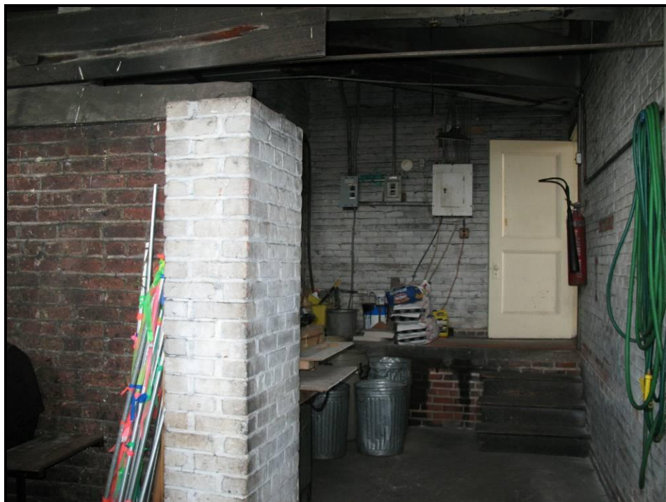
Figure 107. Boiler Room (VDHR #131-0068), View Looking Southwest.
