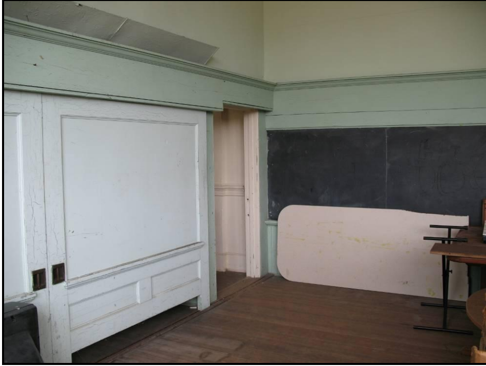
Figure 104. Southeast Classroom (VDHR #131-0068), View Looking North.
