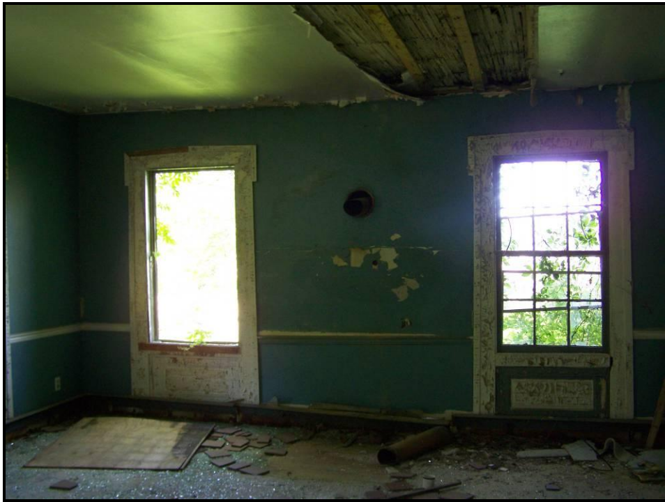
Figure 112. First Floor Room of Main Block, View Looking Northwest.
