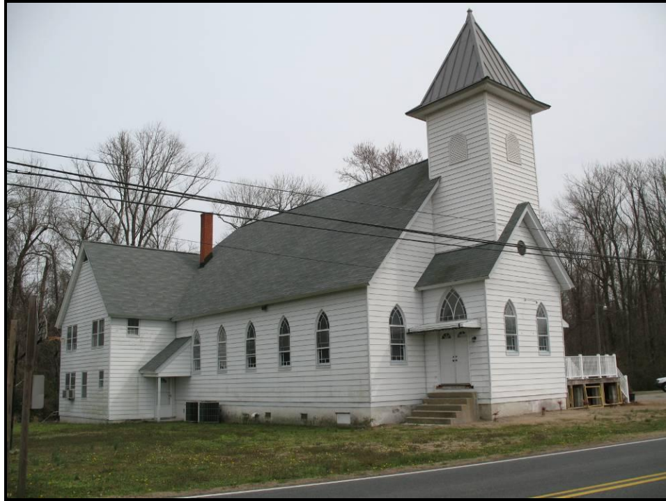
Figure 56. Northwest Baptist Church (VDHR #131-0051), 848 Ballahack Road, View Looking East.
