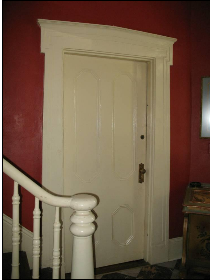
Figure 140. Door Surround on North Wall of Hallway, View Looking Northeast.
