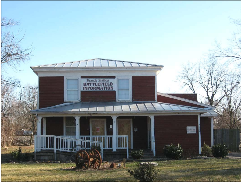
Photo 2: The Graffiti House (023-5092), Primary Elevation.
