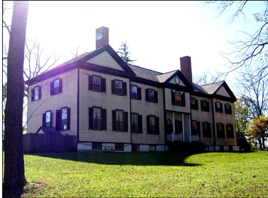
Photo 14: Farley (023-0005), Northeast Oblique.
