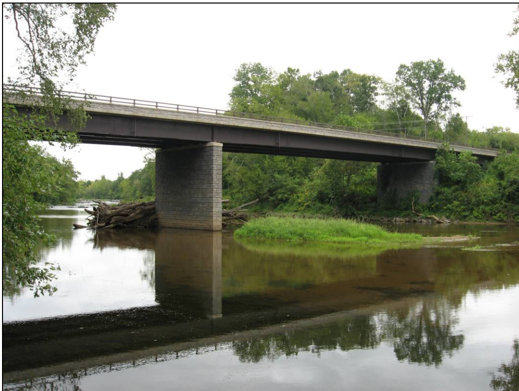
Photo 50: The New Circa 2003 Kelly's Ford Bridge, Looking Northeast.
