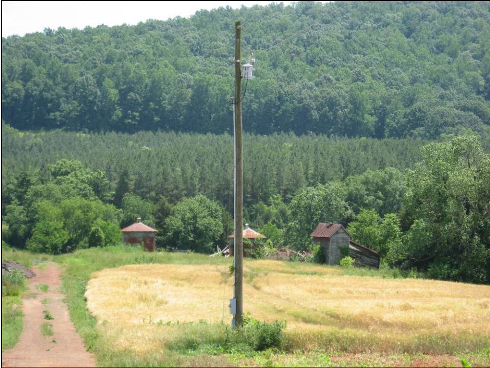
Photo 8: The Crittenden House Site (Foreground) Showing Remaining Outbuildings, Looking South.
