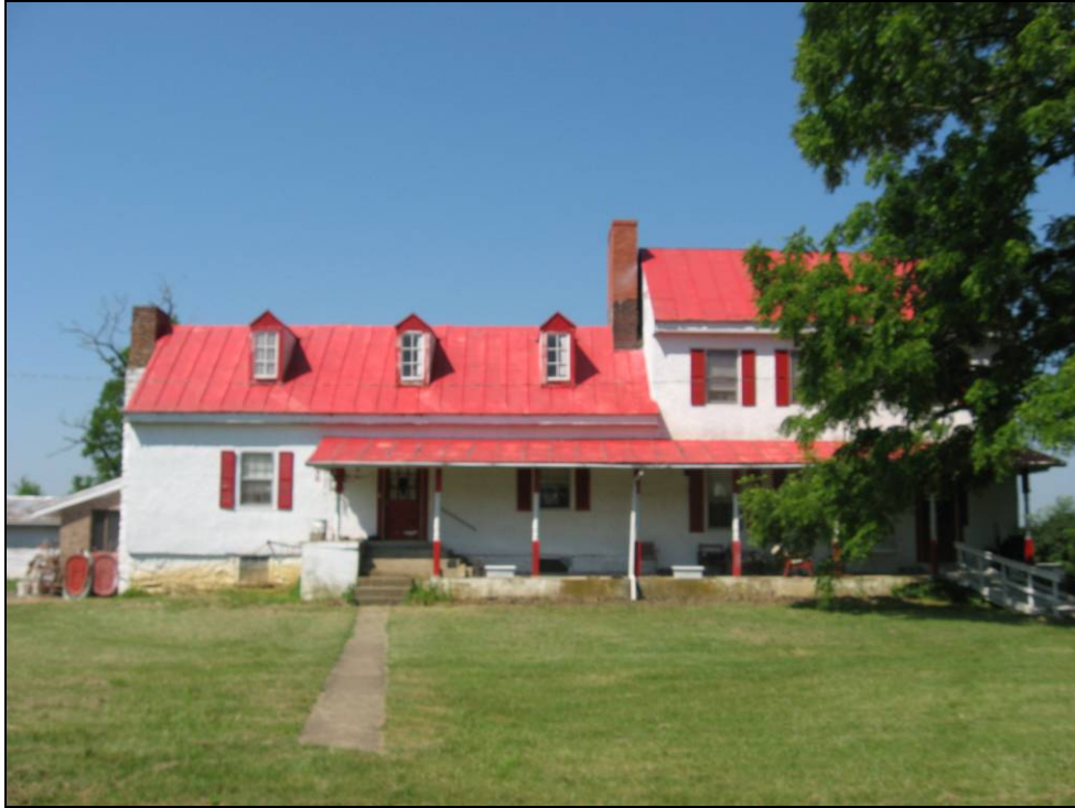
Photo 47: Primary (East) Elevation of Level Green (023-5147).
