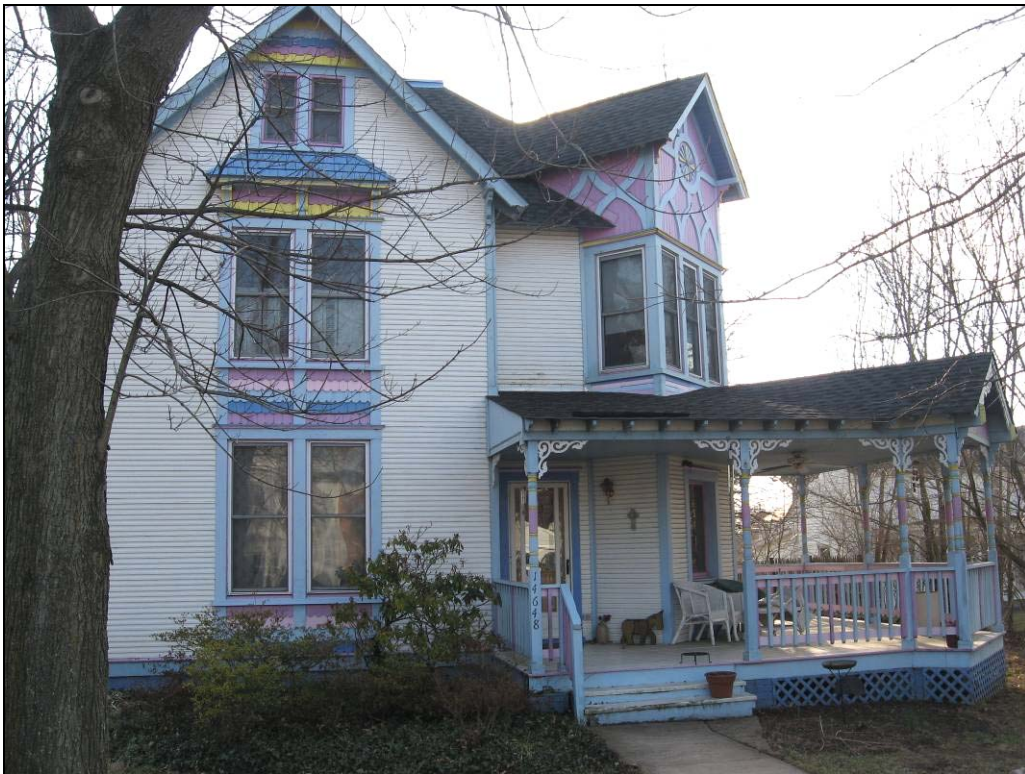
Photo 5: House at 14648 Carrico Mills Road (023-5132), Primary Elevation.
