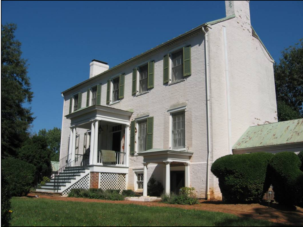
Photo 29: The Main House at North Cliff (023-5349), Southeast Oblique.
