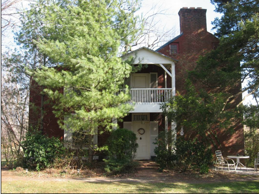
Photo 35: West Elevation of the Fishback House (023-5276).
