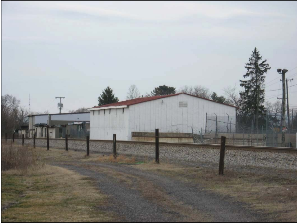
Photo 6: Warehouse at 19424 Brandy Road (023-5110), Looking Northwest.
