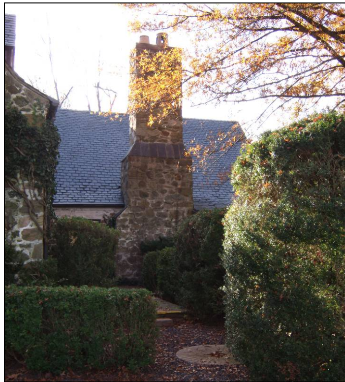
Photo 19: Detail of Stone Chimney and Slate Roof at Brandy Rock Farm.
