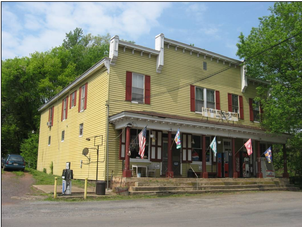
Photo 80: Rapidan General Store (023-5307), Northeast Oblique.
