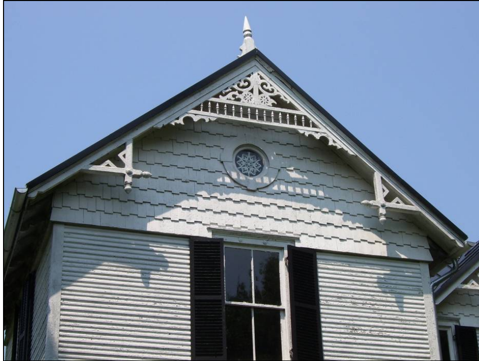
Photo 37: Architectural Detail of The Glebe (023-5271).
