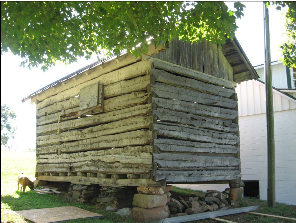
Photo 32: Corn Crib at North Cliff (023-5349), Northwest Oblique.
