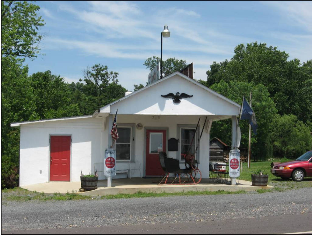
Photo 10: Proctor's Store (023-5286), East Elevation Facing Route 15.
