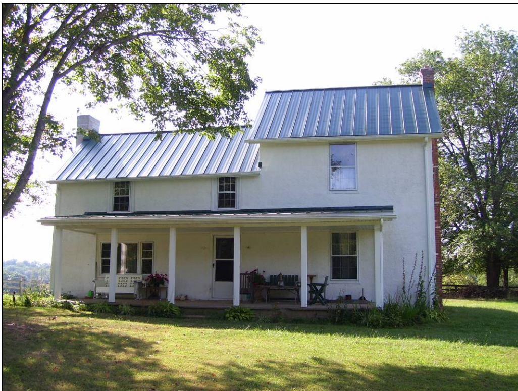
Photo 30: Edgewood (023-5344), Primary (West) Elevation.
