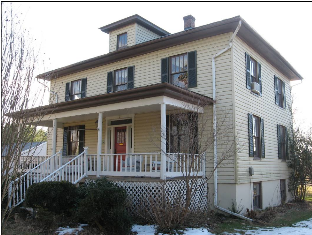
Photo 57: House at 23506 Lignum Road (023-5243), North Oblique.
