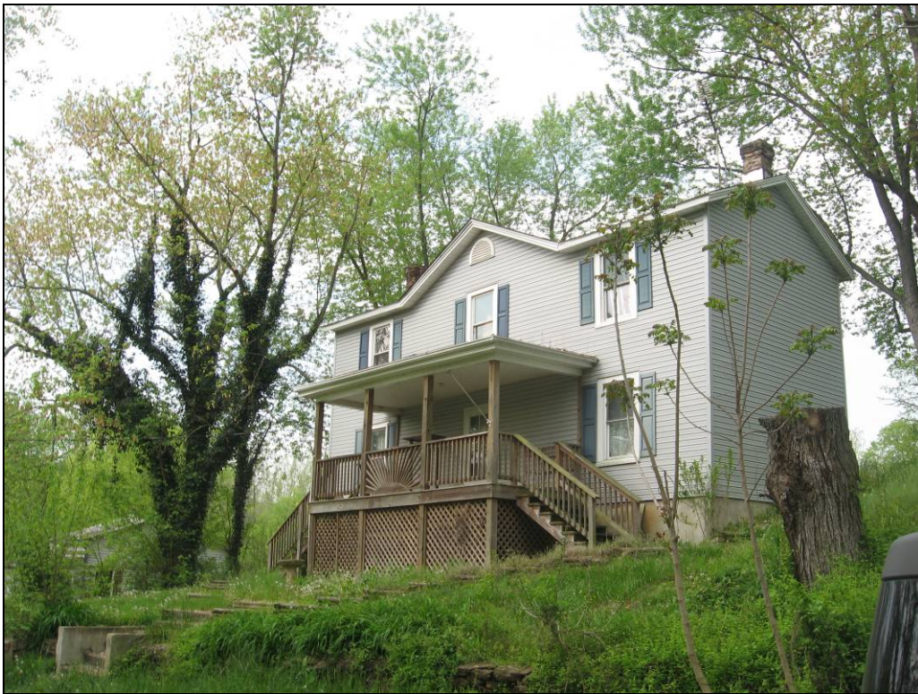
Photo 75: House at 17212 Raccoon Ford Road (023-5298), Northeast Oblique. Note the modifications including new siding, new windows and a new porch.
