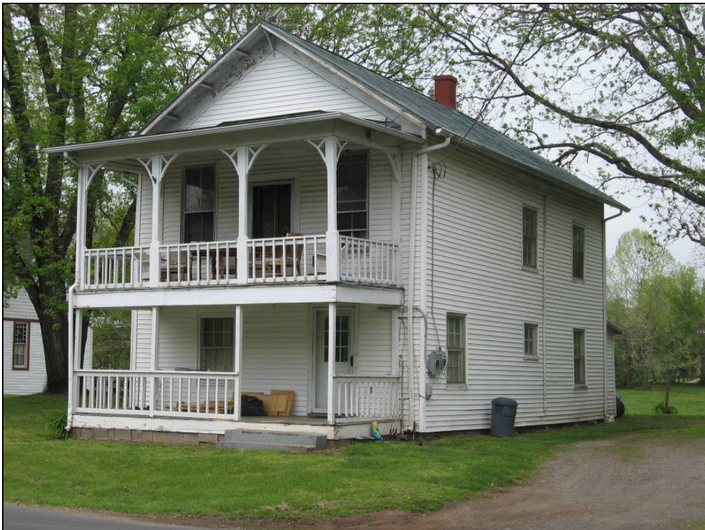
Photo 77: House at 28282 Rapidan Road (023-5308), Northeast Oblique.
