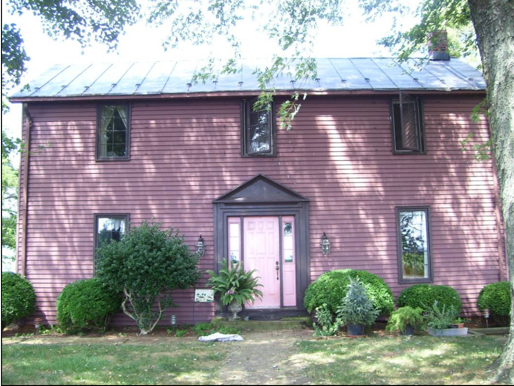
Photo 31: Haught Place (023-5346), Primary (South) Elevation.
