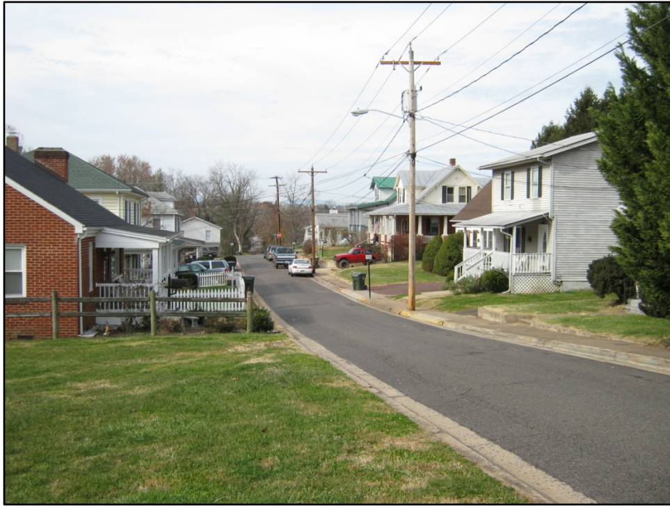
Figure 13. View of residential resources on West Culpeper Street, facing west.
