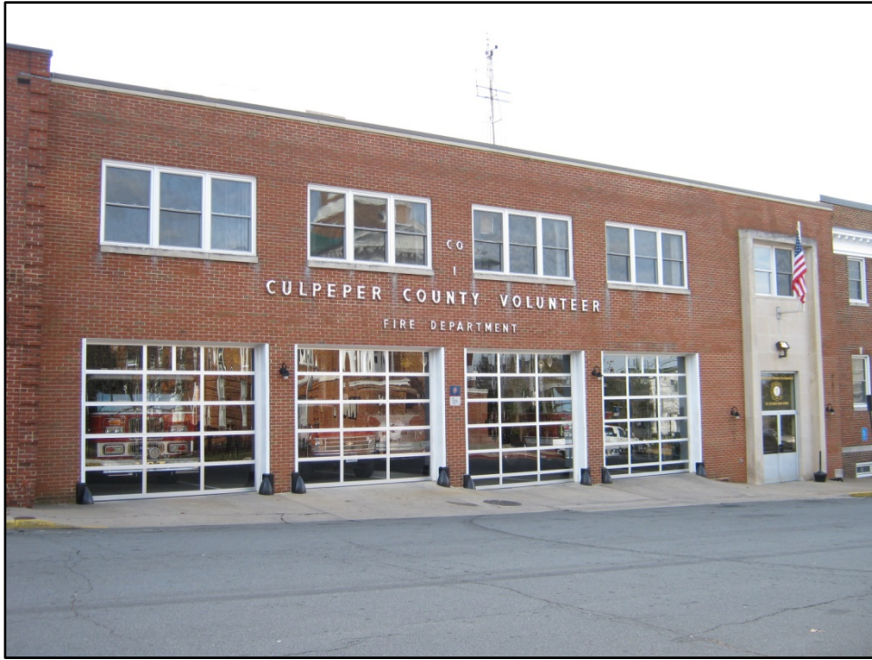
Figure 9: Fire Station, 151 West Davis Street, facing southwest.
