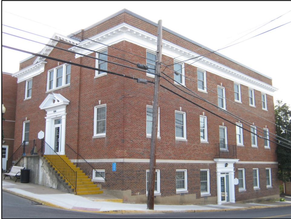
Figure 8. County Office Building, 155 West Davis Street, facing south.
