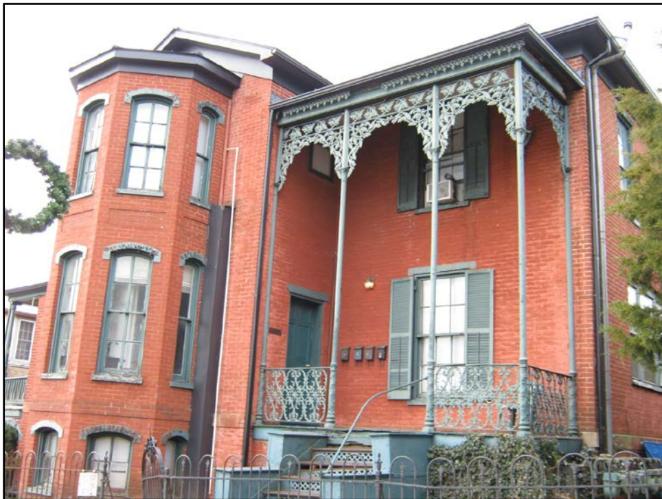
Figure 18. 606 North Main Street, facing southeast.
