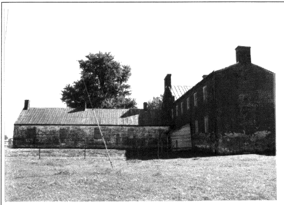
FIGURE 72: Poorhouse 34-99, rear view of main block and north wing.
