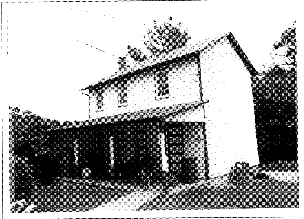
FIGURE 39: Brumback-Douglas House 34-1421, south view summer kitchen.
