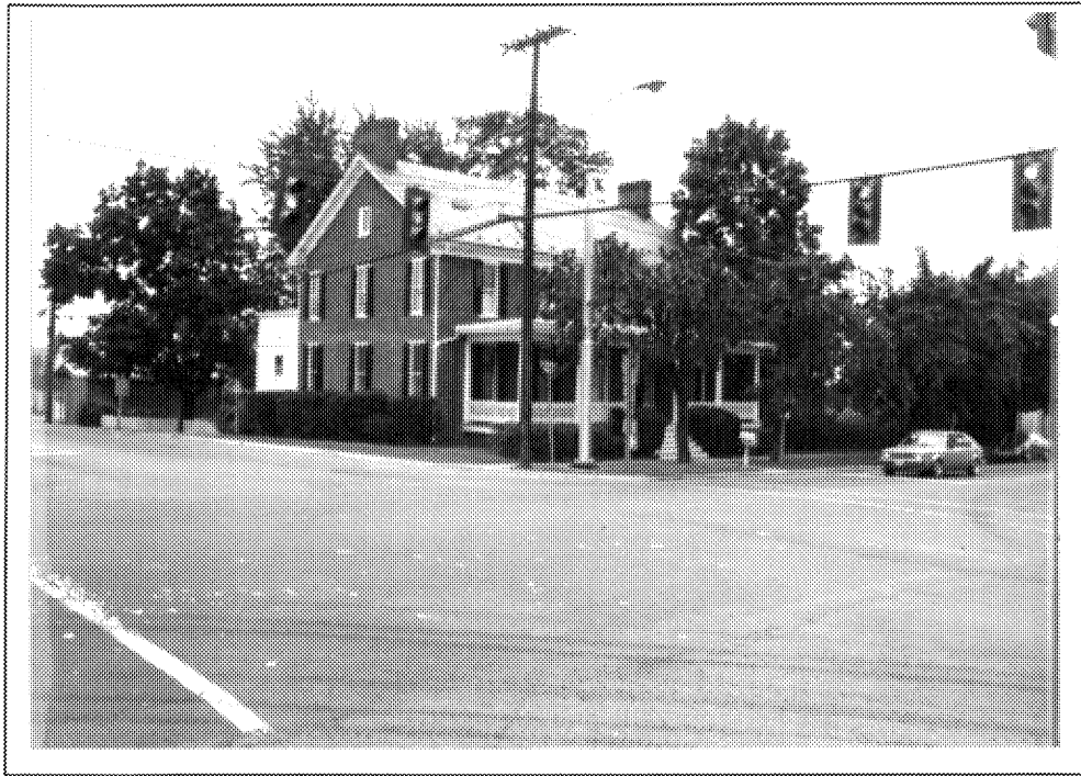
FIGURE 93: Tavern, The 304-65, nw view.
