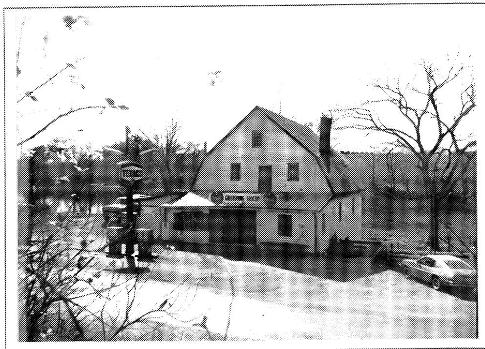
FIGURE 90: Green Springs Grocery 34-151, north view.
