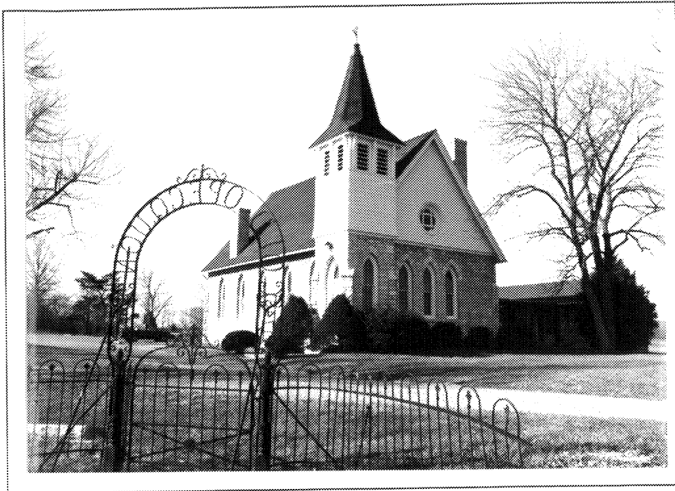
FIGURE 83: Opequon Presbyterian Church 34-9, ne view.
