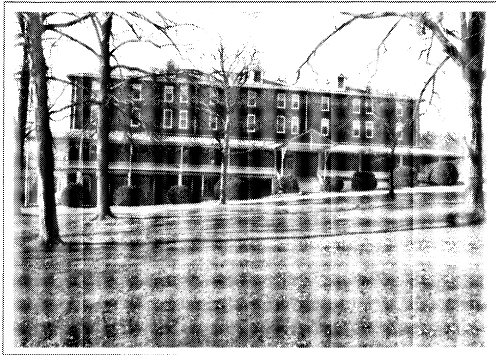
FIGURE 67: Suflur Spring Spa 34-110, north view.
