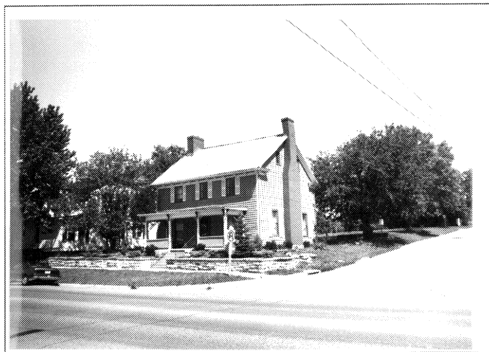
FIGURE 98: 7846 Main Street (Danner House) 260-35, se view.
