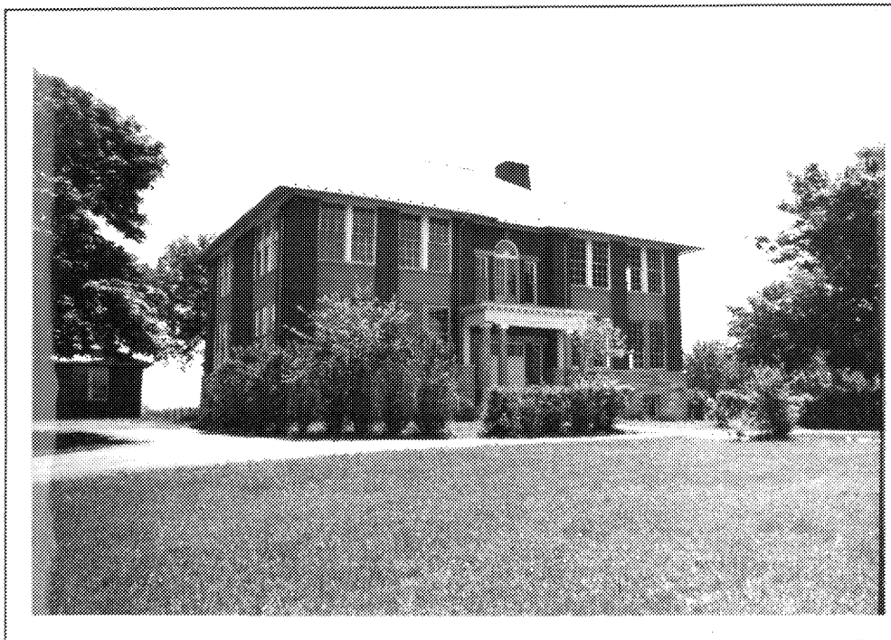
FIGURE 96: Middletown School 260-4, nw view.
