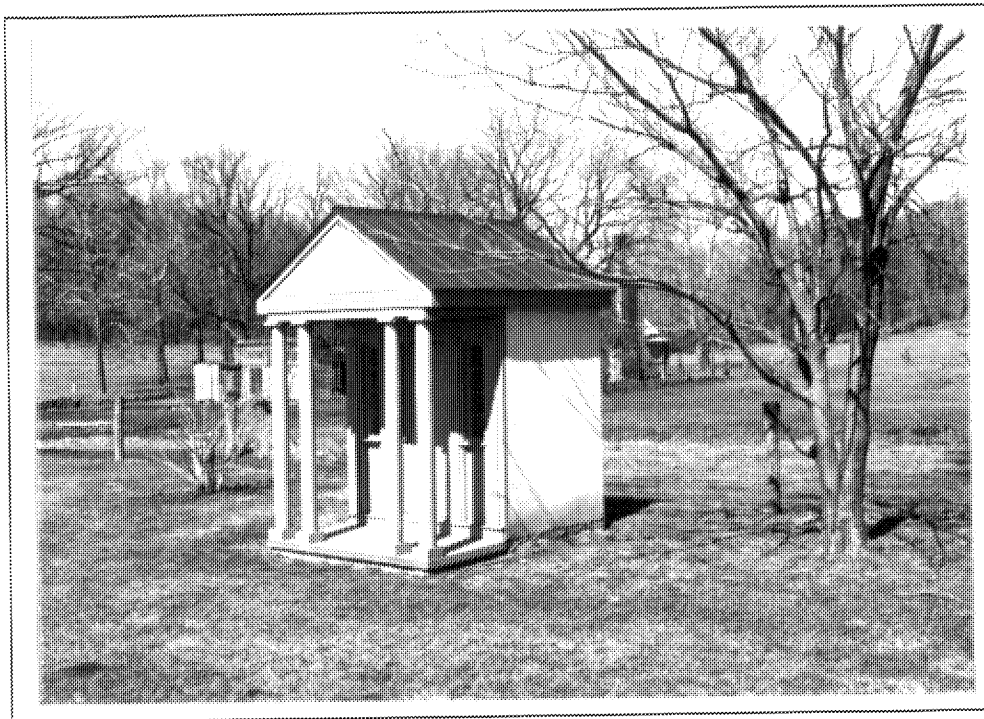
FIGURE 47: Rosedale 34-11, se view of privy.
