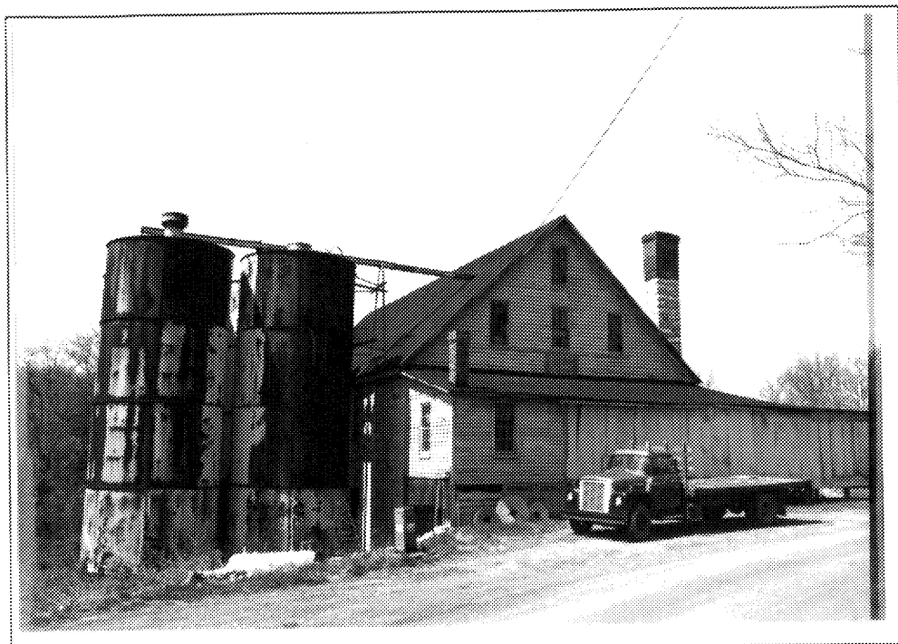
FIGURE 89: Springdale Flour Mill 34-128, east view.
