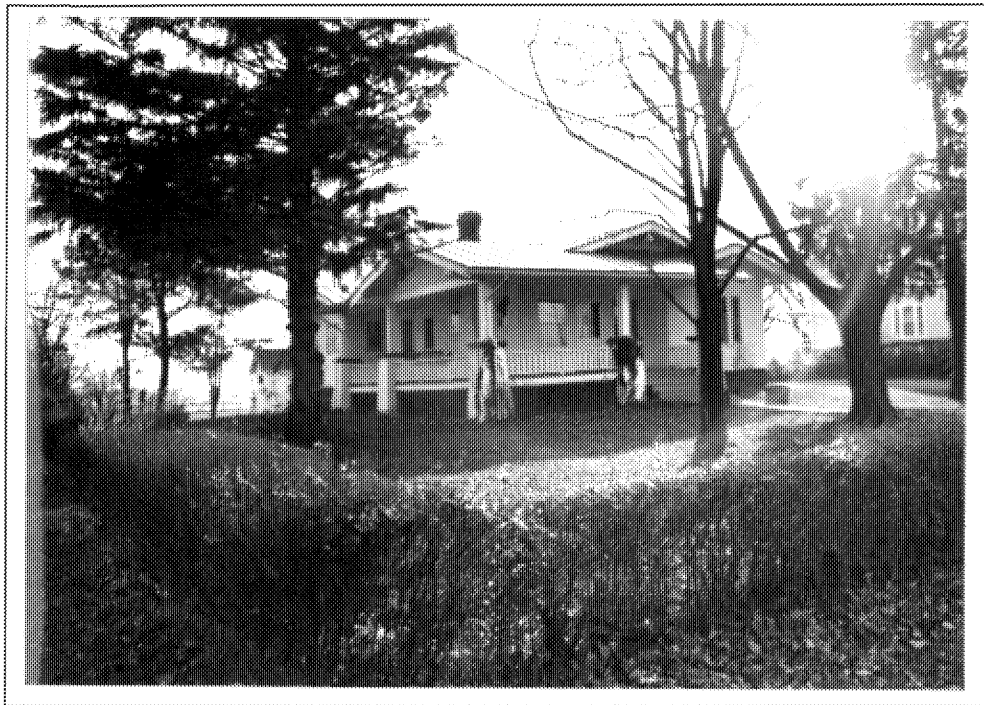
FIGURE 33: Martin-Hollis House 34-994, ne view.
