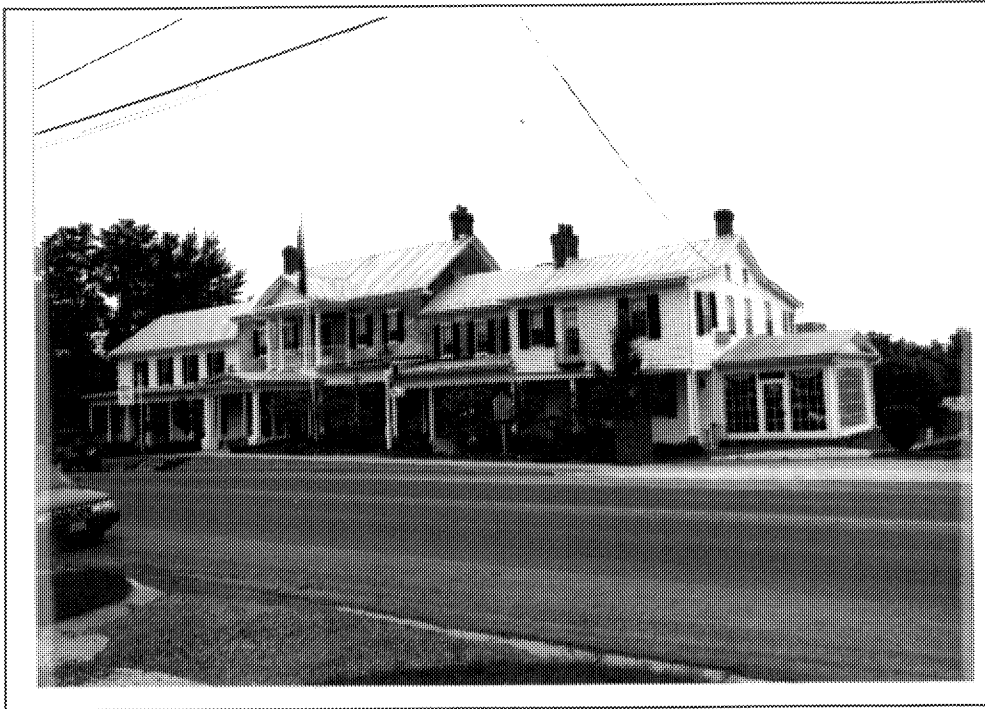
FIGURE 95: Wayside Inn 260-2, ne view.
