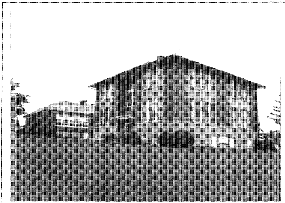
FIGURE 94: Stephens City School 304-80, sw view.
