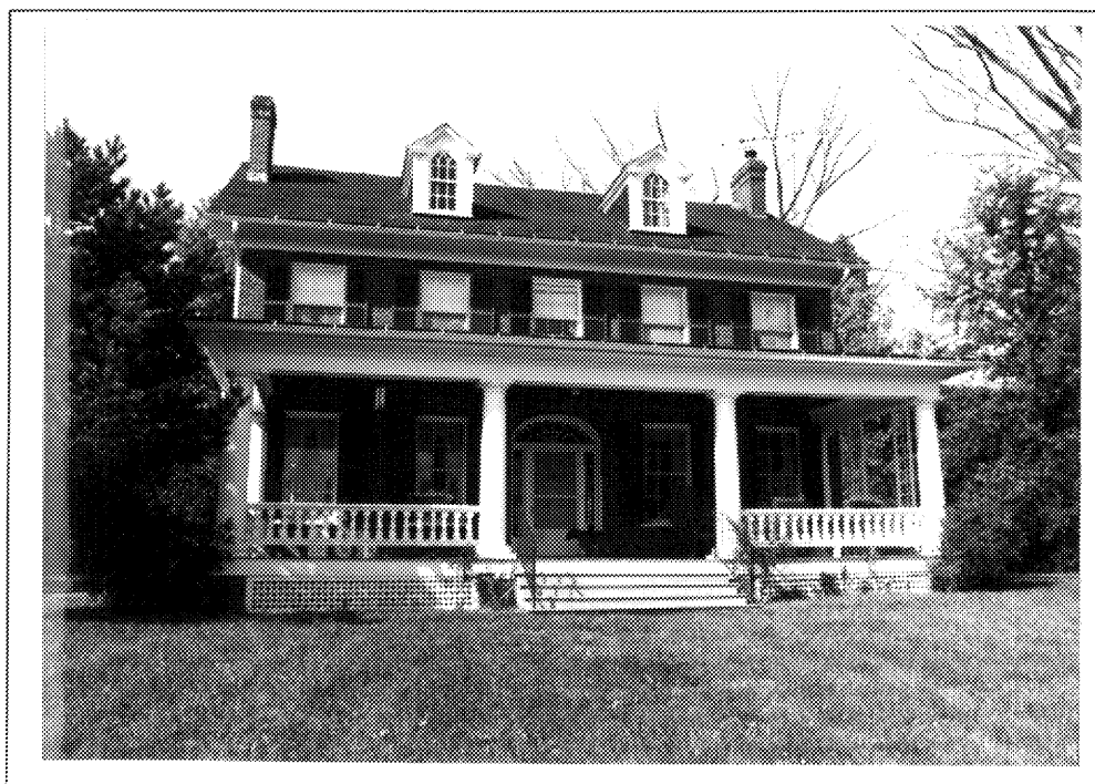
FIGURE 34: Bond House 34-70, east view.
