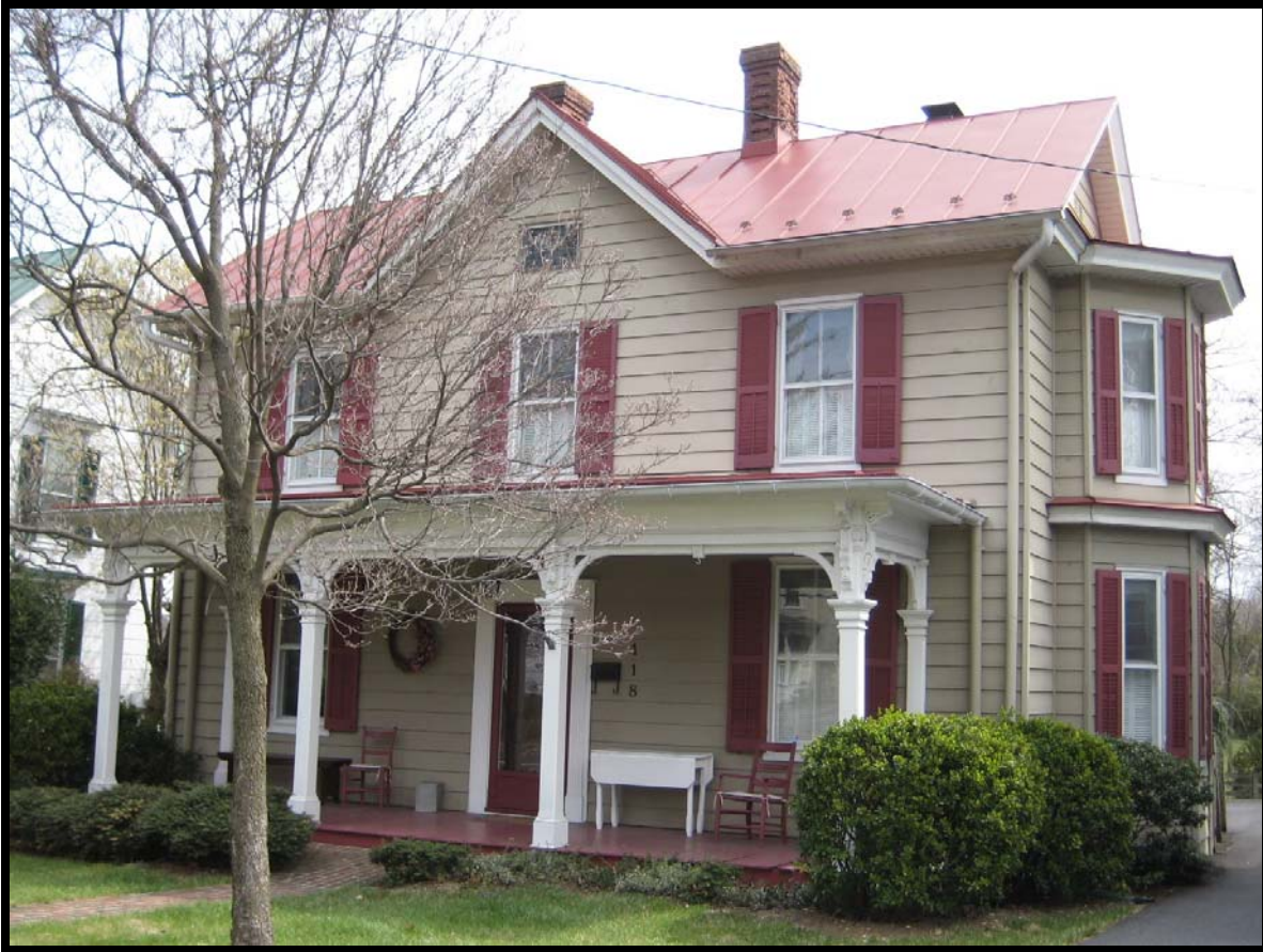
Figure 13: House, 418 Fairmont Street, 138-0042-0440 (EHT Tracerics, 2011)
