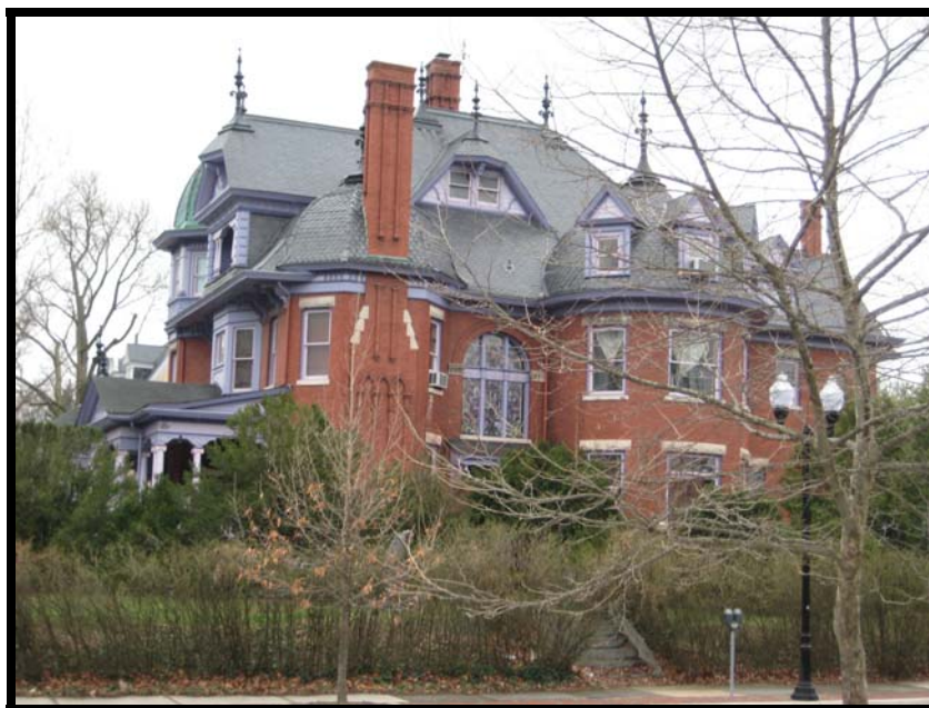
Figure 11: The Gables, 5 South Washington Street, 138-0042-0994 (EHT Tracerries, 2011)
