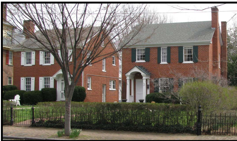
Figure 20: Houses, 210 and 212 South Washington Street, 138-0042-1006 and 1007 (EHT Tracerics, 2011)
