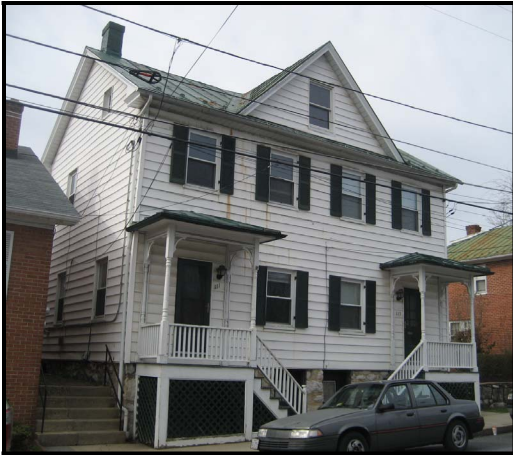
Figure 14: Twin Dwelling, 111-113 West Cork Street, 138-0042-0398 (EHT Tracerics, 2011)
