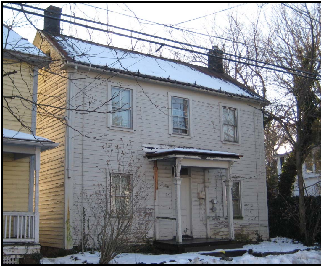
Figure 12: House, 123 West Leicester Street, 138-0042-0626 (EHT Tracerics, 2011)
