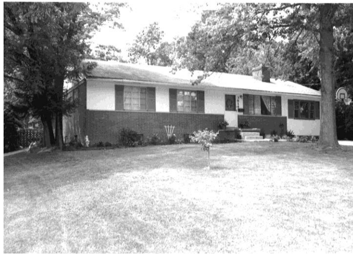
Figure 48: House, 3814 Ren Road, 151-5429 (EHT Tracerics, 2004)
