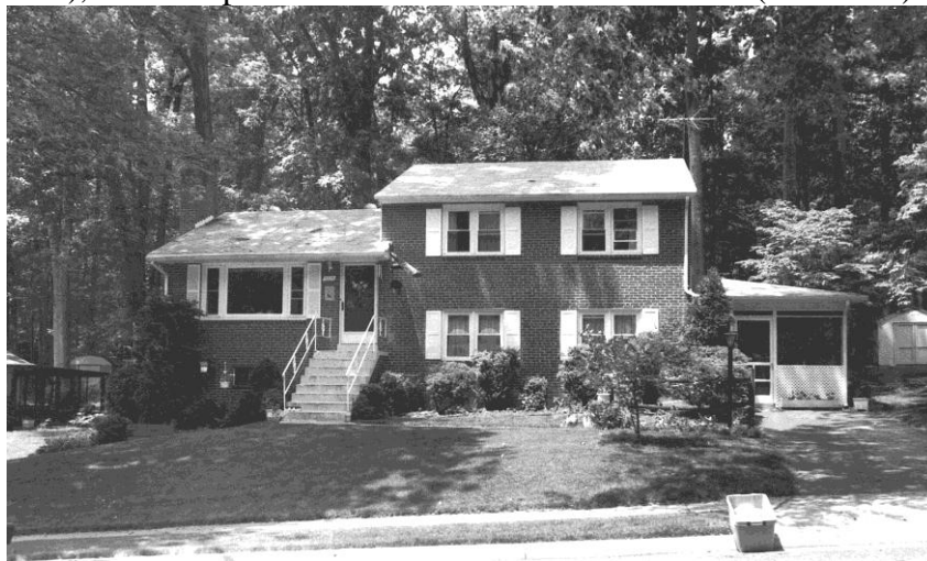
Figure 21: House 4238 Berritt Street, 151-5113 (EHT Tracerics, 2004)
