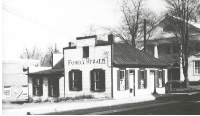
Figure 38: Fairfax Herald Building, 10400 Main Street, 151-0003-0037 (EHT Tracerics, 2004)
