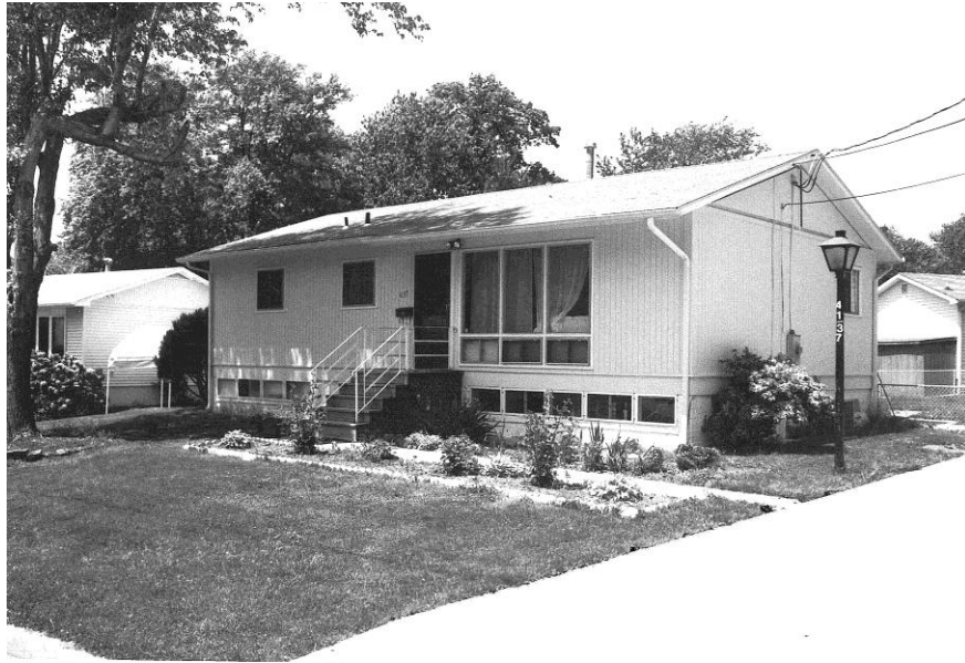
Figure 34: House, 4137 Locust Lane, 151-5054 (EHT Tracerics, 2004)
