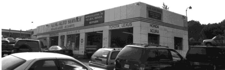
Figure 41: A.I.M. Auto Service Building, 10550 Lee Highway, 151-5230 (EHT Tracerics, 2004)
