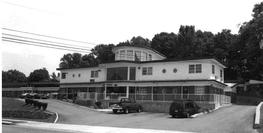
Figure 53: Anchorage Motel, 9865 Lee Highway, 151-5226 (EHT Tracerics, 2004)
