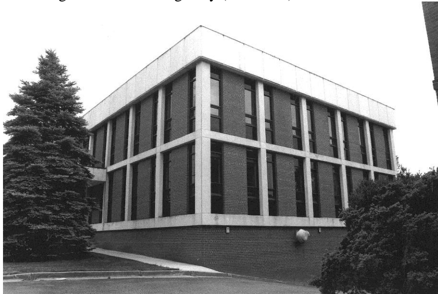
Figure 22: Office Building, 10523 Main Street, 151-5456 (EHT Tracerics, 2004)
