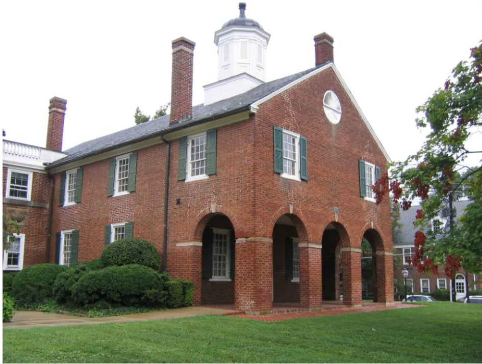
Figure 59: Fairfax County Courthouse, 4000 Chain Bridge Road, 151-0003-0001 (EHT Tracerics, 2004)
