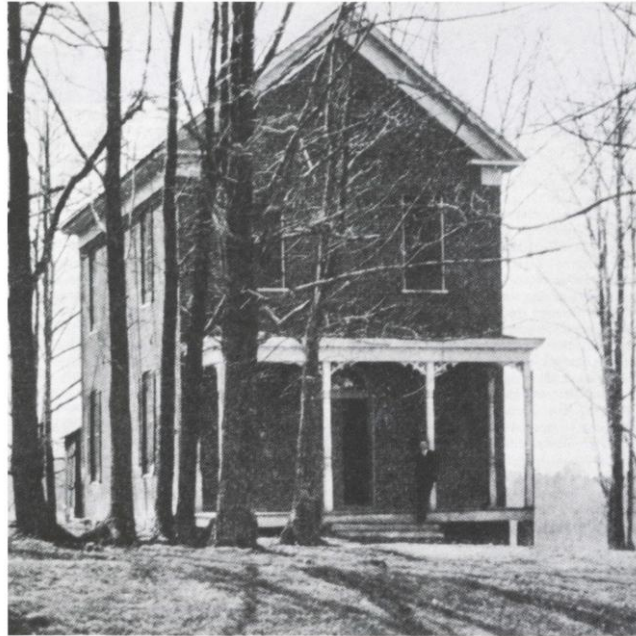
Figure 8: Fairfax Elementary School ( Fairfax, Virginia: A City Traveling Through Time , p. 36)
