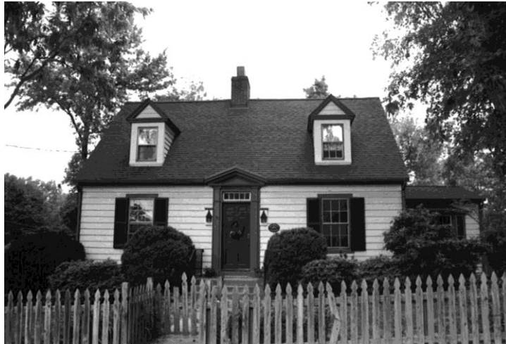
Figure 44: House, 10618 Moore Street, 151-5265 (EHT Tracerics, 2004)
