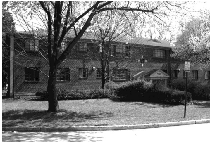
Figure 51: Yorktown Apartments, 4020 Yorktown Drive, 151-5017 (EHT Tracerics, 2004)
