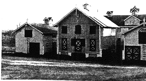
Barn at Thorncliff (038-5148)
