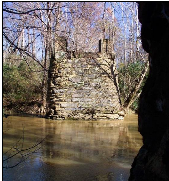
Figure 2.5: Stone Piers of King's Bridge
