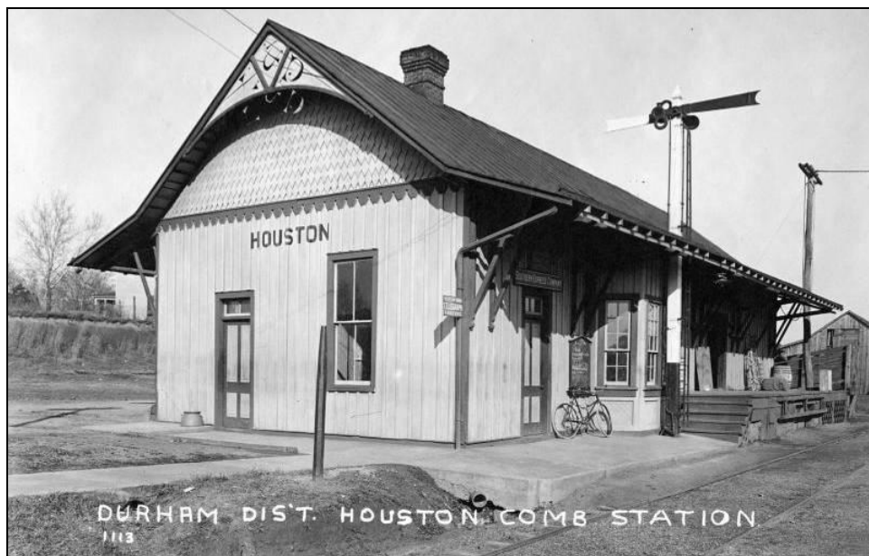
Figure 3.48: Houston Railroad Depot
