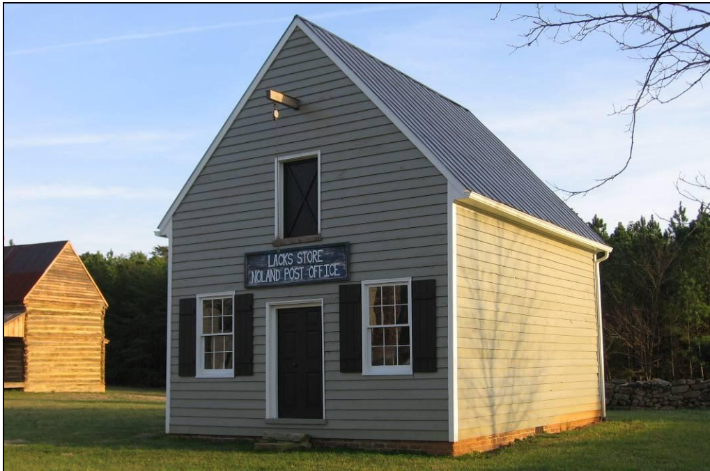
Figure 3.14: Noland Village Post Office/Lacks Store (041-5291) Source: HSPC, Dec. 2006
