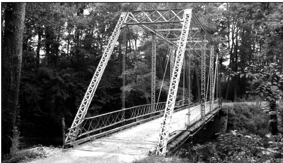
Figure 3.50: Aarons Creek Bridge (041-5081)
