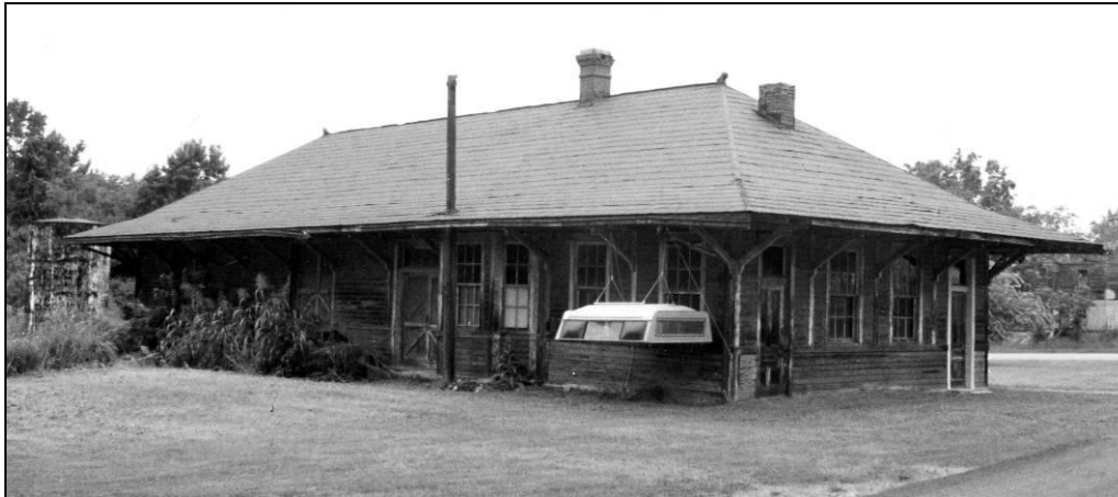
Figure 3.49: Virgilina Railroad Station (318-5007)
