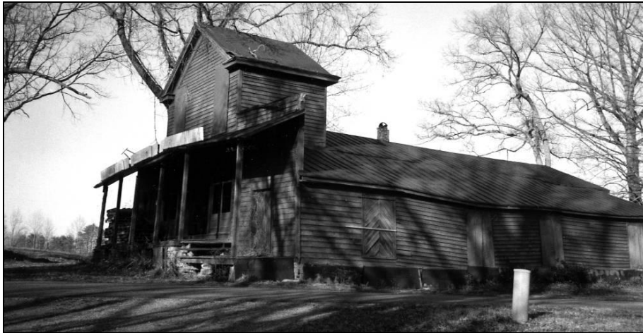
Figure 3.41: Old General Store along Birch-Elmo Road (041-5222)
