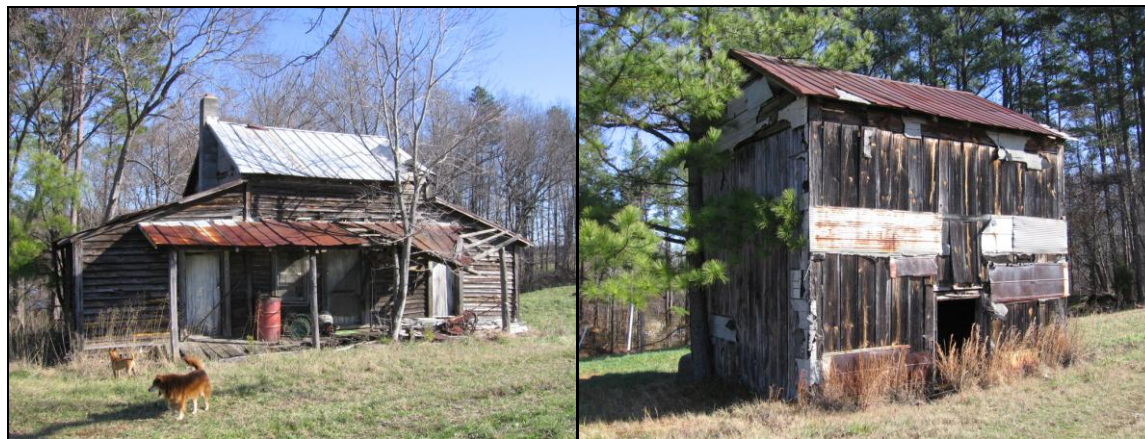
Figure 2.17: Tenant House and Tobacco Barn, Sandy Level Farm Source: HSPC, 2007
