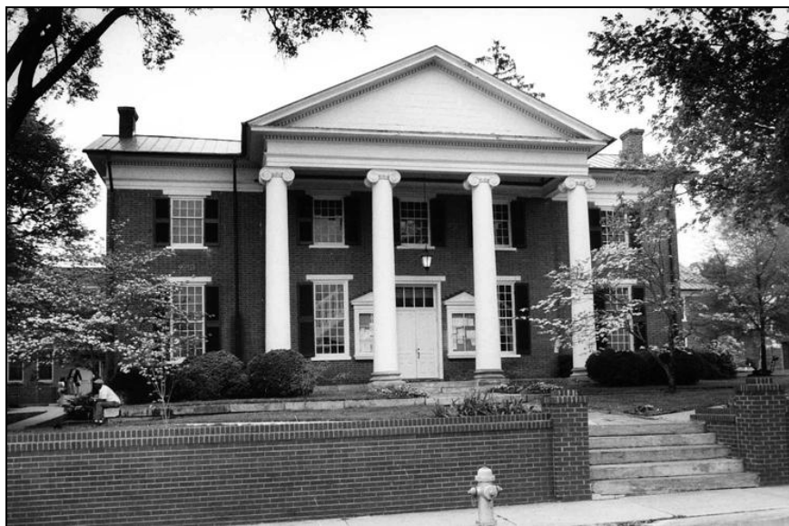
Figure 2.11: Halifax County Courthouse (230-0077)
