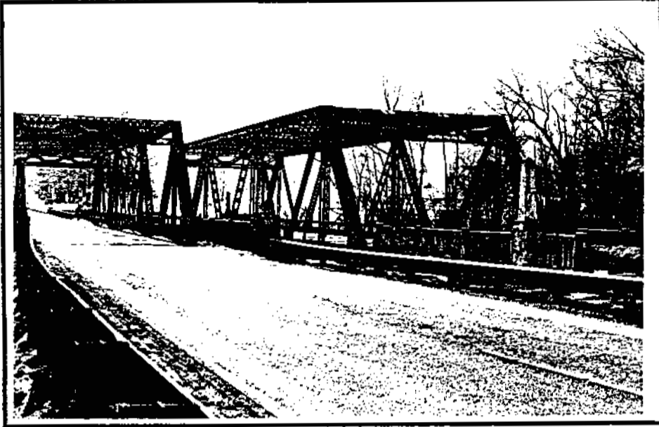
Fig. 68. North End, Fox Bridge (DHR 42-401). (Land and Community Associates)
