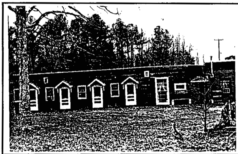
Fig. 76. Hotel Comfort (DHR 42-315). (Land and Community Associates)
