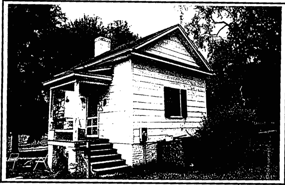
Fig. 41. School, Ingleside (DHR 42-17). (Land and Community Associates)
