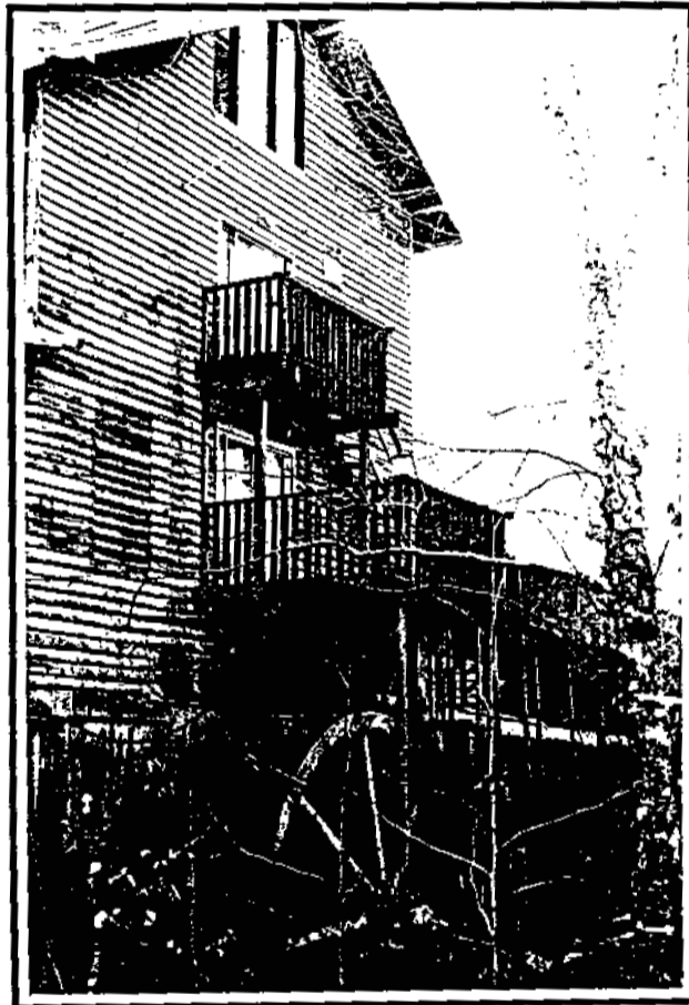
Fig. 66. King Pond Mill (DHR 42-91). (Land and Community Associates)
