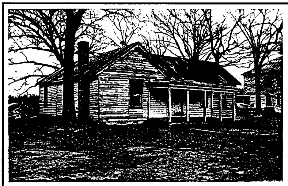
Fig. 46. Old School, Route 33 (DHR 42-485). (Land and Community Associates)
