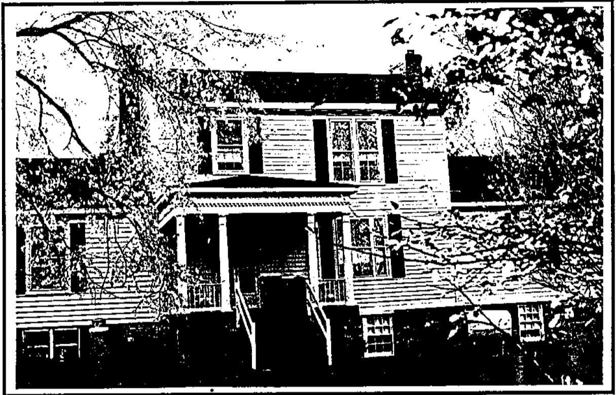
Fig. 17. Rear elevation, Westwood (DHR 42-59). (Land and Community Associates)
