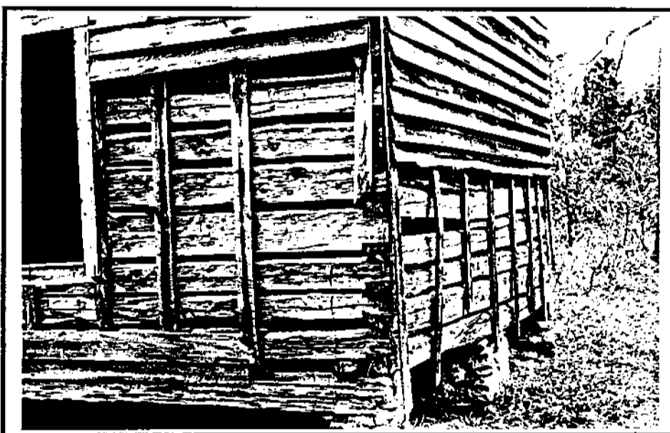
Fig. 13. Exterior corner detail, Log House (DHR 42-450). (Land and Community Associates)
