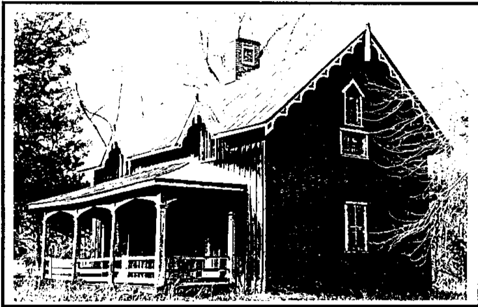
Fig. 24. Library, Hickory Hill (DHR 42-100). (Land and Community Associates)
