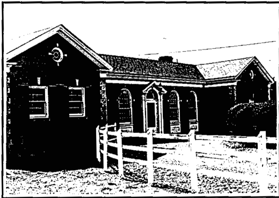
Fig. 74. Doswell Station (DHR 42-93). (Land and Community Associates)
