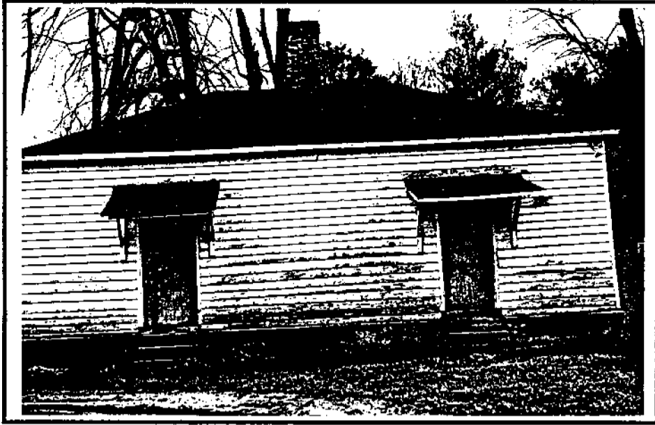
Fig. 23. Kitchen, Hickory Hill (DHR 42-100). (Land and Community Associates)
