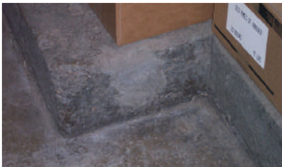
Above: Platform in rear cell, plugged clean out hole.
