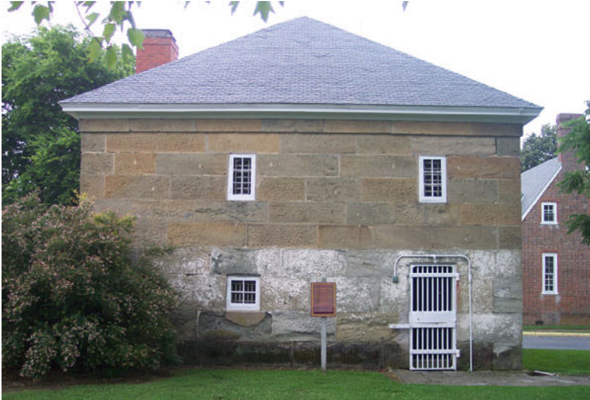
Above: South elevation of jail
