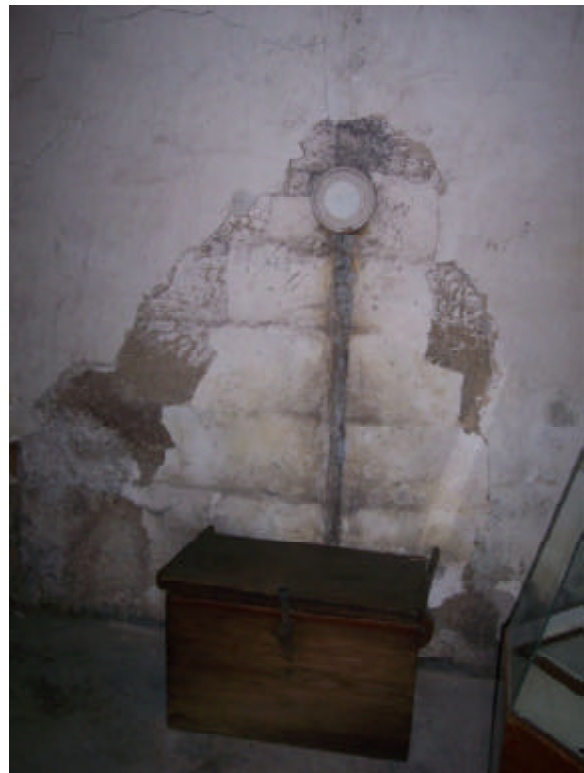
Above: Chimney breast - Front cell - Ground Floor.
