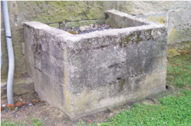
Above: Cesspit for south cell.
