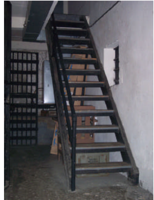
Above: First floor interior.
