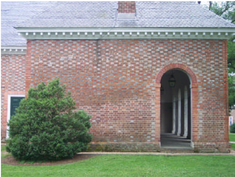
Above: North elevation - Piazza and North Jury Room.
