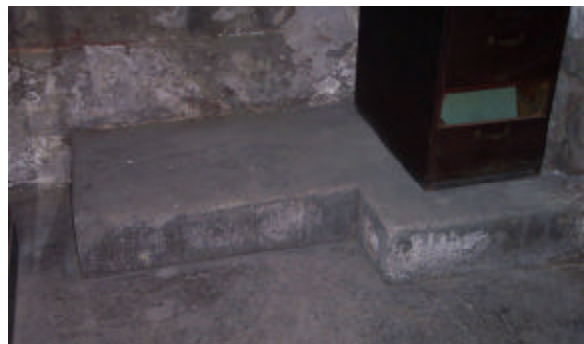
Above: Concrete platform, front cell.
