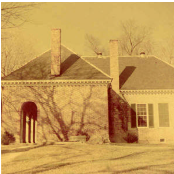
Above: South elevation - c. 1954
