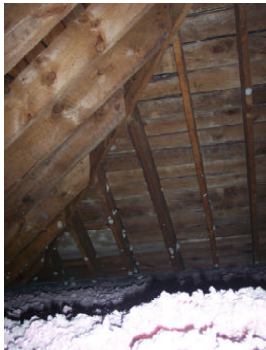
Above: Attic in jail.
