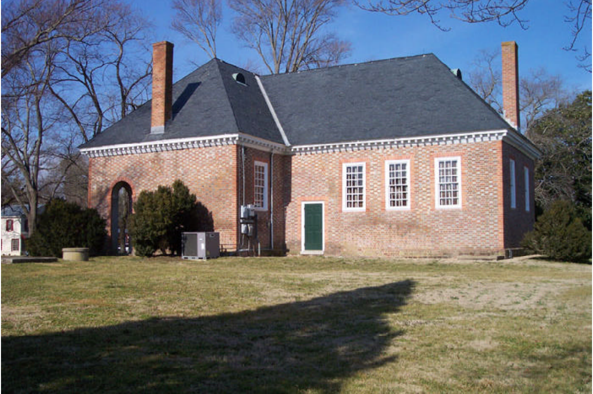
Above: South elevation of courthouse.
