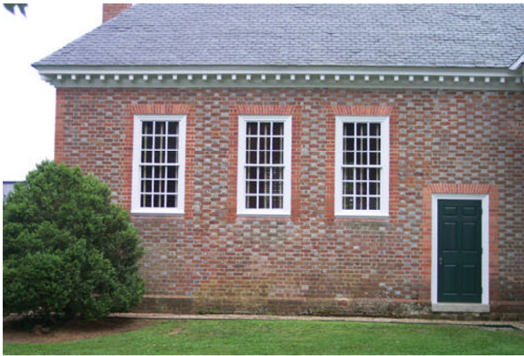
Above: North elevation - Courtroom.
