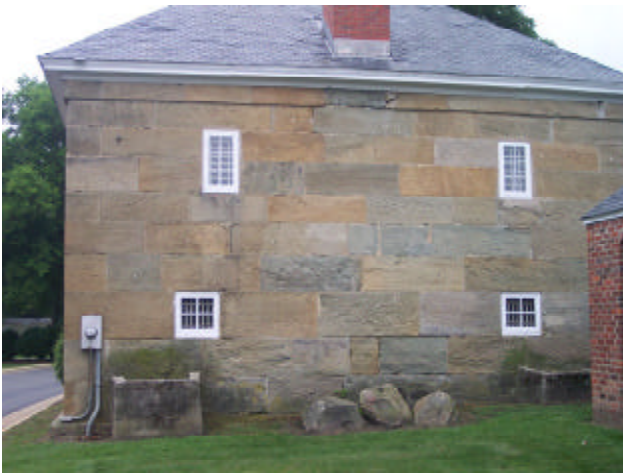
Above: East elevation of jail.
