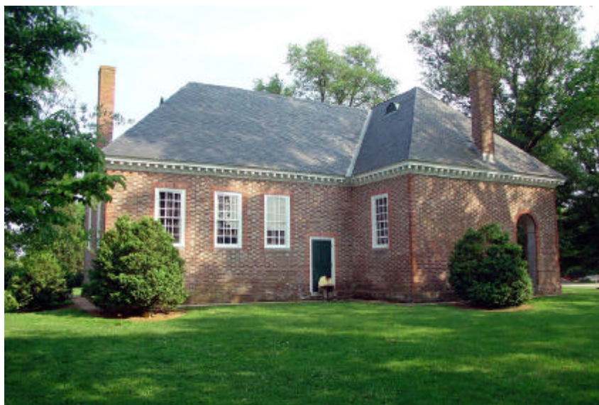
Above: The courthouse from the northeast. The roof ventilators date from the 1955 renovation.
