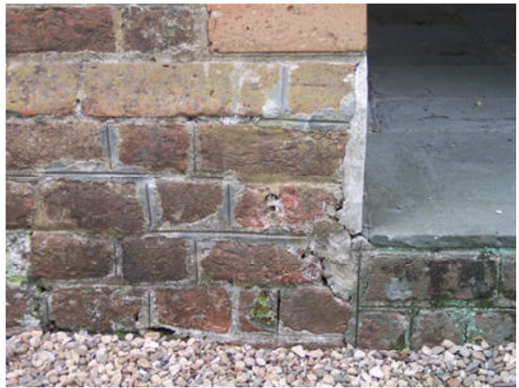
Above: North jamb of arched opening.
