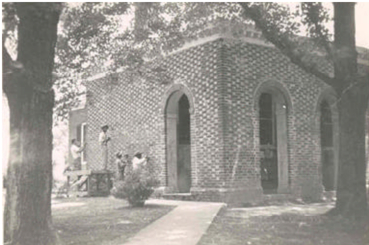
Above: Repainting the Courthouse walls, c. 1955.
