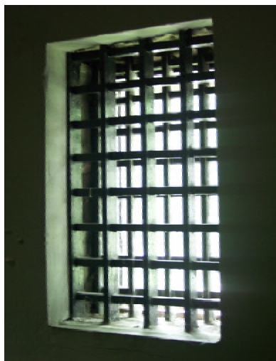
Above: West window - second floor passage.
