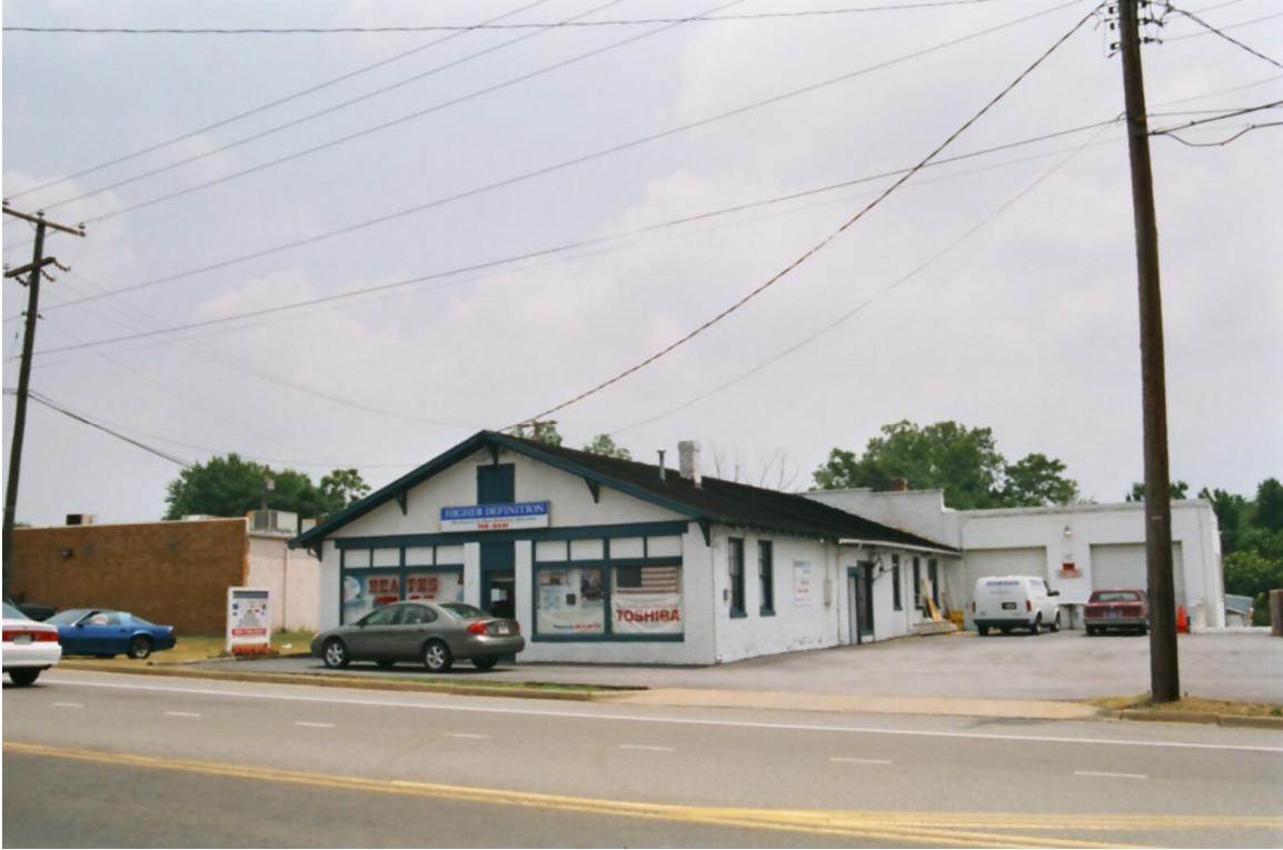
Plate 6. The former Mechanicsville Motor Company now Heath's TV.
