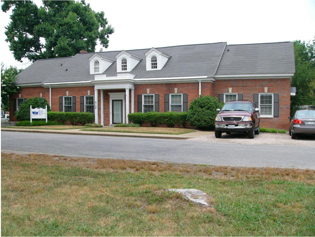
Plate 10. Colonial Revival-style office building in the Virginia Manor area.
