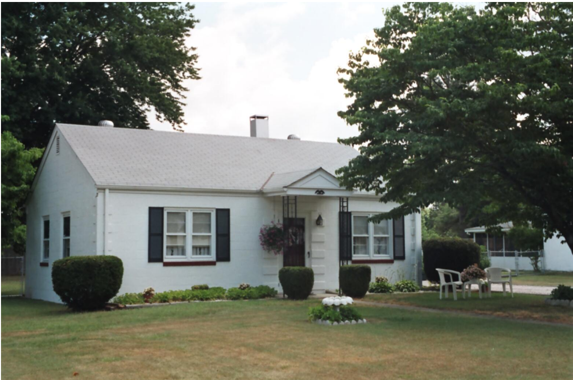
Plate 15. Concrete-block with raised quoins, three-bay façade.
