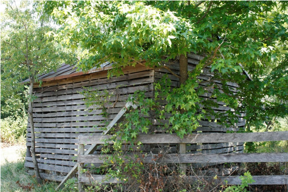
Plate 12. Corncrib on 042-5393. Note the widely spaced boards for ventilation.
