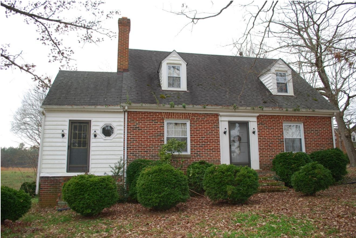
Plate 2. Colonial Revival-style brick house (042-5355)
