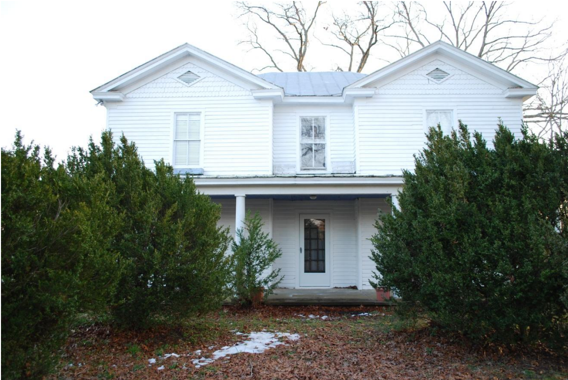
Plate 8. House (042-5378) with parallel projecting gables
