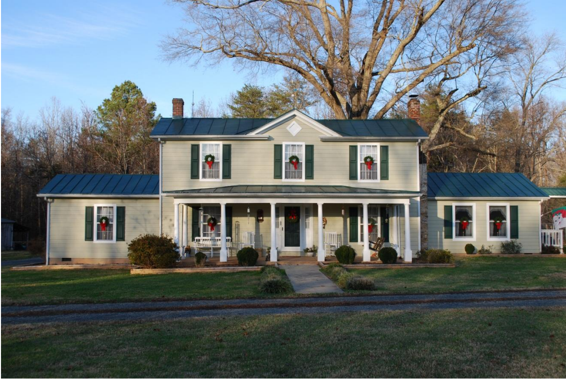
Plate 5 I-house with exterior-end stone chimney (042-5375)
