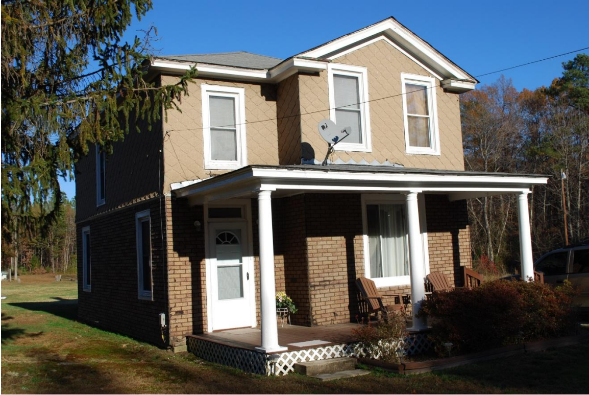
Plate 1. House (042-5323) with bricktex siding
