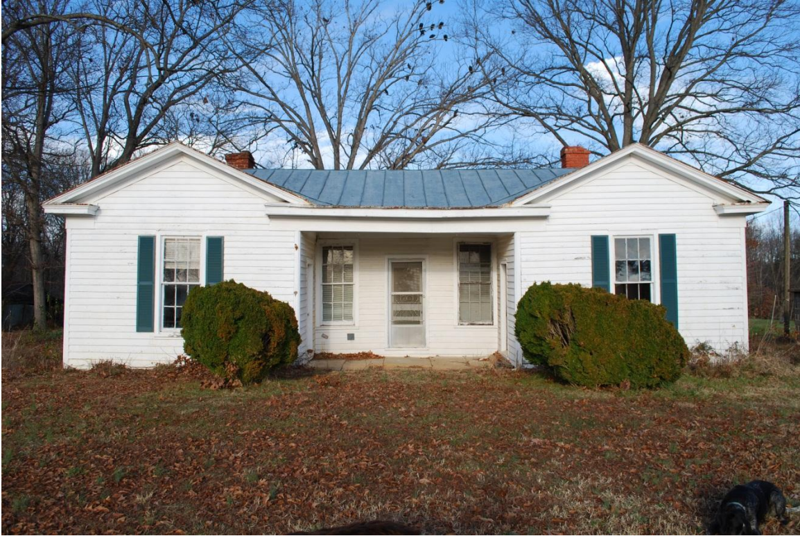
Plate 7. House (042-5353) with parallel projecting gables
