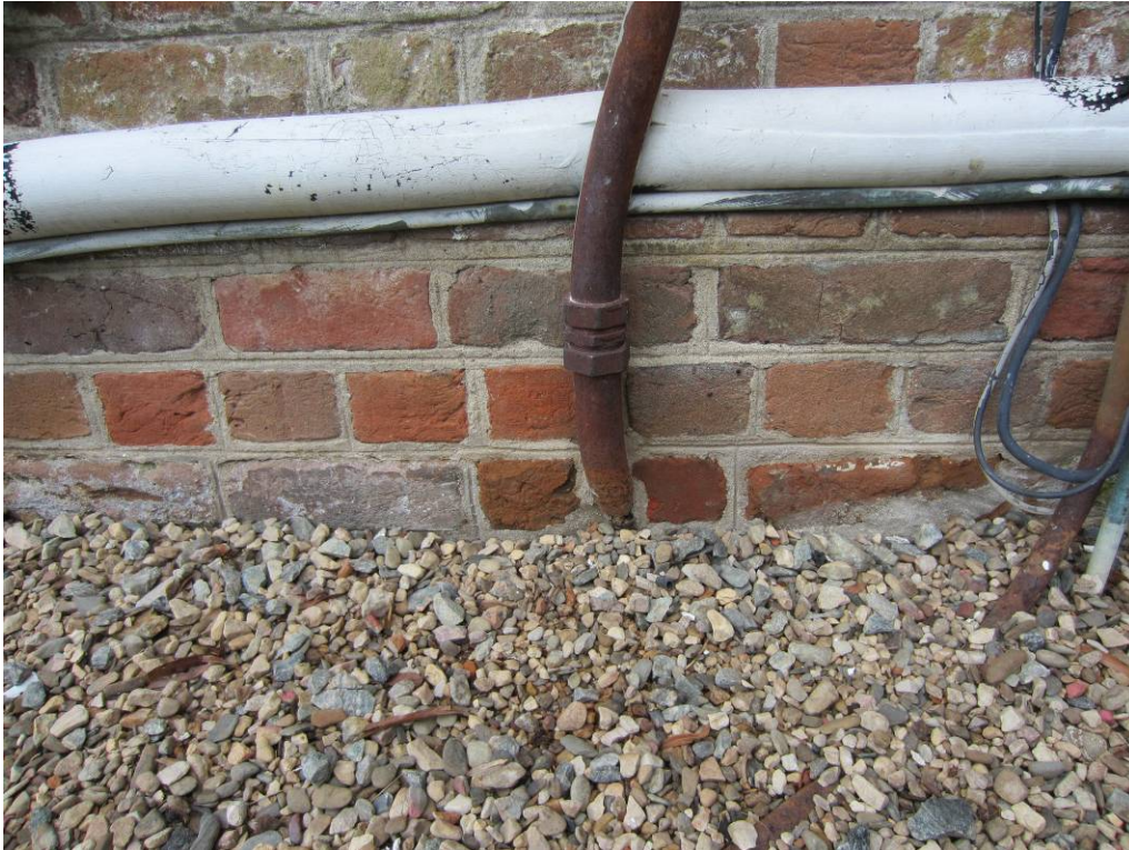
Detail of brick infill on the east elevation after treatment.
