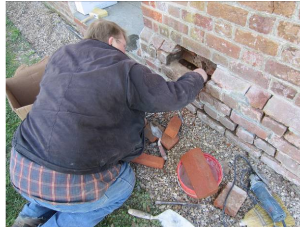
(Left) Existing condition of the base of the building on the north elevation, before restoration work. (Right) Removing deteriorated and damaged brick.
