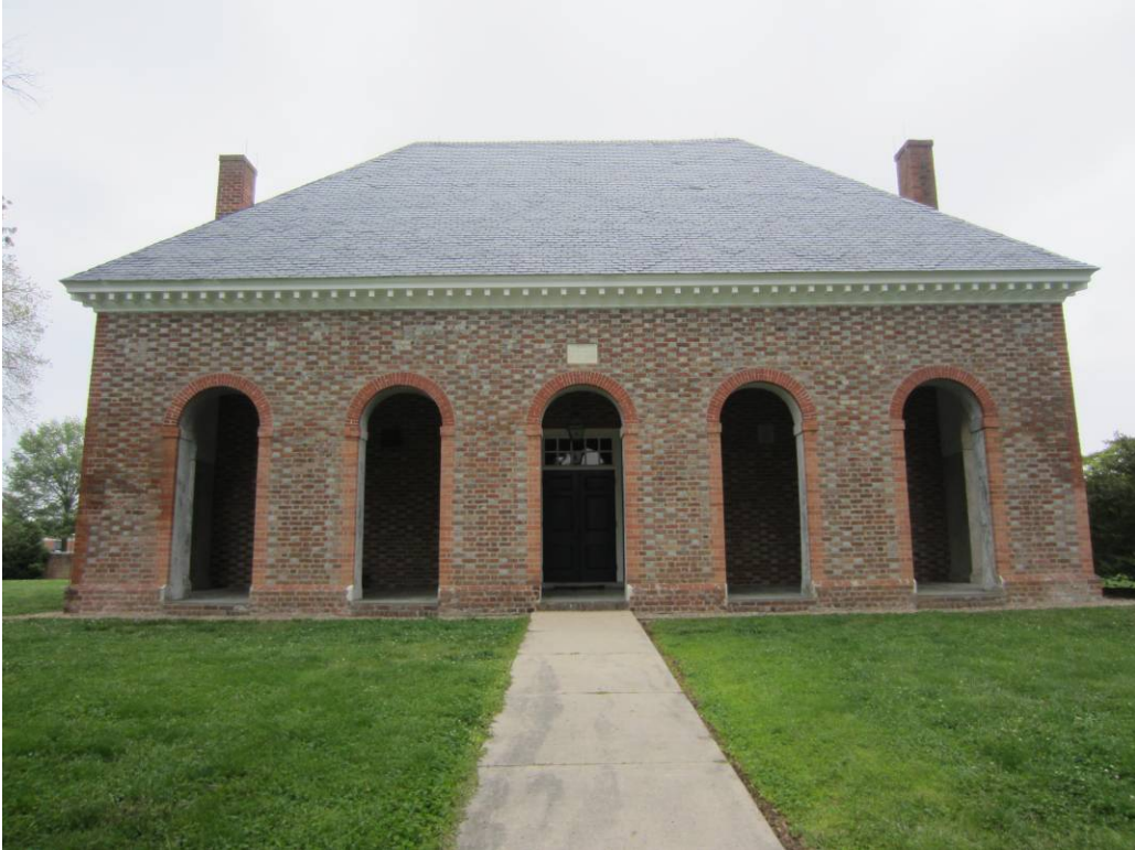
The main (west) elevation after treatment.
