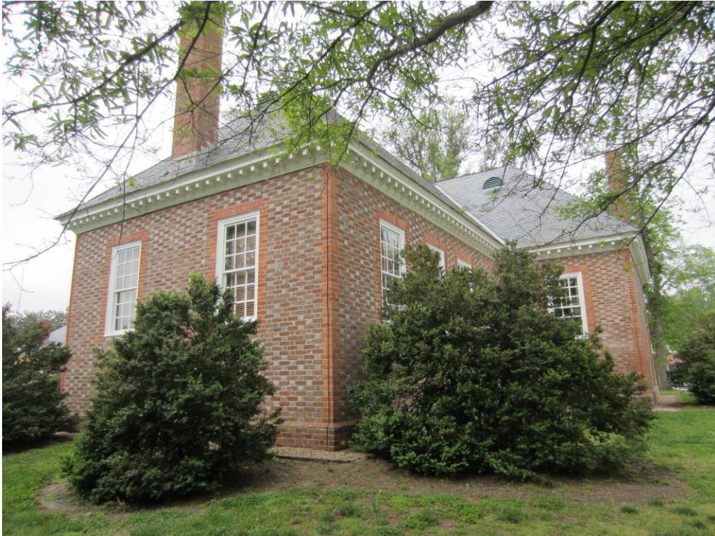
The east elevation after treatment.
