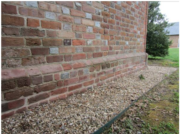
(Left) Installation of original and new brick on the east elevation. (Right) View of work after completion, east elevation.
