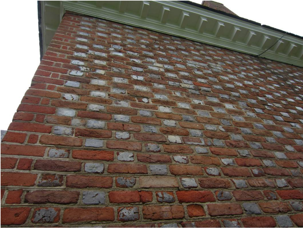
Detail of repointing work on the north elevation after treatment.
