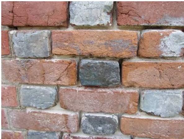
(Left) The glazed header after patching. (Right) Blending in the patching material with mineral stains for masonry.
