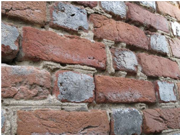
(Left and right) Detailed views of existing conditions of the south elevation before restoration, showing open mortar joints and biological growth. Note the weathered glazing on the headers (left) and biological growth on the masonry (right).
