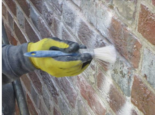
(Left and right) Removing deteriorated mortar and cleaning the joints of all dust and mortar debris.
