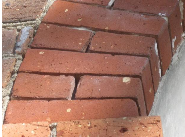
(Left and right) Detailed views of existing conditions of the west elevation before restoration, showing open mortar joints and eroded brick.
