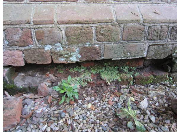
(Left and right) Removing damaged brick and cleaning biological growth on the east elevation.
