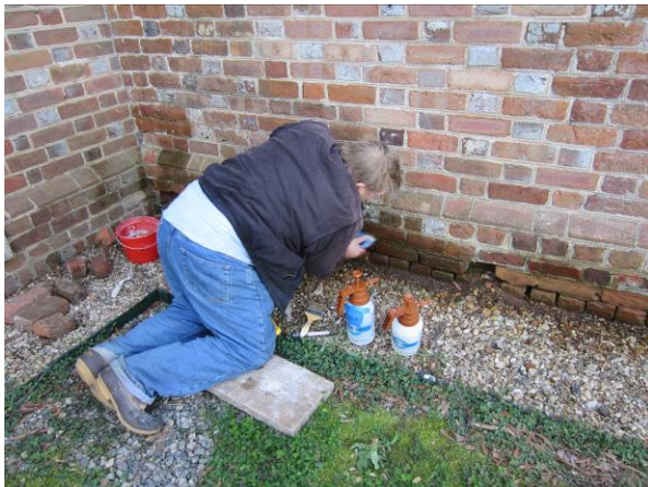
(Left and right) Removing damaged brick and cleaning biological growth on the east elevation.
