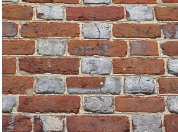
(Left) View of the various repointing campaigns, side by side. (Right) A non-original repointing campaign, in which a white mortar has been used, and the indentation is thin and deep.
