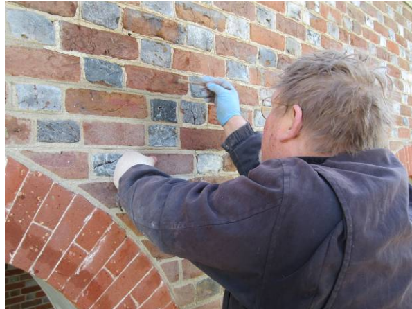
(Left) The glazed header after patching. (Right) Blending in the patching material with mineral stains for masonry.
