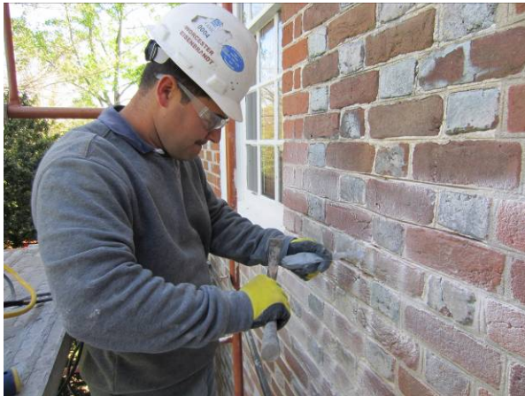
(Left and right) Removing deteriorated mortar and cleaning the joints of all dust and mortar debris.
