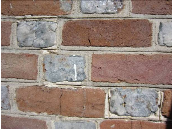
(Left) View of the various repointing campaigns, side by side. (Right) A non-original repointing campaign, in which a white mortar has been used, and the indentation is thin and deep.
