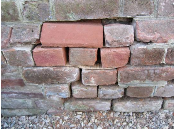
(Left) The new brick inserted in the wall, before setting and repointing. (Right) A damaged glazed header.
