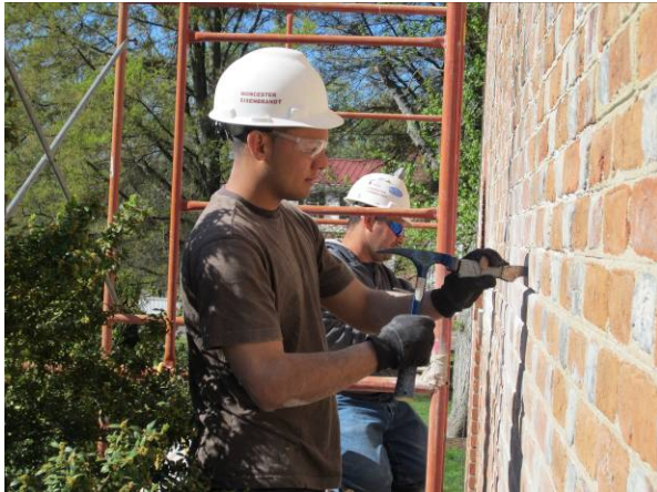
(Left) Removing deteriorated mortar from joints. (Right) Detail after removal and before repointing.
