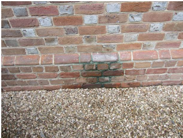
(Left and right) Copper staining on the brickwork due to lightning protection located directly above. This is visible on all four elevations. A copper stain remover might reduce the staining, but should be tested before application.
