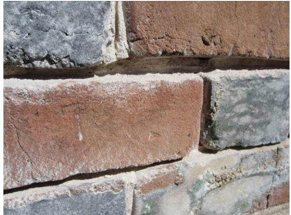
(Left) Removing deteriorated mortar from joints. (Right) Detail after removal and before repointing.
