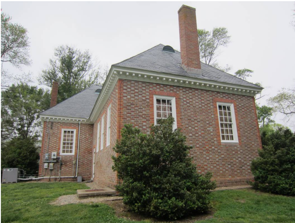
The east elevation after treatment.
