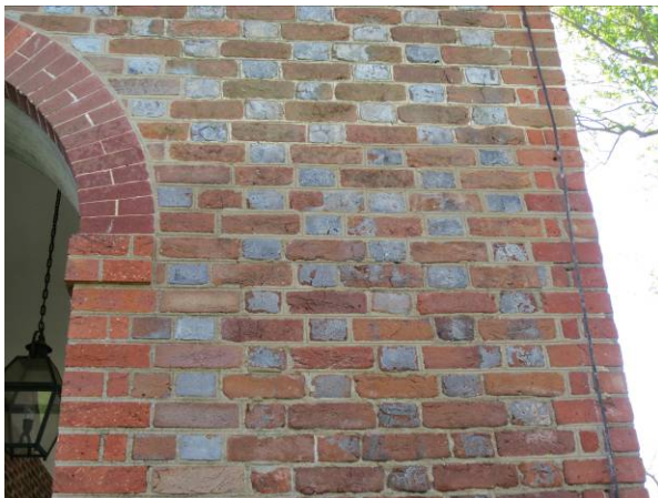
(Left and right) Two views of the wall after repointing.
