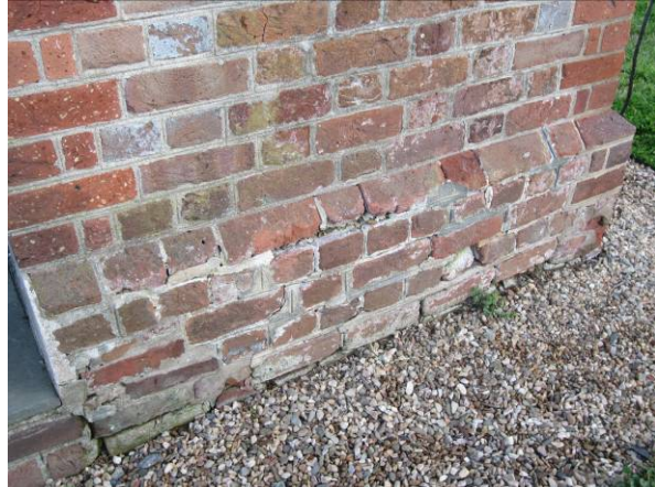
(Left and right) Detailed views of existing conditions of the north elevation, showing biological growth, open joints, and damaged brick. Note the Portland cement repointing at the base.
