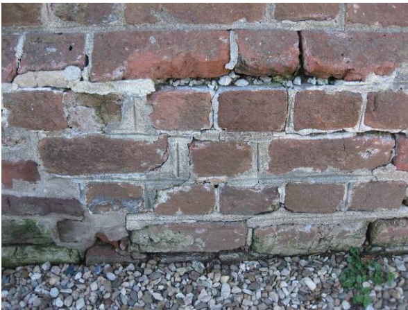
(Left) Existing condition of the base of the building on the north elevation, before restoration work. (Right) Removing deteriorated and damaged brick.
