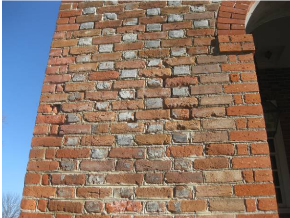
(Left and right) Detailed views of existing conditions of the west elevation before restoration, showing open mortar joints and eroded brick.
