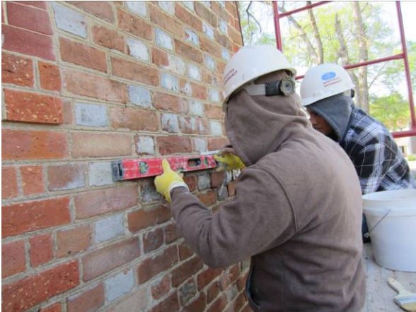
(Left) Using a level to provide a continuous strike across the joints. (Right) The grapevine joint is achieved using a slicker containing a raised bead that is pressed against the mortar, creating an indented u-shaped shadow line in the center of the joint.
