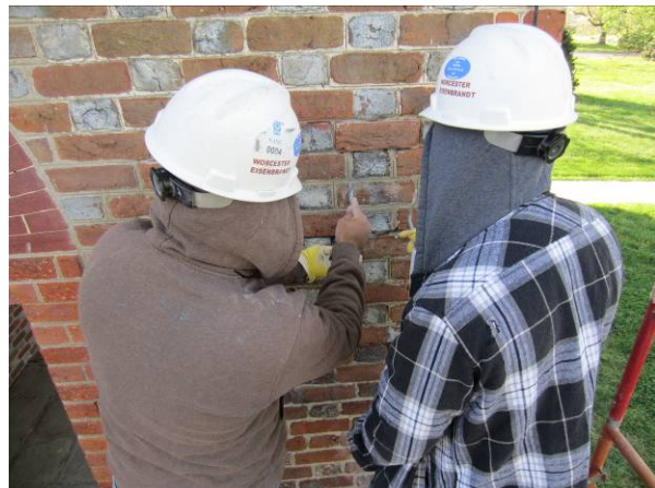
(Left) Wetting down the joints before repointing. (Right) Repointing with a natural hydraulic lime mortar.
