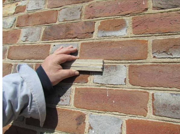
(Left and right) Reviewing samples of brick and mortar for masonry replacement and repointing work.
