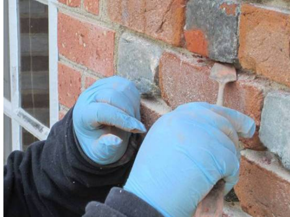
(Left) Two shades of brick patching mortar were used. (Right) Patching the glazed header with Jahn repair mortar.
