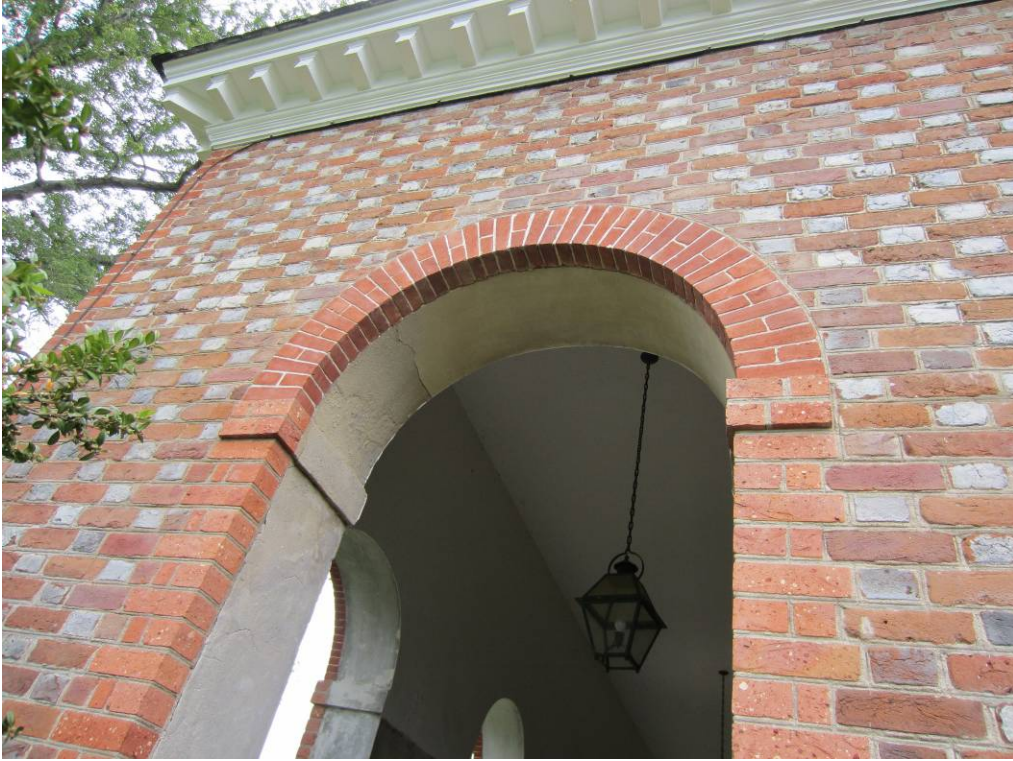
Detail of the piazza arch on the south elevation after treatment.
