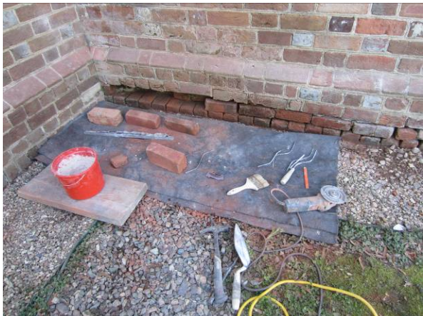
(Left) Installation of original and new brick on the east elevation. (Right) View of work after completion, east elevation.
