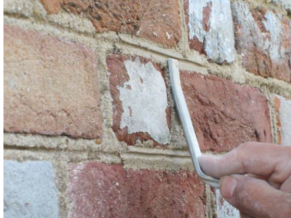
(Left) Using a level to provide a continuous strike across the joints. (Right) The grapevine joint is achieved using a slicker containing a raised bead that is pressed against the mortar, creating an indented u-shaped shadow line in the center of the joint.
