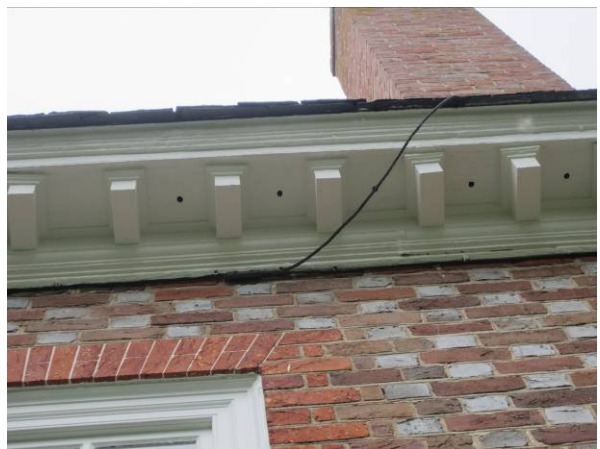
(Left and right) Copper staining on the brickwork due to lightning protection located directly above. This is visible on all four elevations. A copper stain remover might reduce the staining, but should be tested before application.
