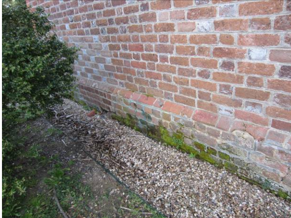
(Left and right) Detailed views of existing conditions of the north elevation, showing biological growth, open joints, and damaged brick. Note the Portland cement repointing at the base.
