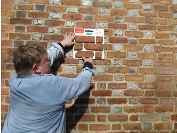
(Left and right) Reviewing samples of brick and mortar for masonry replacement and repointing work.
