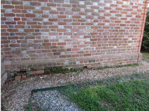
(Left and right) Detailed views of existing conditions of the east elevation before restoration, showing open mortar joints, biological growth, and loose and damaged brick.
