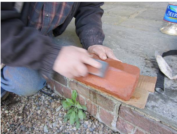
(Left and right) Shaping and preparing new brick, which was sawn with a diamond blade and then hand finished.
