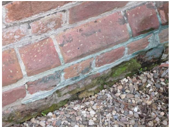
(Left and right) Detailed views of existing conditions of the south elevation before restoration, showing open mortar joints and biological growth. Note the weathered glazing on the headers (left) and biological growth on the masonry (right).
