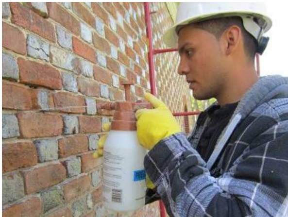
(Left) Wetting down the joints before repointing. (Right) Repointing with a natural hydraulic lime mortar.
