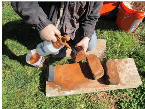
(Left and right) Shaping and preparing new brick, which was sawn with a diamond blade and then hand finished.
