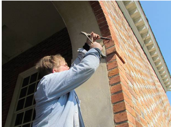
(Left and right) Removing samples of mortar from the wall and arch of the south elevation.
