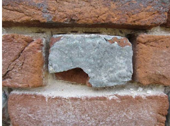
(Left) The new brick inserted in the wall, before setting and repointing. (Right) A damaged glazed header.
