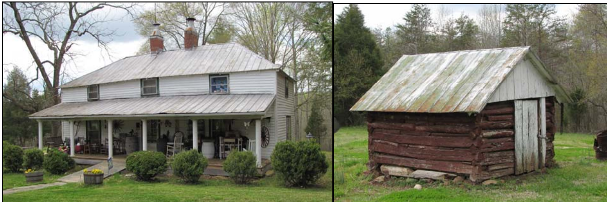
Figure 19: The log house and log smokehouse associated with the 1878 Lawson Farmstead (044-5292) .
