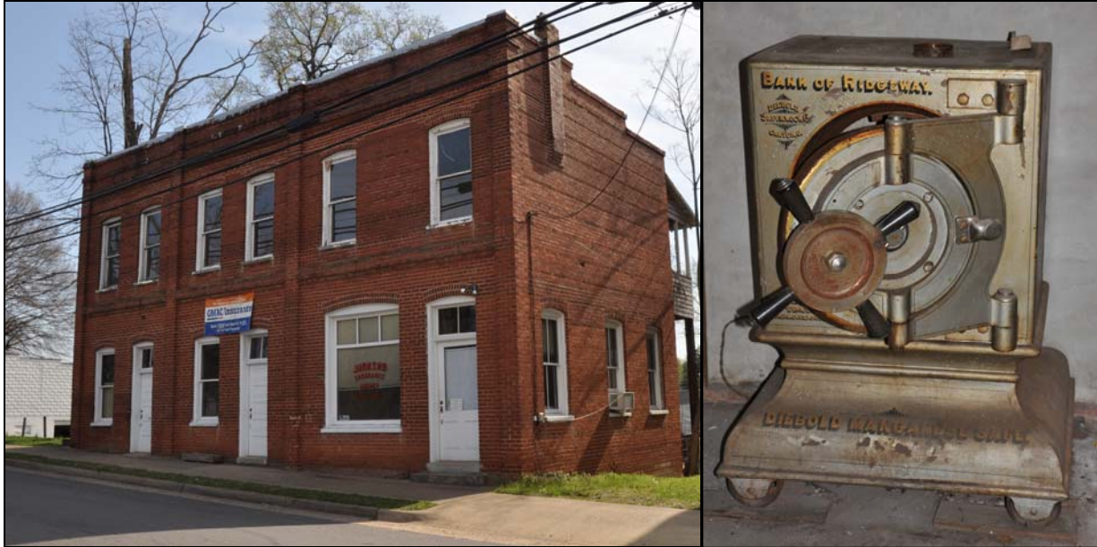
Figure 21: One of only two banks surveyed during the project, the 1909 Bank of Ridgeway (044-5030) and its original safe.
