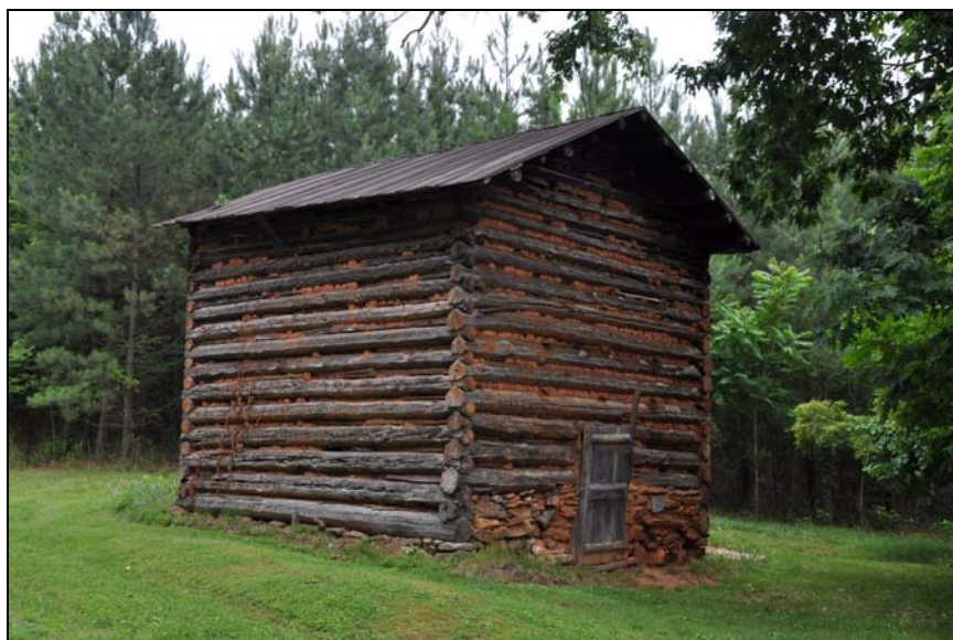
Figure 36: A good example of a 1920s Log Tobacco Barn (044-5358) in the Mayo area of southern Henry County.
