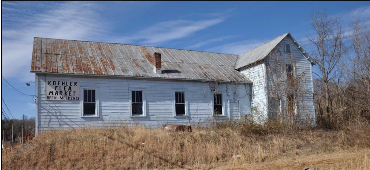
Figure 48: The 1936 frame Koehler Baptist Church (044-5247) retains good integrity but is threatened with neglect and possibly demolition as it sits vacant in the declining community of Koehler. A 1901 Henry County map denoted this area as Wallers Station, which featured a saw mill. By 1920, a board-and-batten Koehler train station was established. Koehler is situated just south of Fieldale, which also had a station; both the Norfolk & Western and the Danville & Western railroads served these communities.
