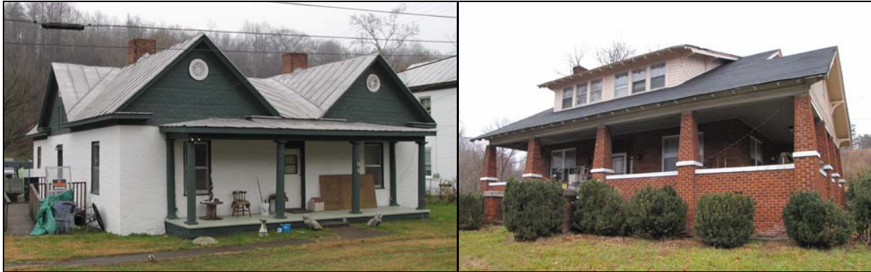
Figures 28 and 29: The Twin Gables House (044-5200) and the Weaver/Rich House (044-5202) are good examples of an atypical Folk Victorian house and an early Craftsman style house both in Bassett.
