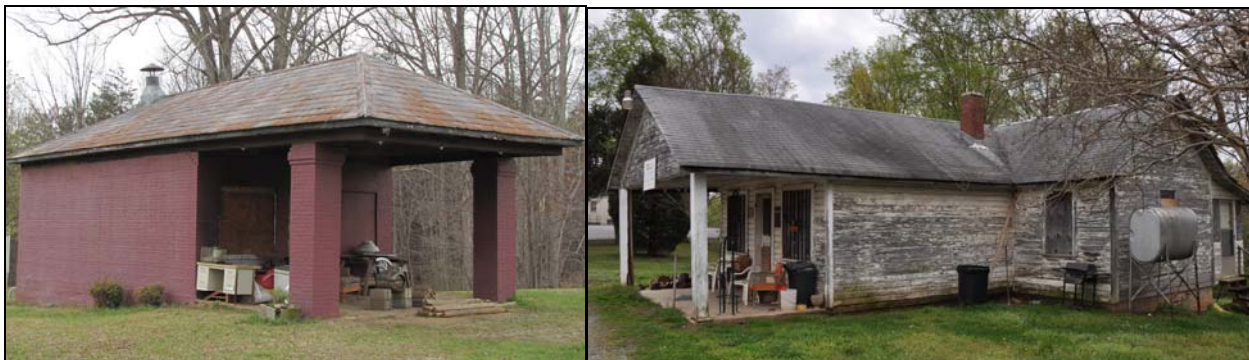
Figures 33 and 34: Two good examples of 1920s porte-cochere style gas stations found in southern Henry County include: the brick Filling Station (044-5285) with a pressed metal shingle roof and a pressed metal tin ceiling, sitting vacant just north of the North Carolina border off S.R. 87; and the frame Odell's Trading Post/Filling Station (044-5291) with an attached residence on Old Leeksville Road between Ridgeway and North Carolina.
