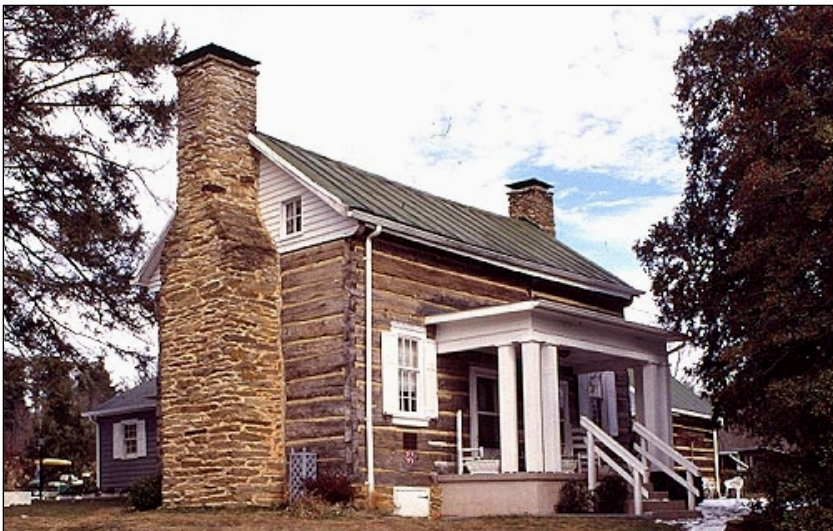
Figure 8: The massive stone and log construction of the Old Turner Place (NRHP 044-0105) .
