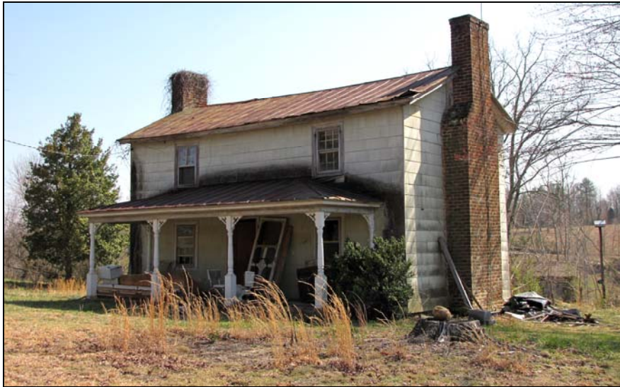
Figure 13: The ca. 1850 Lester House (044-5267) in the Figsboro community features a three-bay center-passage, single-pile plan on a fieldstone foundation. Exterior-end brick chimneys heated the residence.
