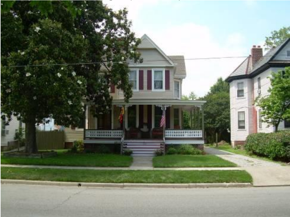
Figure 3.7: 323 E. Pembroke Street Hampton (114-0118-0021)
