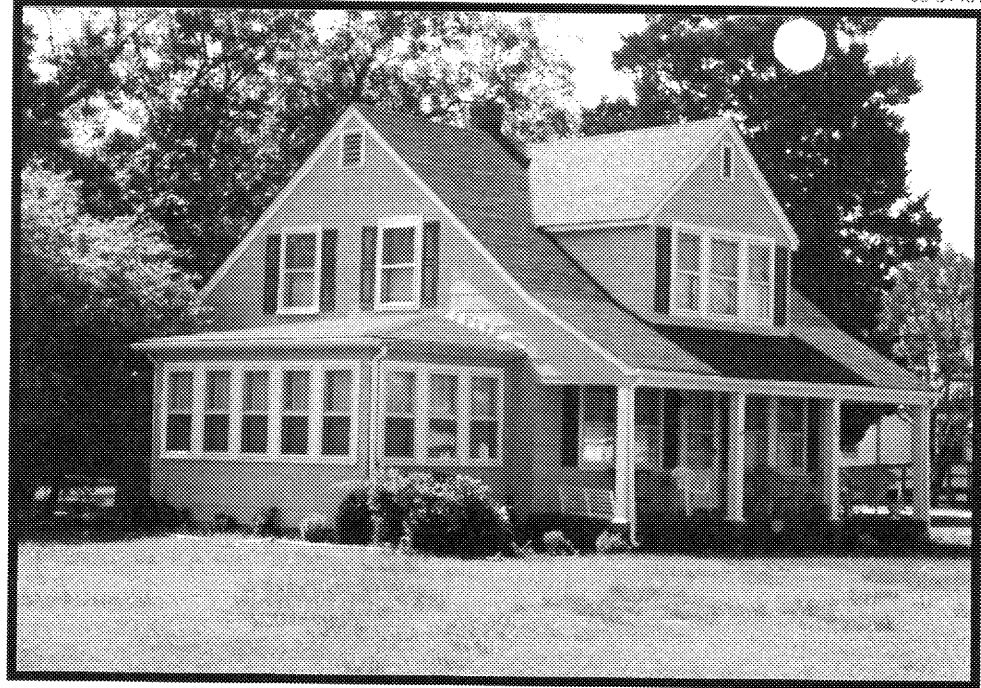
Plate 2. House (300-5013) typical of houses built in the first half of the twentieth century in Smithfield.
